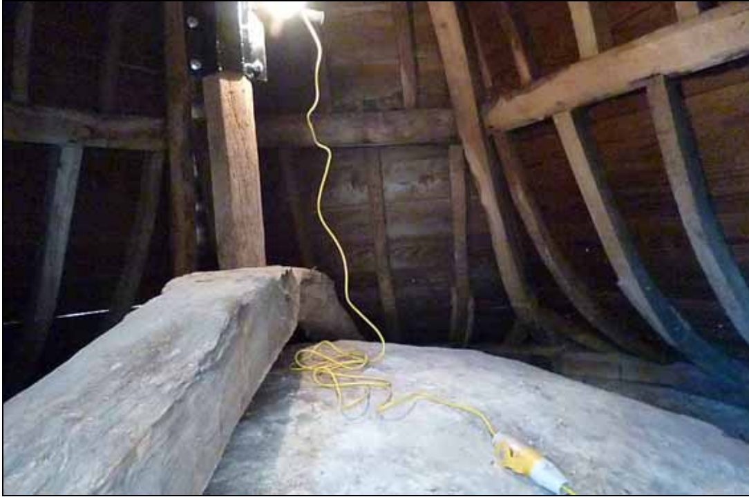
Figure 4: Muniment Room roof (photograph Robert Howard)
