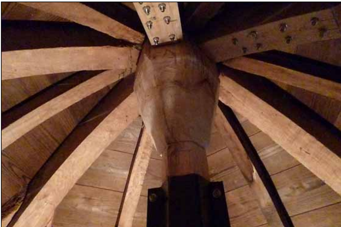
Figure 5: Muniment Room roof (photograph Robert Howard)
