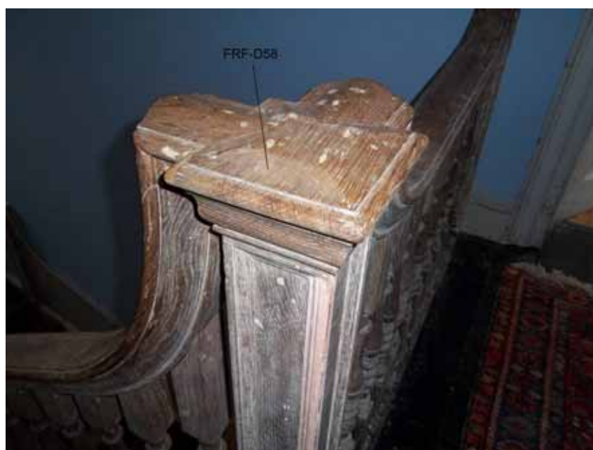
Figure 28: Photograph of first-floor newel post cap, showing the location of sample FRF-D58 in the Connecting range (RobertHoward)
