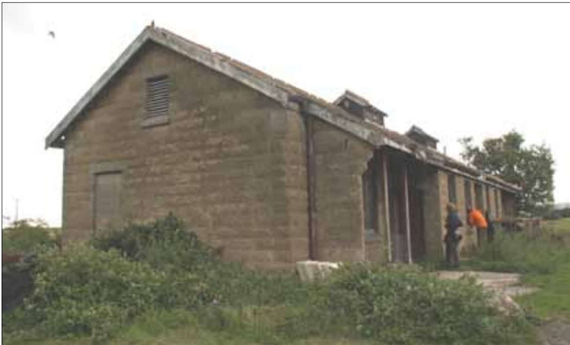
Figure 30. Powerhouse from the north-west.
