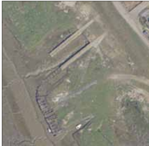
Figure 9. Further detail showing wharf and dock.
