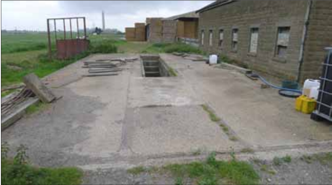
Figure 38. Concrete base with inspection pit, formerly a railway engine shed, from the north-west.
