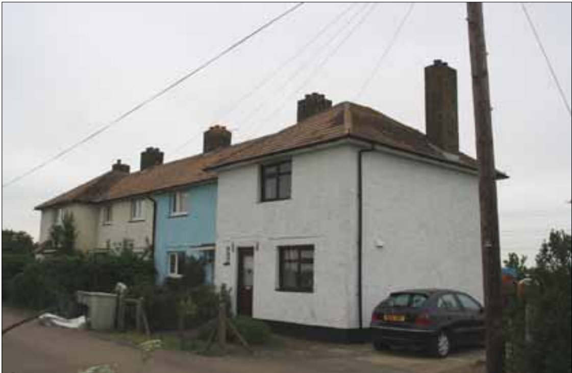
Figure 22. Frontage of police cottages, viewed from the northwest.
