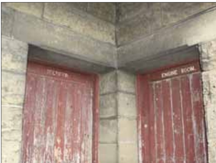
Figure 32. Detail of powerhouse doors, showing high quality of masonry and good condition of paintwork on panelled wooden doors.
