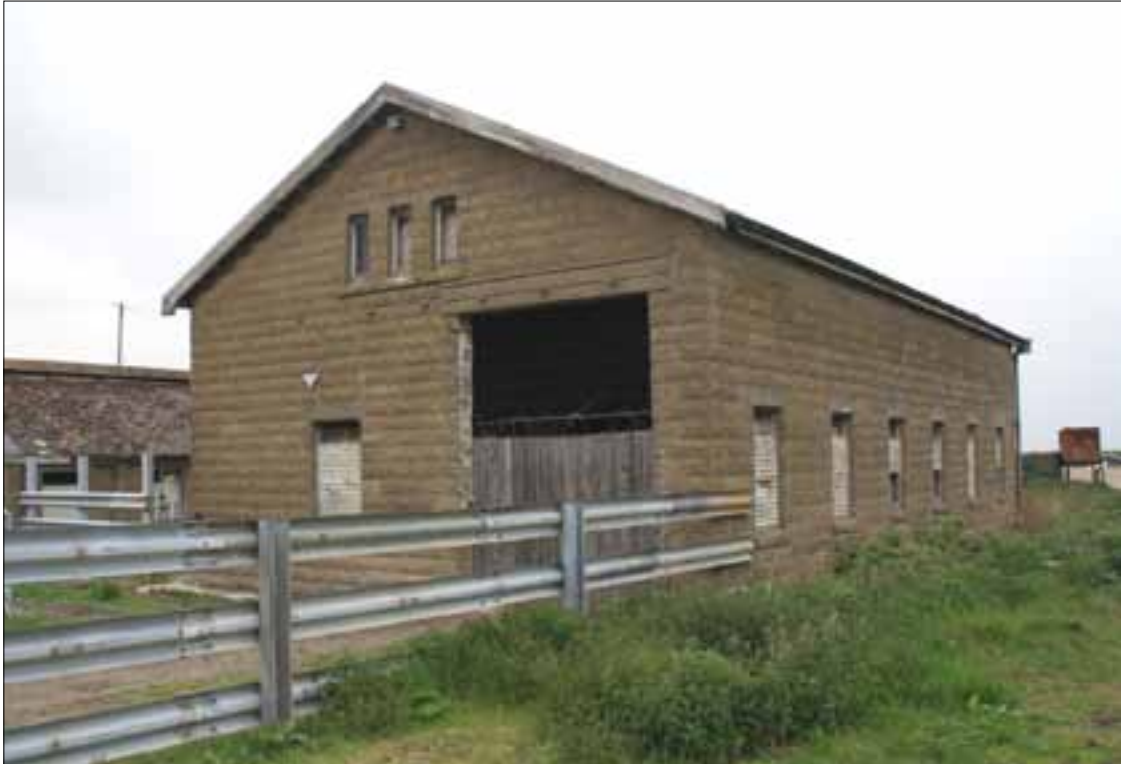
Figure 35. Main workshop building from the east.
