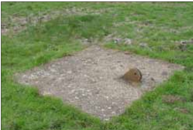
Figure 50. Anchor point for velocity screen mast cable. The embedded metal fixing for cable attachment points towards the position of the former velocity screen mast.
