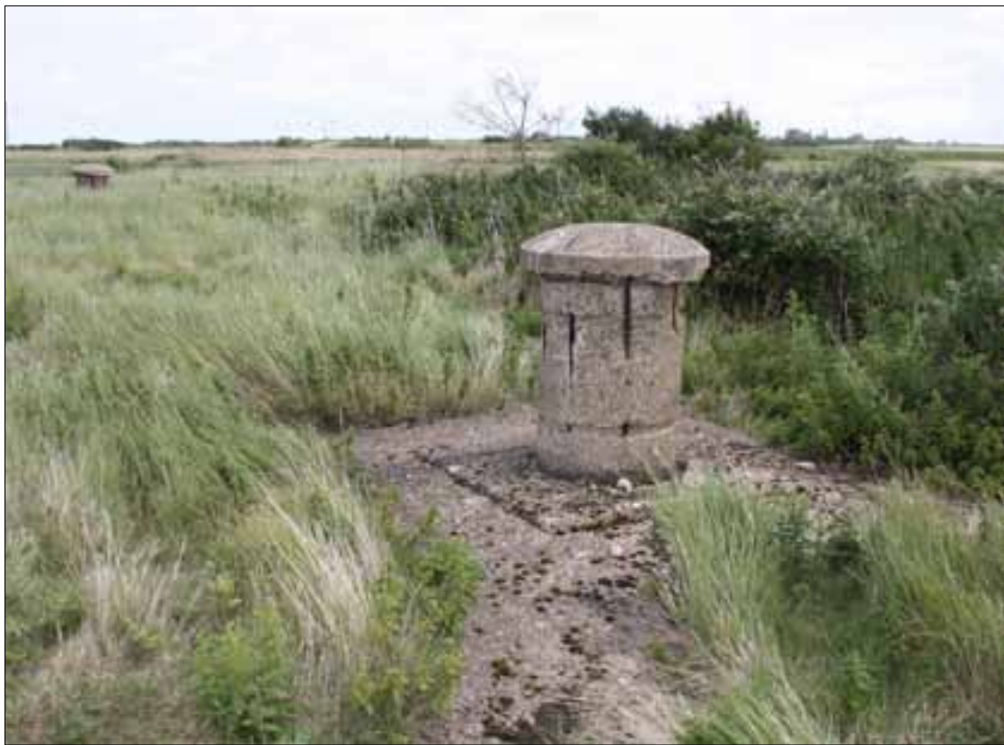
Figure 56. Bollards for tethering, looking east.
