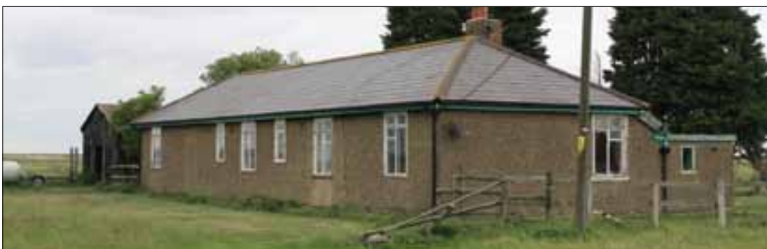
Figure 27. Former barracks and NCO rooms, from the southwest.
