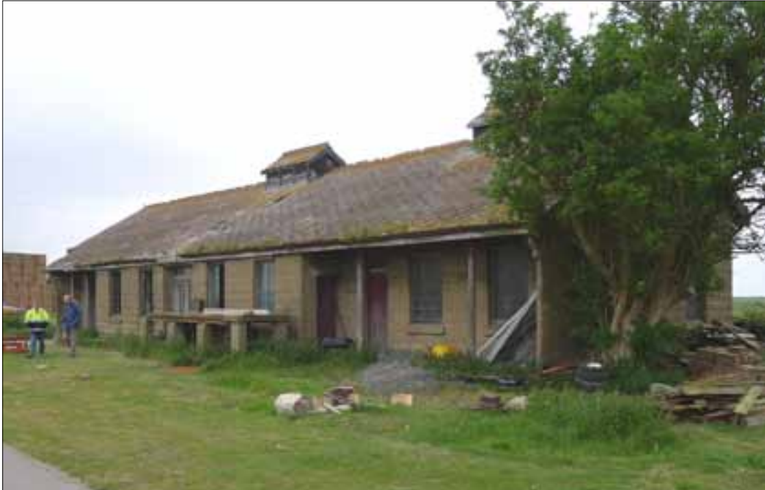
Figure 29. Powerhouse from the south.
