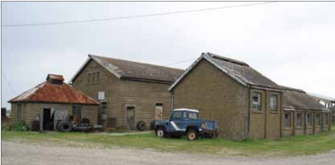
Figure 33. Workshop complex from the west.
