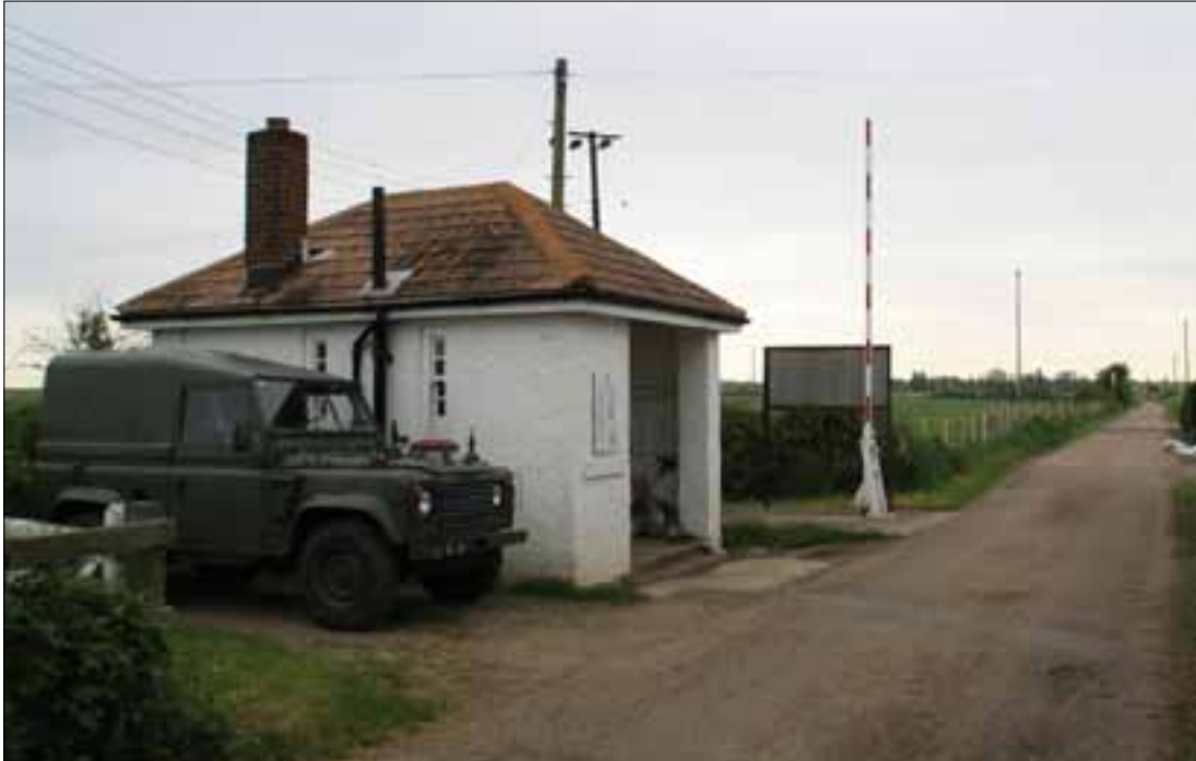
Figure 26. Guardhouse and barrier from the west.
