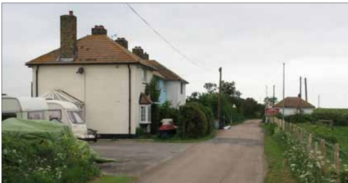
Figure 21. Row of police cottages and guardhouse from the east, as seen from the road approaches.
