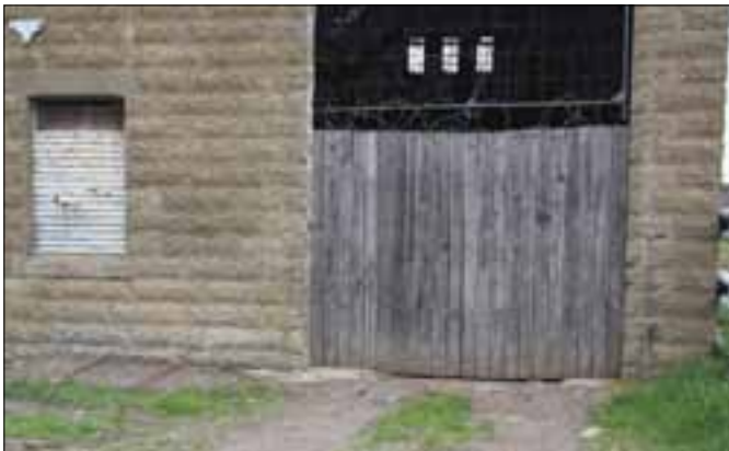
Figure 36. Detail of main workshop entrance, from the south-east. Standard gauge rails are visible on the ground heading into the workshop. Also visible are narrow gauge rails apparently heading under the walls to the left of the entrance.
