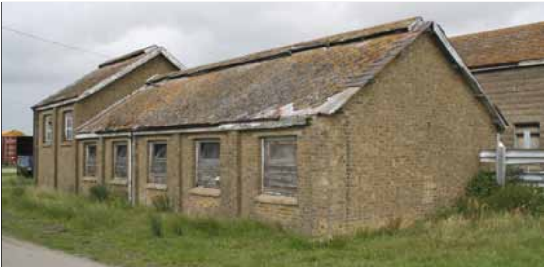
Figure 39. Later building to south-west of main workshop, from the south.
