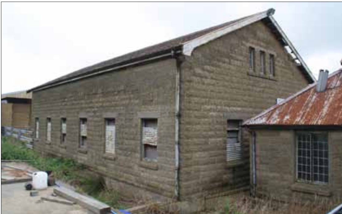
Figure 34. Main workshop building from the north.
