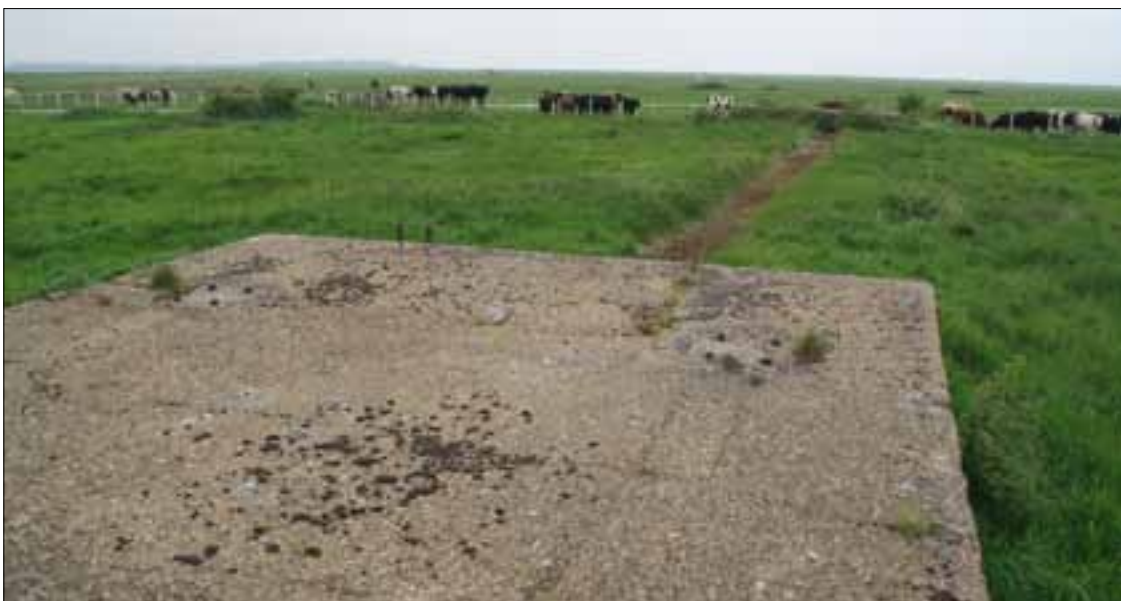
Figure 48. Looking northwest along arm of outer and longer velocity screen mast base.
