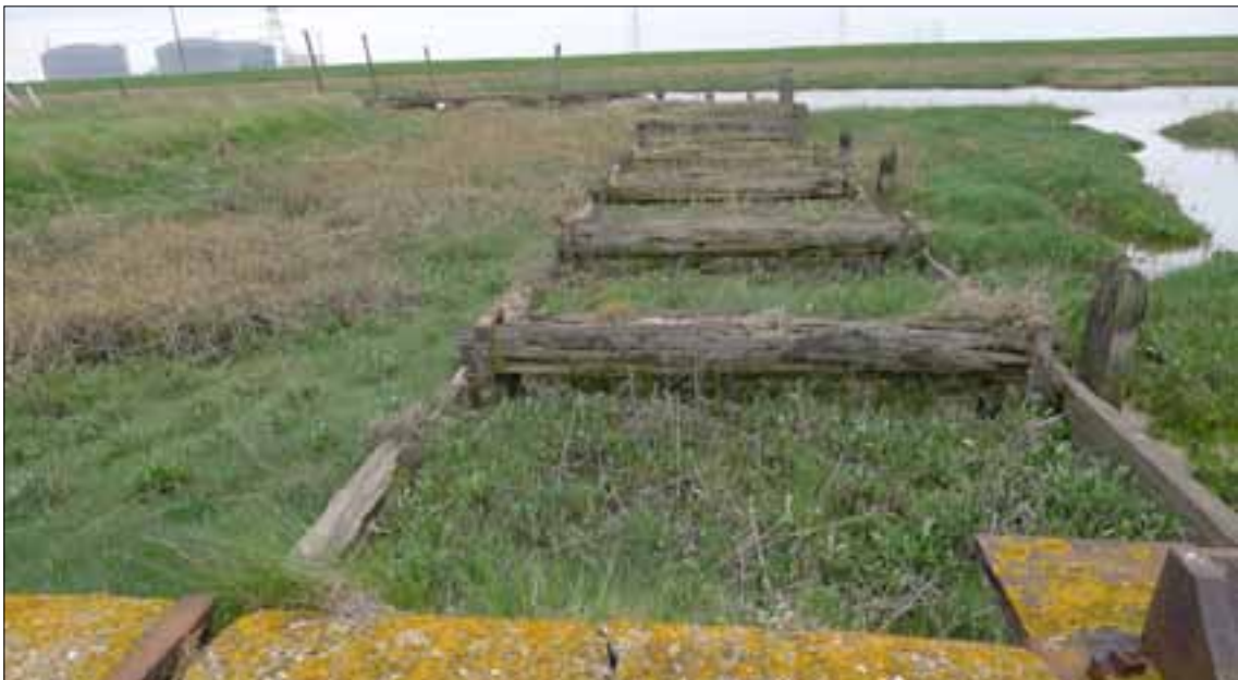
Figure 45. Timber wharf base, looking south-west from end of dock.
