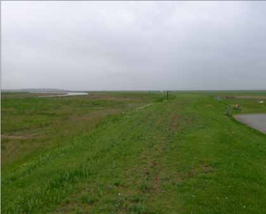
Figure 58. Floodbank, looking northwest, from top of bank level with gantry path.
