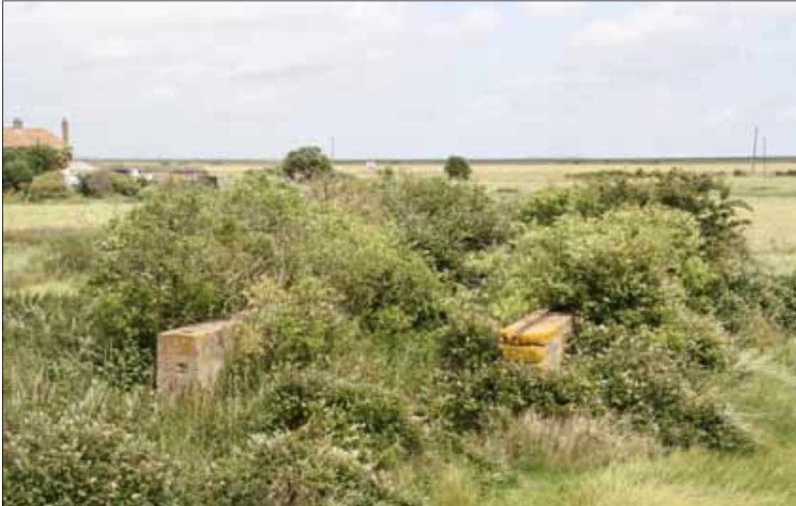
Figure 55. Overgrown remains of railway firing point structures, looking east.
