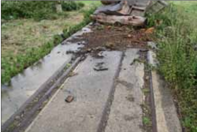
Figure 42. Detail of rails on one of the linear concrete bases of the gantry path.
