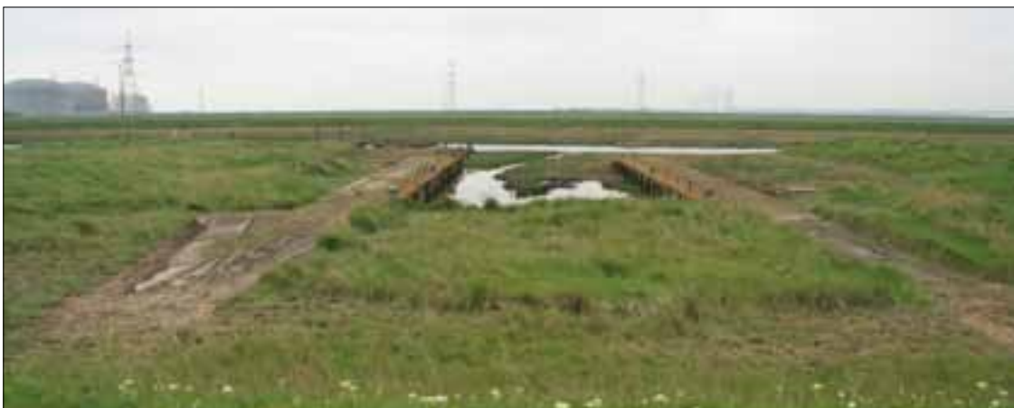
Figure 43. Dock, from bank, looking south-west.
