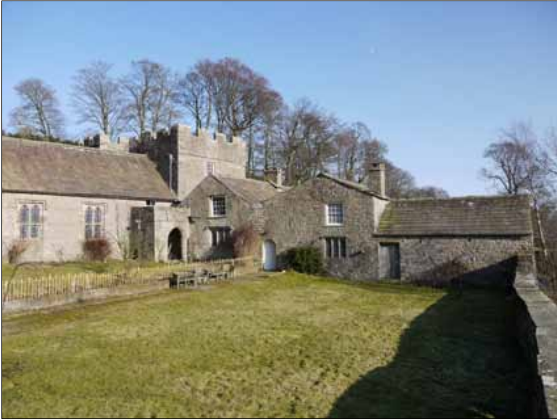
Figure 9. The service range viewed from within the courtyard (photograph Adam Menuge, English Heritage).
