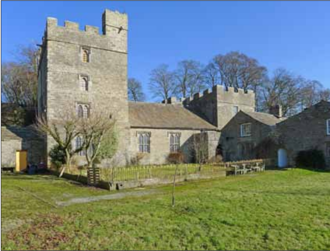
Figure 4. The hall range viewed from the south (photograph: Lucy Jessop, English Heritage)
