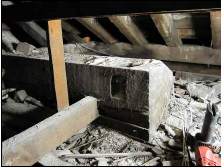
Figure 6: The T21 tiebeam end with a rafting or hauling hole. Photo Ian Tyers
