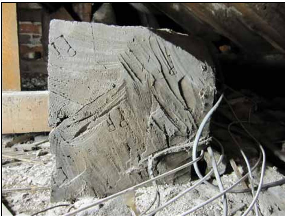
Figure 7: The T21 tiebeam end with multiple PR stamps. Photo Ian Tyers
