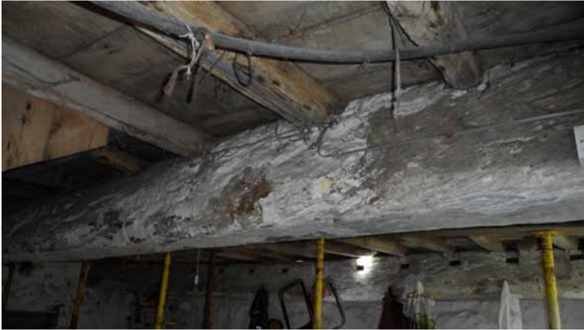
Figure 15: Service range, Tack room, ground-floor ceiling, photograph taken from the north-west (Alison Arnold)
