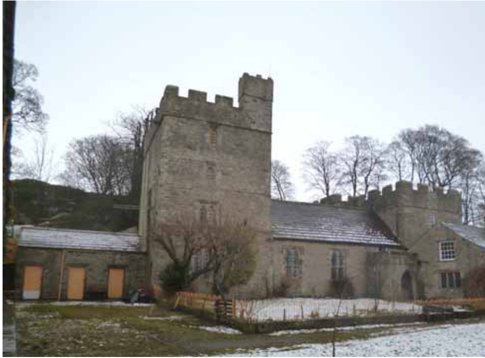
Figure 5: North range, with Woodshed to left and Low-end tower to right (Alison Arnold)
