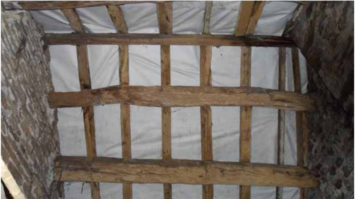
Figure 11: Woodshed, roof, bay 2, photograph taken from the south-west (Alison Arnold)
