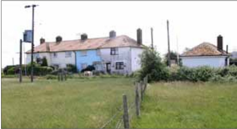
Figure 19 The police cottages on Peat Way (P57330005)
