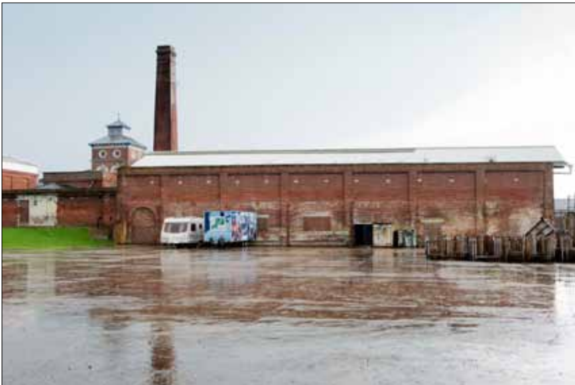
Figure 28. Gunboat sheds from the east (EHA DPI61542)
