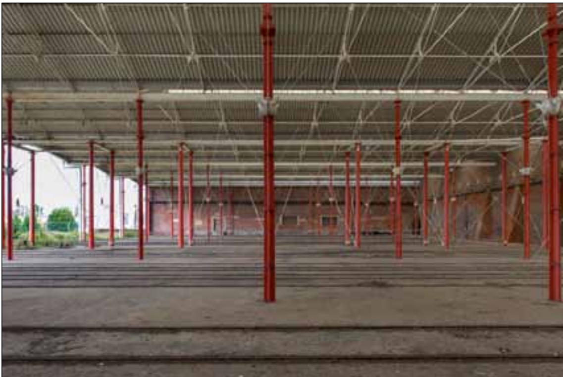
Figure 31. Gunboat sheds interior from south west (EHA DPI61548)
