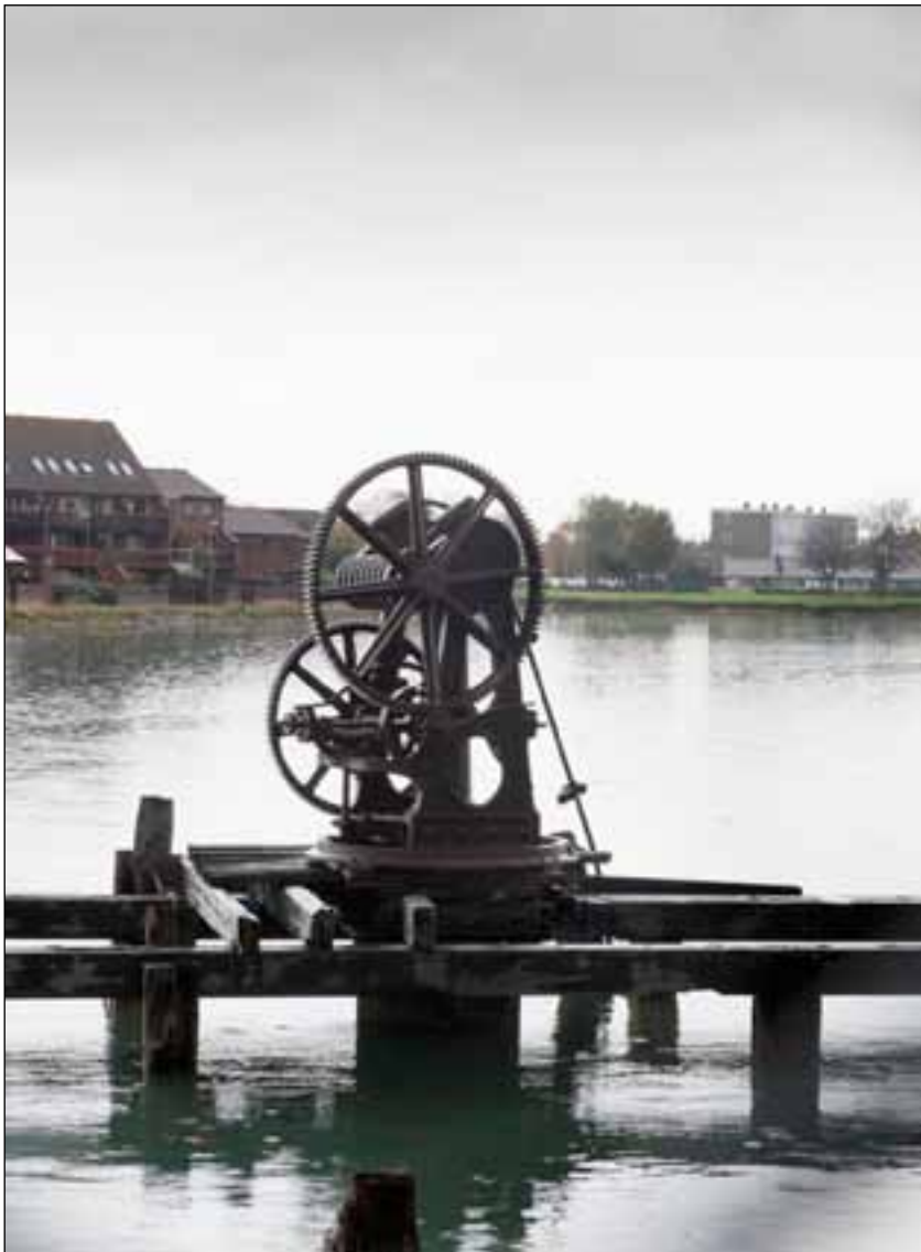
Section of timber jetty with crane (EHA DPI61577)
