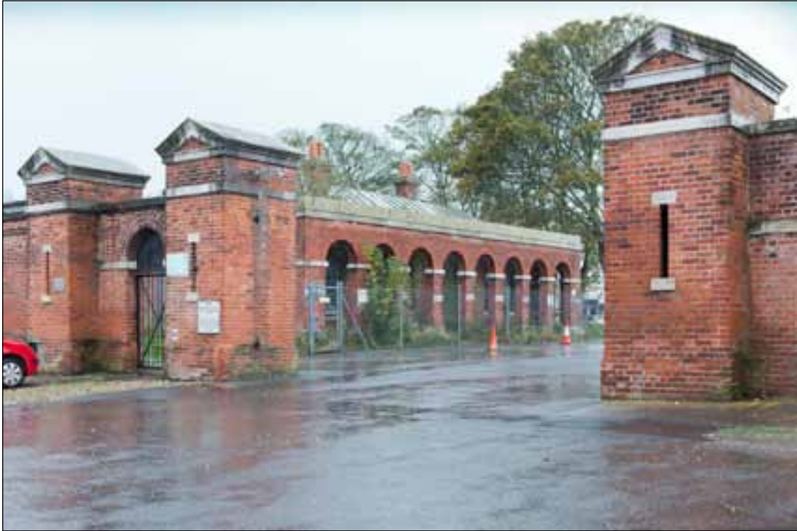
Figure 55. Main entrance to the Gunboat Yard (EHA DPI61568)
