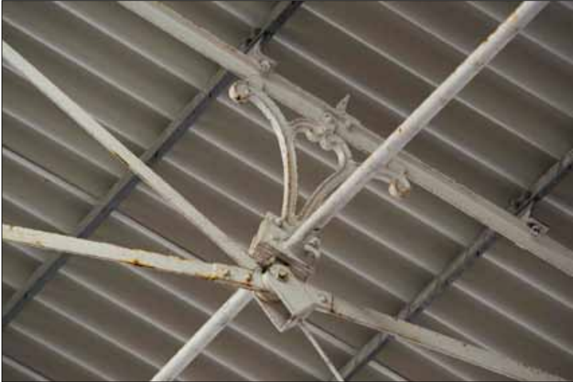
Figure 39. Decorative spandrel detail (EHA DPI61556)
