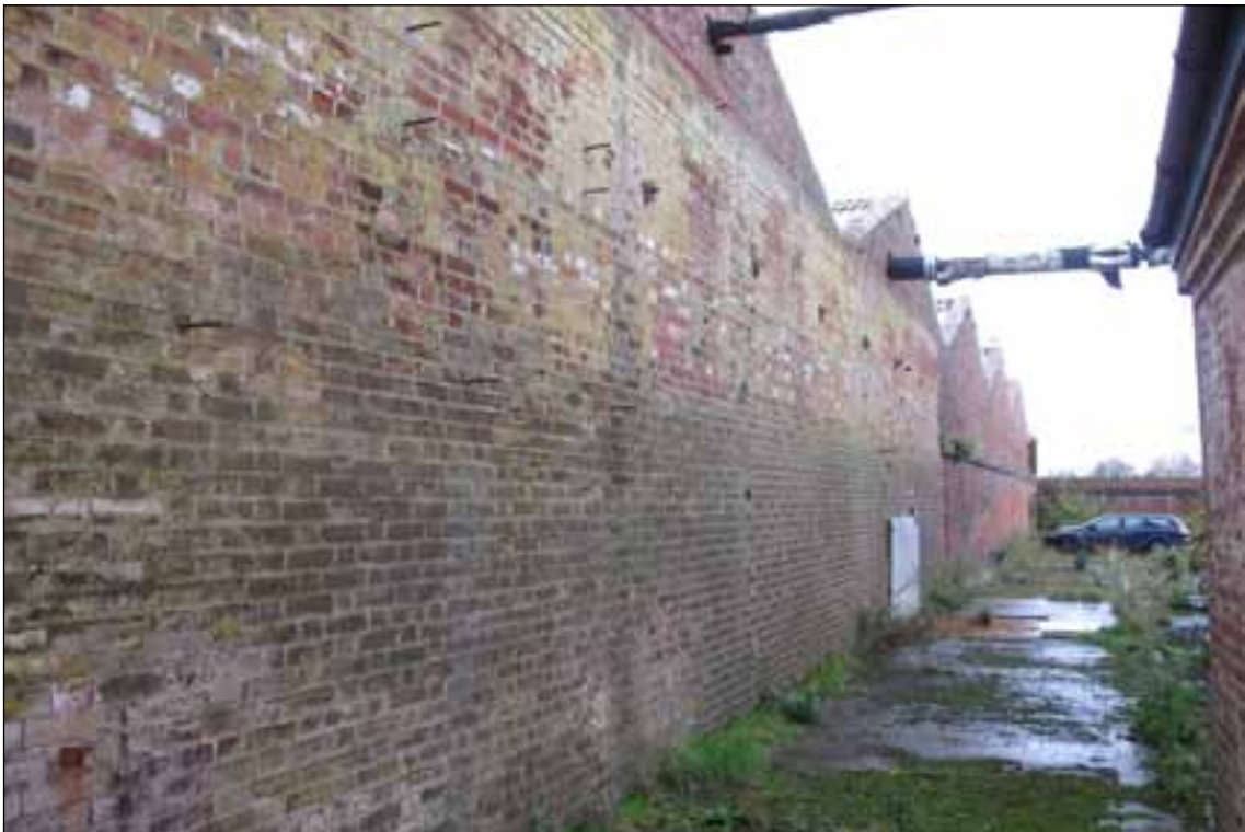
Figure 29. Brick gable on south wall of sheds (© English Heritage)
