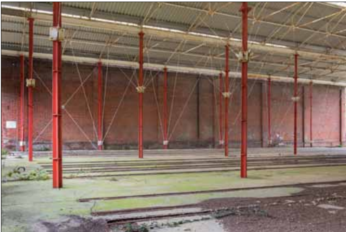
Figure 40. Rails visible in shed interior (EHA DPI61551)
