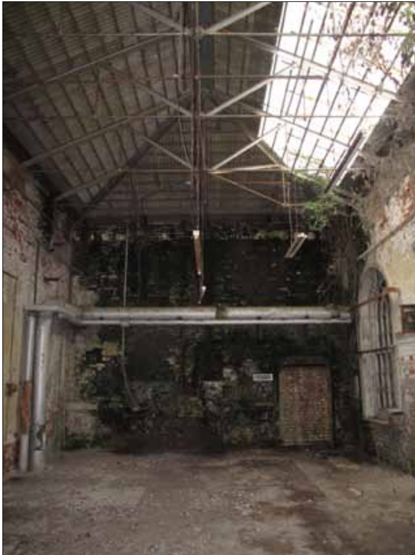
Figure 47. Interior of the engine house looking west, showing the blocked doorway to the boiler house (© English Heritage)
