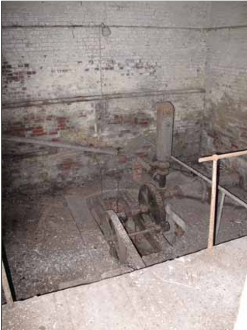
Figure 48. Interior of well house to the east of the engine house showing winch mechanism (© English Heritage)
