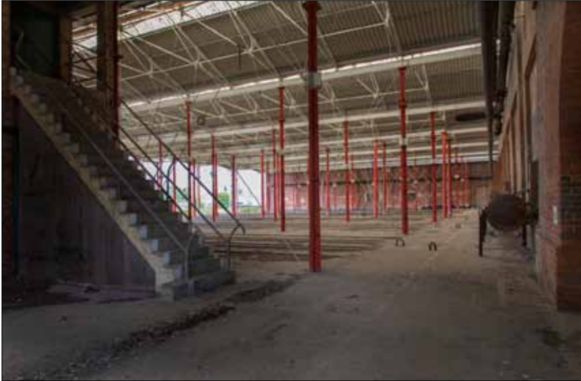
Figure 33. Interior of gunboat sheds from south, showing the stair to the upper storey of the inserted brick building (EHA DPI61552)
