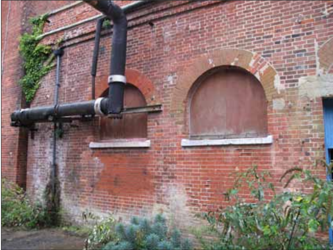
Figure 44. North elevation of the boiler house, showing the two window openings
