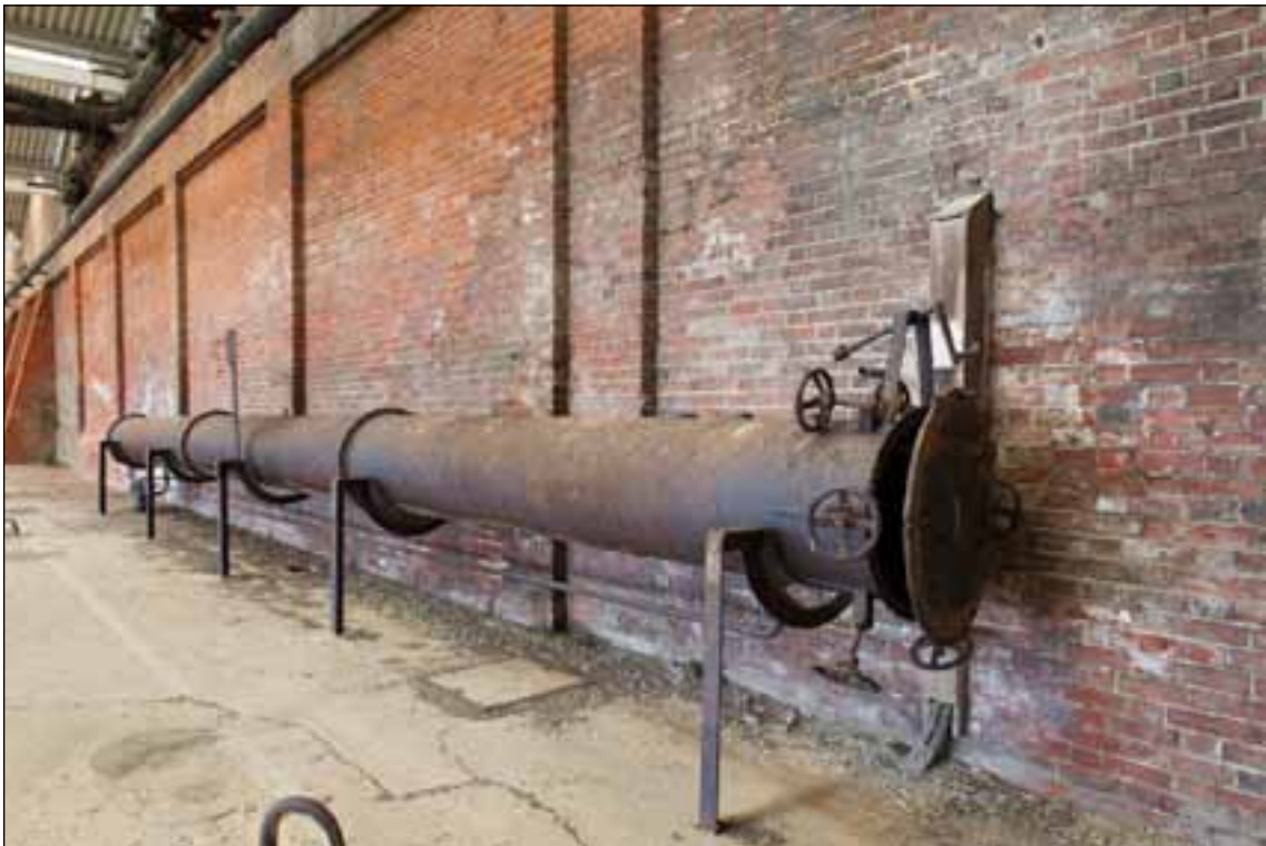
Figure 32. Steam pipe for softening wood (EHA DPI61555)
