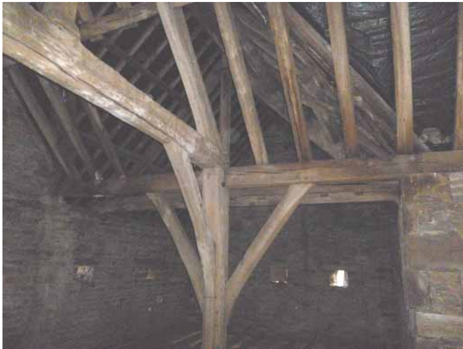
Figure 3a/b: Views of the barn looking east to west (top) and from truss 1 into present short south wing (bottom) (Robert Howard)
