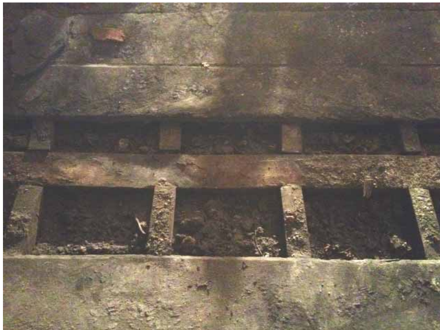
Figure 8: Attic-floor frame, viewed from above (Alison Arnold)
