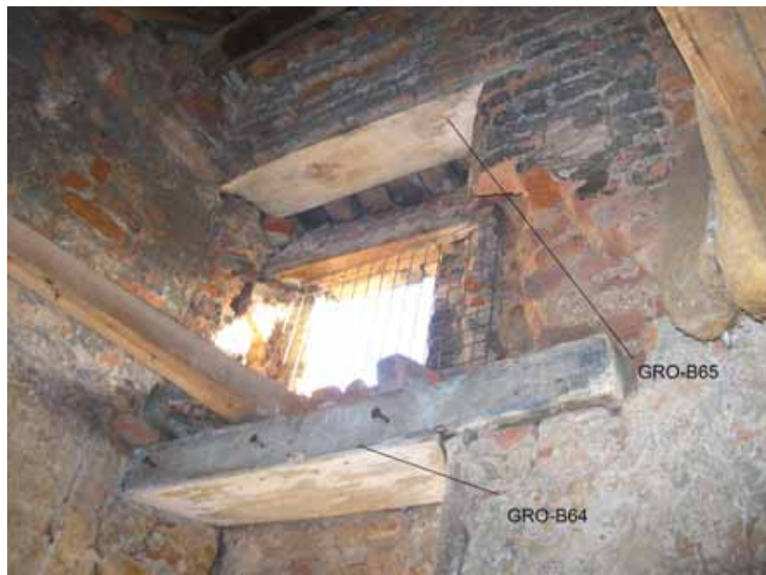
Figure 16: Tower 2 window lintels (GRO-B64 and GRO-B65), photographs taken from the north-west (Alison Arnold)
