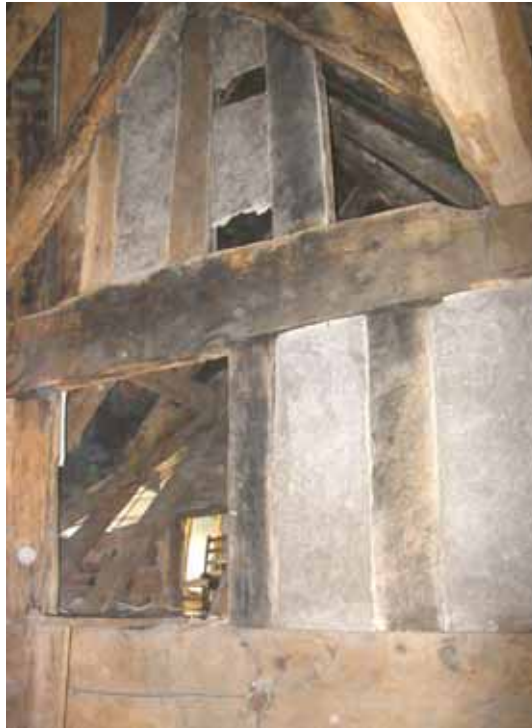
Figure 5: Smoke-blackened truss in the former open hall, photograph taken from the north (Robert Howard)
