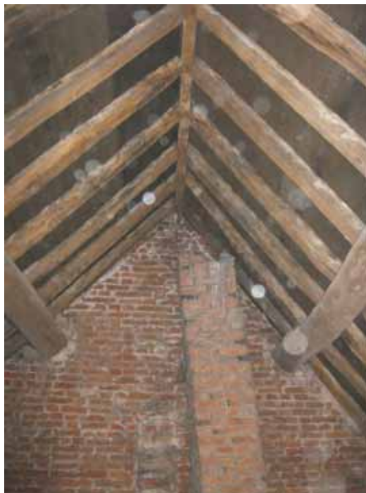
Figure 5: Smoke-blackened truss in the former open hall, photograph taken from the north (Robert Howard)
