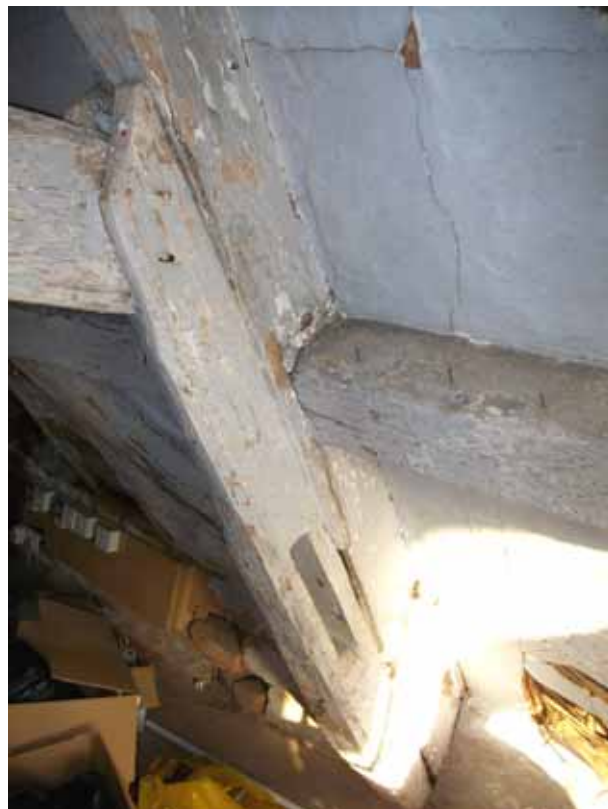
Figure 8: Repair to the principal rafter, truss 1 in the cross-wing, photograph taken from the south (Alison Arnold)
