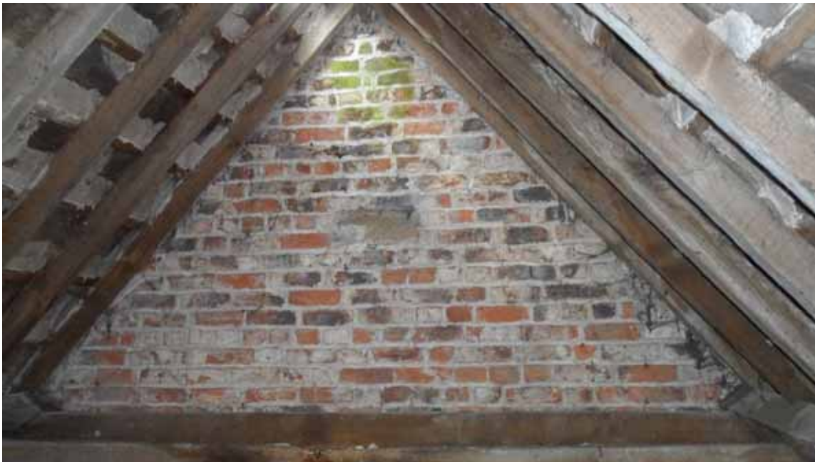
Figure 14: The mash house roof, photograph taken from the north (Alison Arnold)
