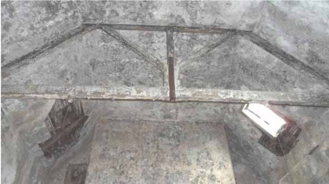
Figure 11: Sockburn Hall, north rear-range roof, photograph taken from the north-west (Alison Arnold)
