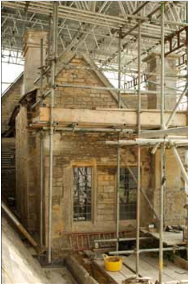
Fig 4. The 15th-century chimney stack on north side of former south lodging tower, seen on the side elevation, to the left. (DPI52835)
