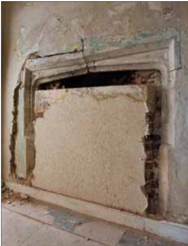
Fig 5. Fireplace in north wall of S3.03, attic of south range. (DPI61398)
