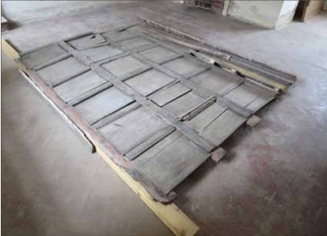
Fig 15. Panelling from the south wall, with added pine rails to rear. (N. Hill)
