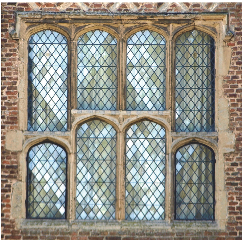
Figure 4. Oxburgh Hall, King's Room, north-facing window (exterior)
