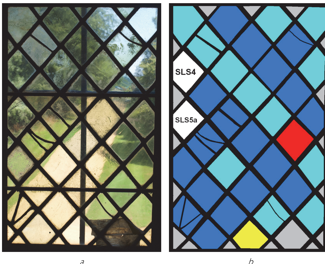
Figure 7. The lower portion of window K3 in the King's Room Turret a = photograph b = diagram of the same window (dark blue = HLLA1; light blue = HLLA2; red = kelp; yellow = façon de venise; white = SLS; grey = not analysed)
