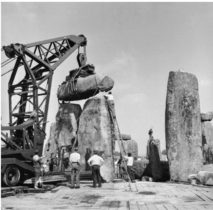
Figure 8: Re-erection of the Trilithon lintel by the 60 ton crane, the larger of two cranes used to lift the stones. The lintel is being lowered and moved into its final resting position on upright stones 57 and 58. January 1958. Reproduced by permission of English Heritage. Reference Number: P50217
