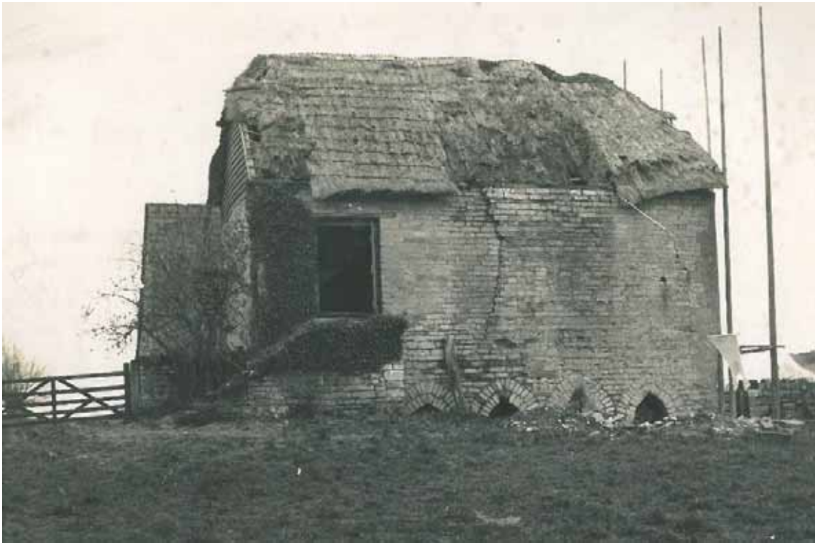
Figures 21 and 22: Muchelney Abbey reredorter in 1931 prior to repair (Copyright The National Archives. File: WORK 14/741) and today (Copyright A Riley).
