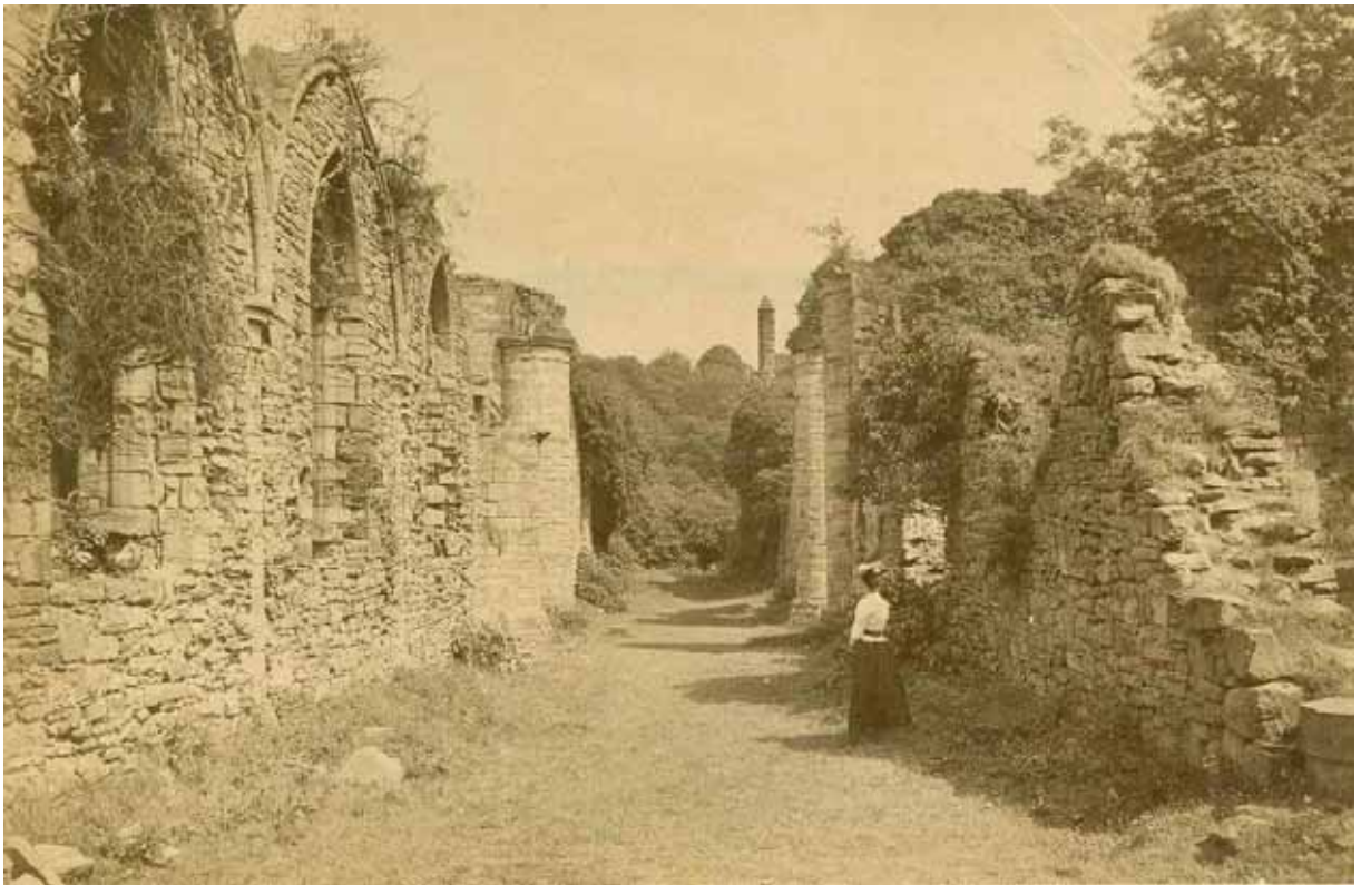
Figures 30 and 31: Top: Finchale Priory in 1906. Copyright The National Archives. (File: WORK 14/34). Bottom: The same view today. © English Heritage Photo Library.
