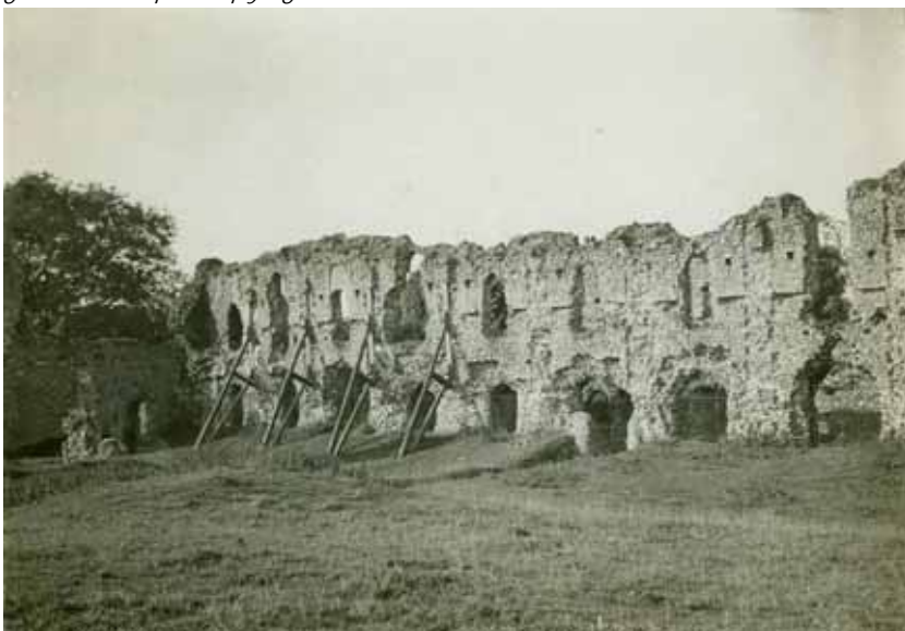
Figure 10: The shored up east wall of the dorter at Castle Acre Priory prior to guardianship. Copyright The National Archives.
