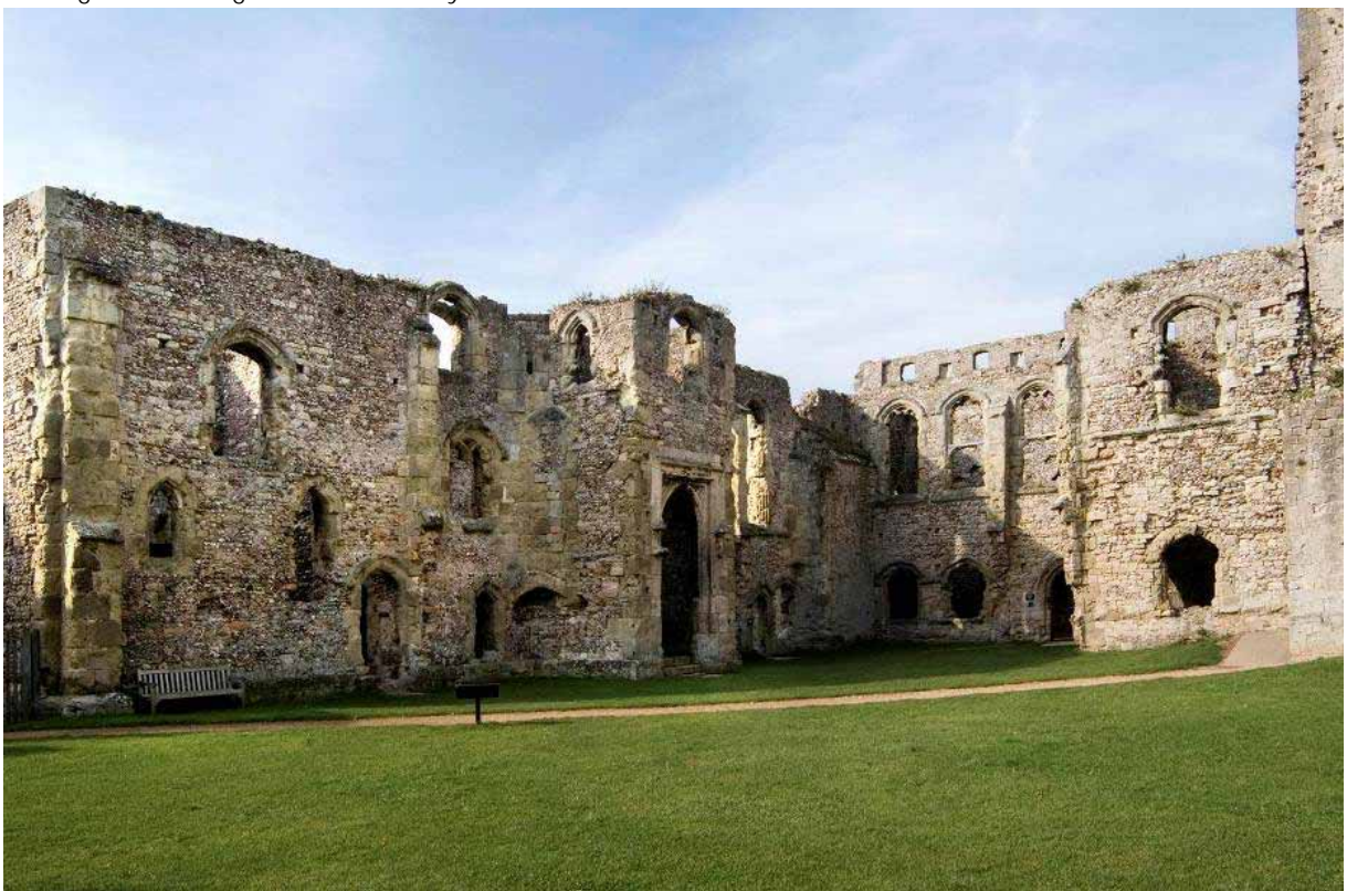
Figure 35: The Great Hall, Solar and Chapel, Portchester today. © English Heritage Photo Library.
