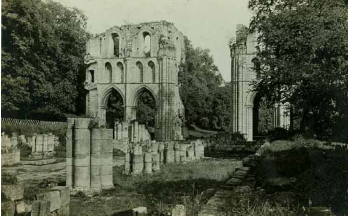
Figure 15: Roche Abbey nave circa 1920. Copyright The National Archives. (File: WORK 14/455).
