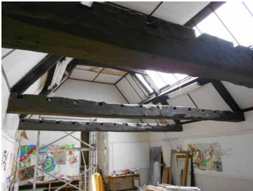
Figure 3: View of the three original tiebeams at first-floor level, looking west. (Photograph Martin Bridge)
