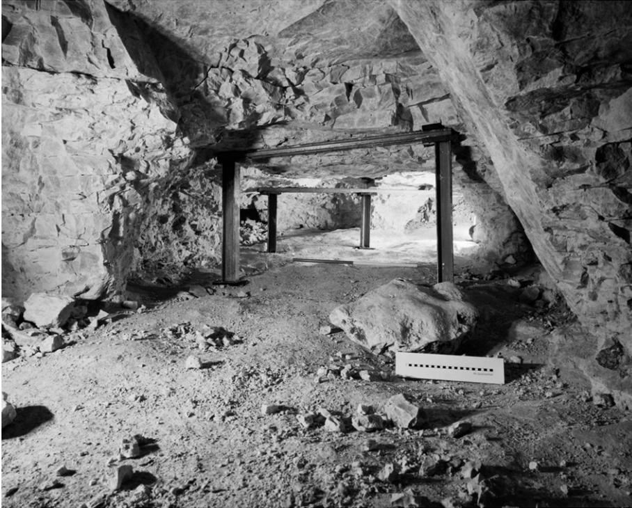
*Figure 22: Greenwell's pit gallery III2B. The pit props were inserted following investigations by the Prehistoric Flintmines Working Group of the Dutch Geological Society, Limburg Section © English Heritage*
