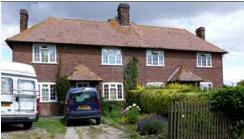
Figure 11 A block of four cottage flats forming part of the SRDC's Pips View development of 1948-53. (P5733052)
