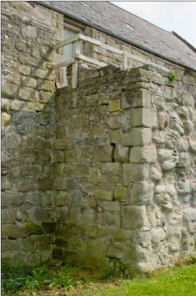
Figure 12: Turret on the south-west elevation of the vaulted building (DPI56908 © English Heritage, photograph: Alun Bull).
