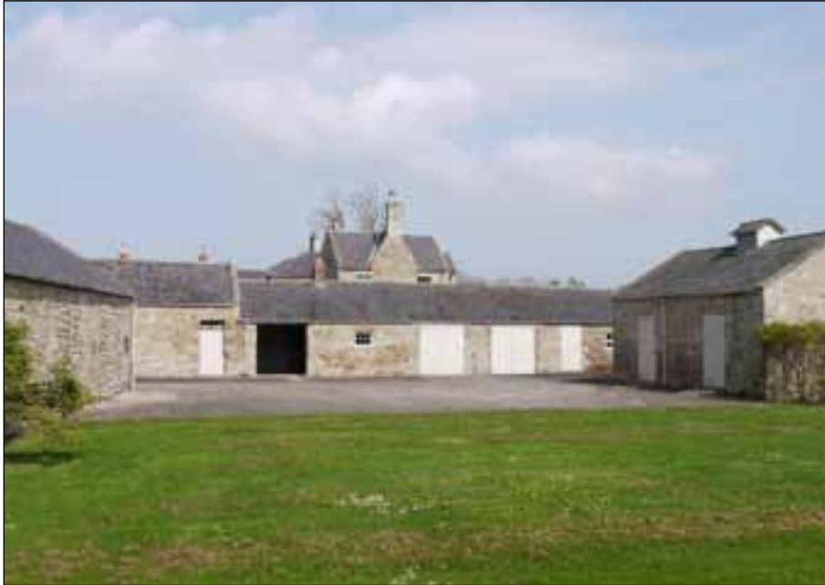
Figure 37: The outbuildings to the south-west of the farmhouse (© English Heritage, photograph: Clare Howard).
