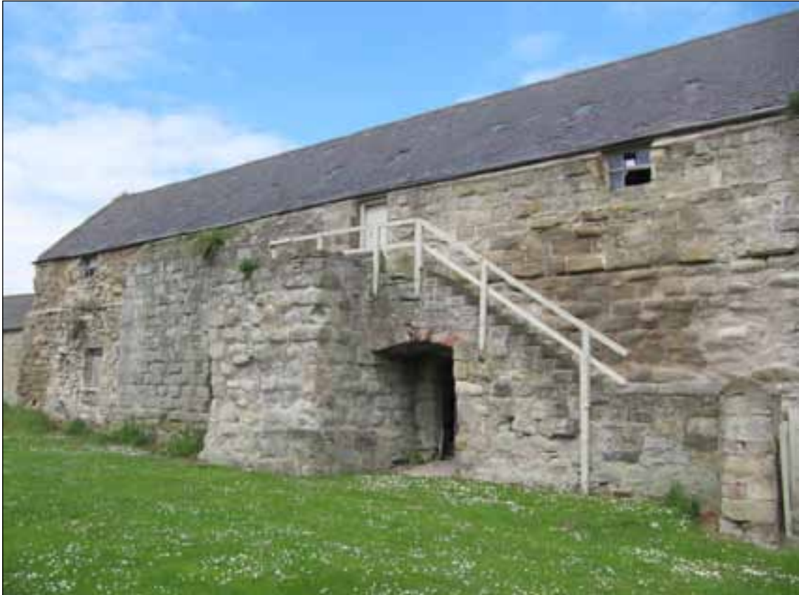
Figure 11: The south-west elevation of the vaulted building (© English Heritage, photograph: Clare Howard).
