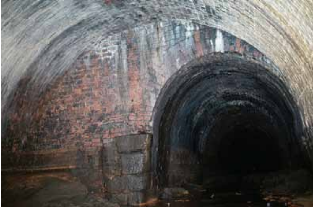
Figure 10: East facing internal elevation of the wide hole, showing stone quoins protecting the projecting west corner, looking west (after Witter 1979, image 11), © Robin Witter, reproduced with permissions
