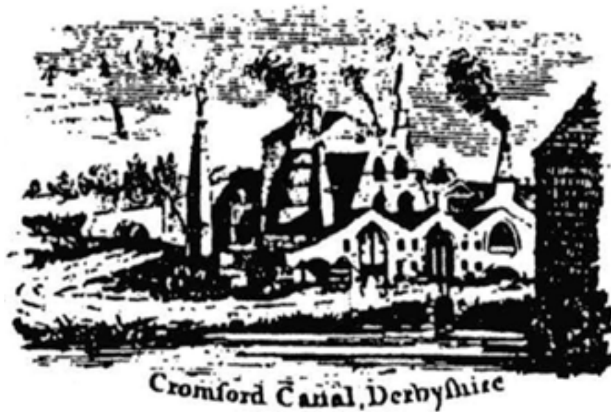
Figure 18: Detail from an 1801 Bill of Exchange showing the Butterley ironworks (after Riden 1990, 50 figure 2), reproduced with permissions
