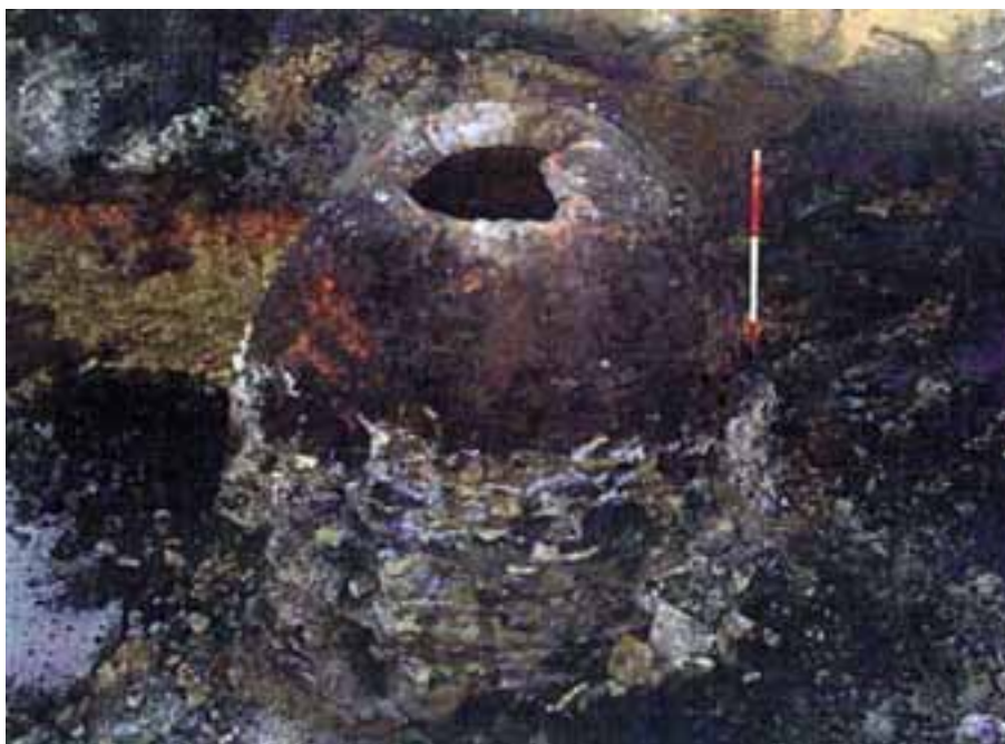
Figure 17: Domed brick capping on a shaft exposed during archaeological watching brief (after Farnworth-Jones and Boucher 2007, 7, figure 4), © ULAS, reproduced with permissions
