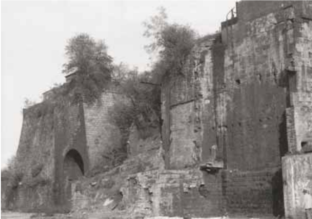
Figure 4: Remains of the two blast-furnaces incorporated within the retaining wall at the Butterley Ironworks ('Structure 1'), looking north-east (after Palmer and Neaverson 1992, 103, figure 115). Reproduced by kind permission, © Marilyn Palmer
