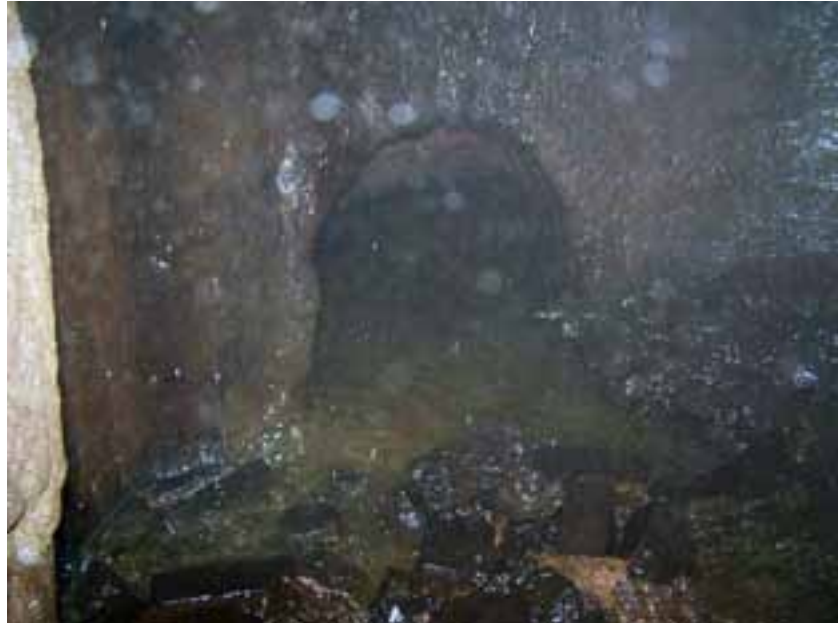
Figure 13: Low entrance to blast receiver shaft, seen from inside shaft, looking south-east (after Cordon 2006, image 64) © Tina Cordon, reproduced with permissions
