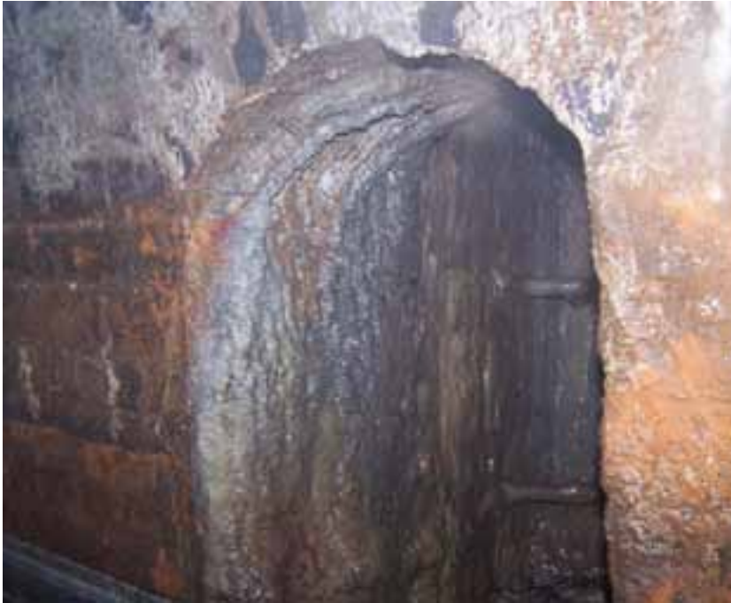
Figure 15: Entrance to narrowed vertical shaft, showing iron rungs (after Cordon 2006, image 82), © Tina Cordon, reproduced with permissions
