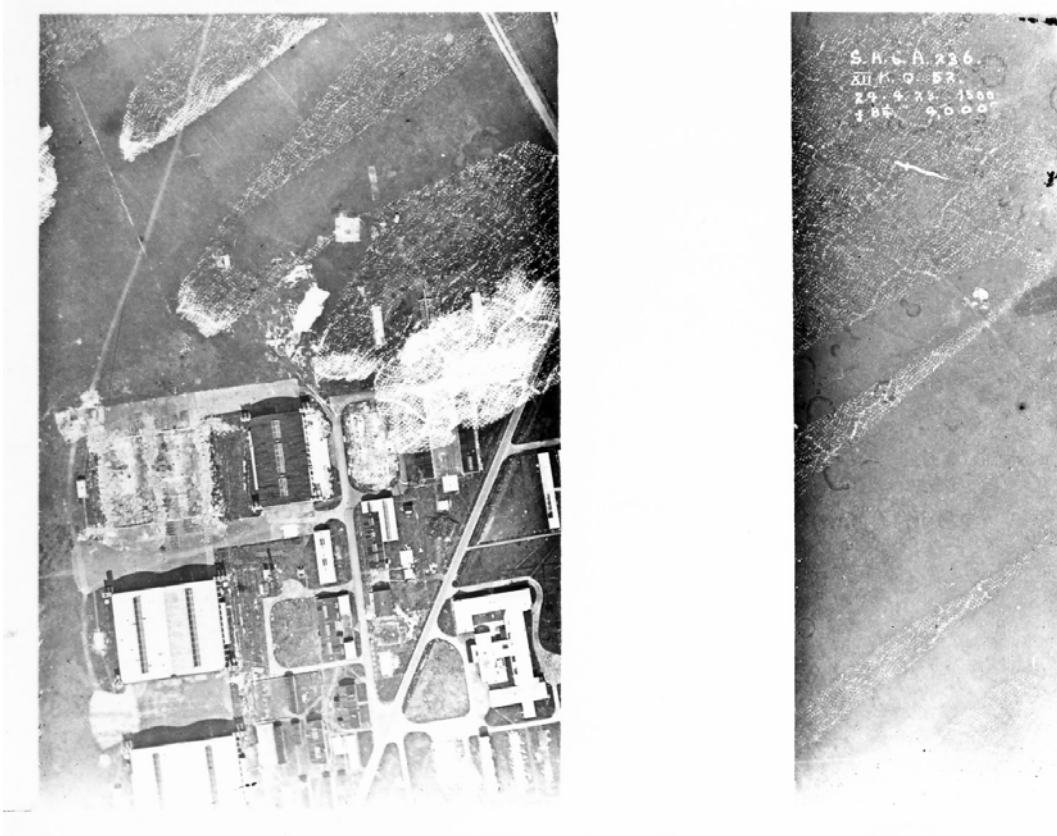
Figure 20: RAF vertical, 24 th April 1923 – print from a damaged glass plate showing evident signs of repair, including traces of adhesive tape. 11 months on from the auction, and the process of dismantling at least some of the buildings has clearly begun. The easternmost hangar, far left of centre, has disappeared, presumably removed almost entirely by whoever bought it at the auction, as have a couple of the smaller buildings on the Domestic Site (bottom centre, immediately left of the white strip). A number of the smaller structures within the Technical Site also seem to have been removed. Obviously this is a far from ideal image, but there is little sign of activity. English Heritage Archive Crawford Collection SU 1141/6 24 April 1923.
