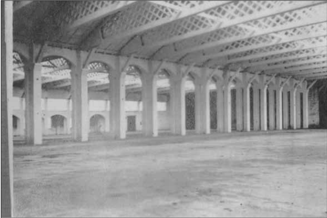
Figure 20: Interior of Building 17 photographed in 1923 (© Hooton Park Trust).
