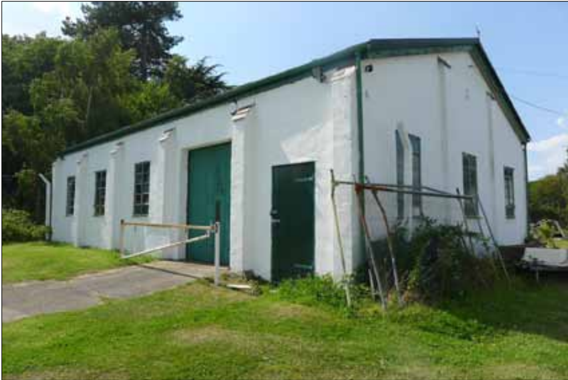
Figure 29: Building 42 from the south-east (© English Heritage, photograph: Clare Howard).
