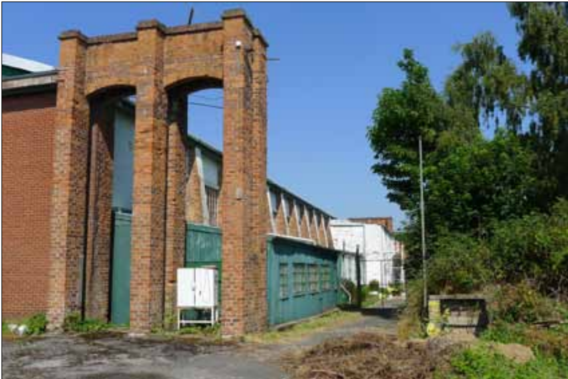
Figure 23: Annexes, north-east elevation of Building 17 (© English Heritage, photograph: Clare Howard).
