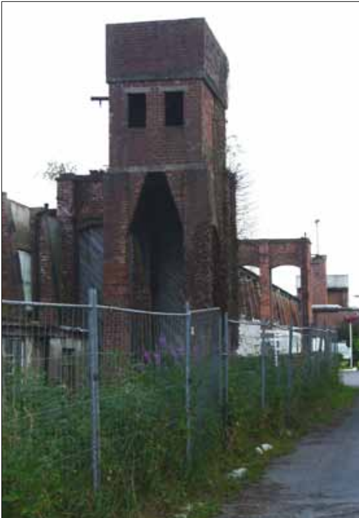
Figure 22: Tower above the gantry, Building 16 (© English Heritage, photograph: Simon Taylor).
