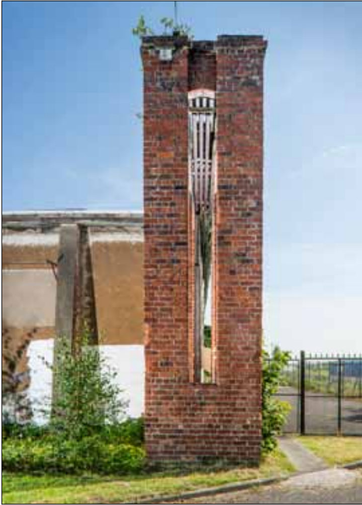
Figure 13: Door gantry on Building 18 (DPI68364 © English Heritage, photograph: Alun Bull).
