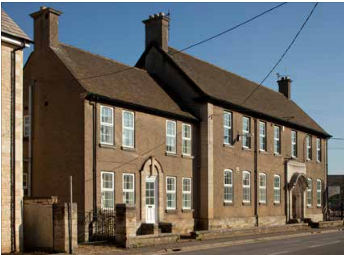
Fig 77 A handsome drill hall of c.1930 with attached staff house in Oundle. © English Heritage DPI56073
