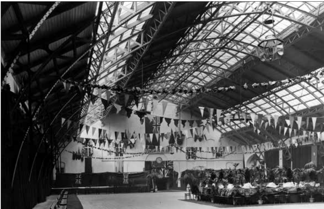
Fig 12 The interior of Sheffield's Edmund Road drill hall showing the cast-iron latticed trusses by Andrew Handyside. © Sheffield City Council, Libraries Archives and Information: Sheffield Local Studies Library Picture Sheffield: s07477
