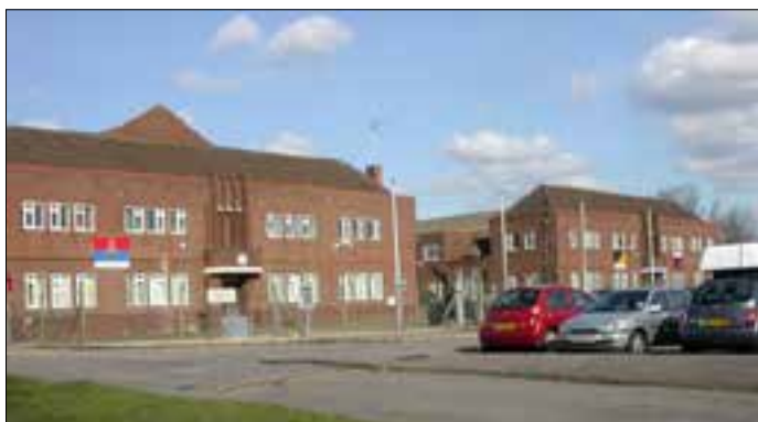
Fig 94 Blighmont drill hall in Southampton is actually a pair of drill halls built c.1939 for anti-aircraft and searchlight divisions, each with its own hall and facilities. © Mike Faherty. This work is licensed under the Creative Commons Attribution- Share Alike 2.0 Generic Licence
