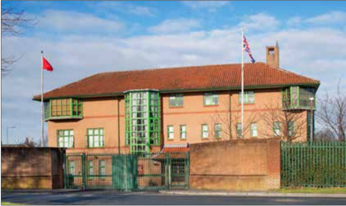
Fig 103 Chavasse House, Liverpool – the late 21st century once again saw greater variation in the design of drill halls but they can often still be mistaken for office buildings of the period. © English Heritage DPI66573
