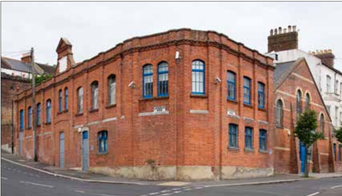
Fig 22 The 1973 drill hall in St-Leonards-on-Sea has an unusual plan with the hall lying beside the front block, which itself varies in height due to topography. © English Heritage DPI66098
