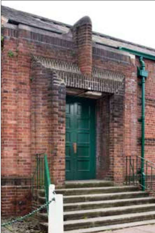
Fig 88 The highly distinctive and lively door-surrounds of Crewe's drill hall. © English Heritage DPI66576
