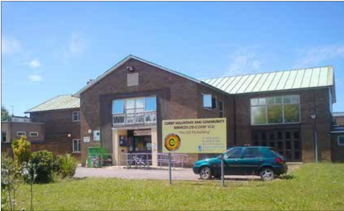
Fig 102 The drill hall on Elizabeth Street, Corby, was built in 1967 and is reminiscent of contemporary church design. © Martin Jeffs
