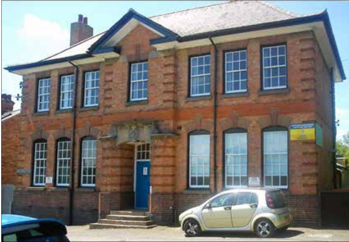
Fig 68 The drill hall on Penn Street, Oakham, was built in 1914 and displays typical features of the modified Wrenaissance style, such as rusticated brick quoins, hipped roof and sash windows. © Martin Jeffs
