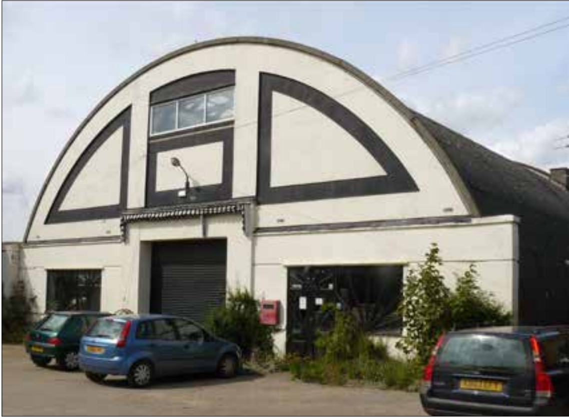
Fig 97 The c.1930 drill hall in Southwold is one of a few based on geodesic barrel designs. © Wayne Cocroft
