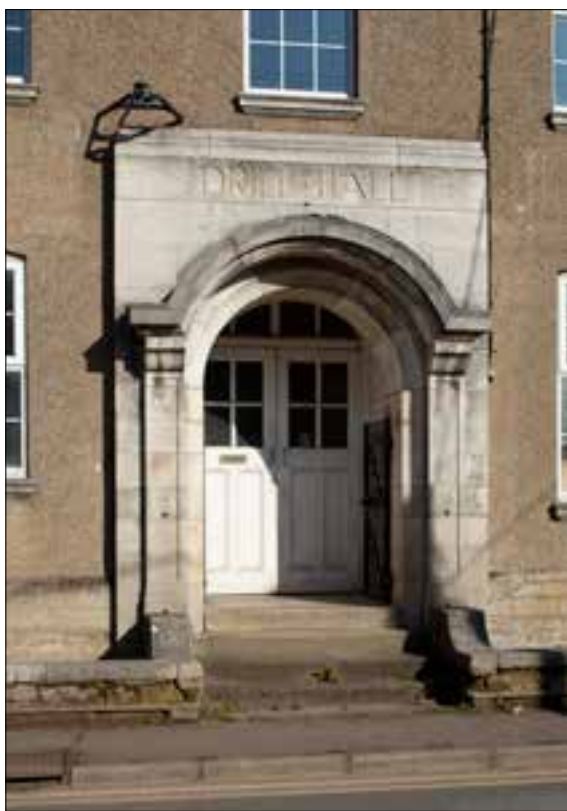
Fig 78 The door surround of Oundle's drill hall. © English Heritage DPI56076
