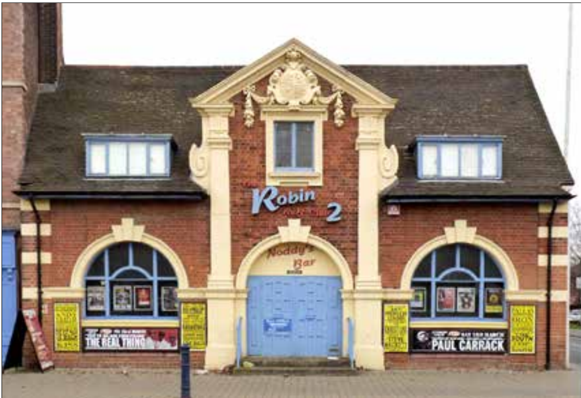
Fig 52 An unusual Neo-Baroque drill hall of 1902 in Bilston. © Alan Murray-Rust. This work is licensed under the Creative Commons Attribution-Share Alike 2.0 Generic Licence
