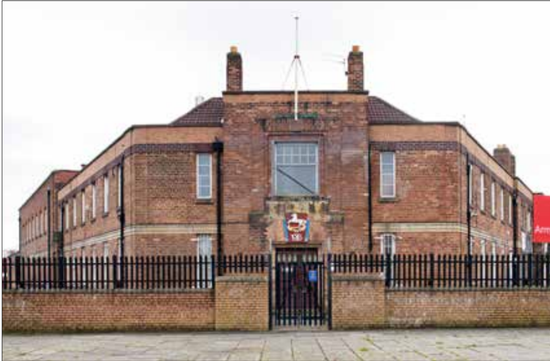
Fig 83 Townsend Avenue drill hall, Liverpool, situated on an acutely angled site and built in 1936 with hints of the fashionable moderne style © English Heritage DPI66593
