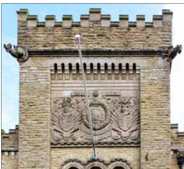
Fig 17 A detail of the crest above the entrance of the 1907 extension to Bury drill hall. © John Minnis
