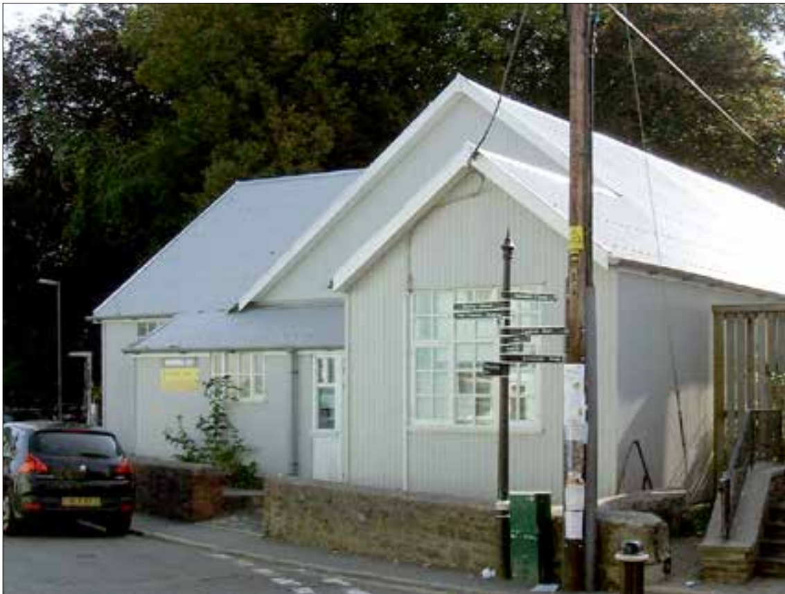
Fig 71 The 1914 drill hall in Lostwithiel is an unusual corrugated iron design, a building form more commonly associated with hospitals and churches. © John M. This work is licensed under the Creative Commons Attribution-Share Alike 2.0 Generic Licence
