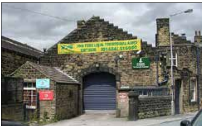
Fig 15 Keighley's drill hall, built in or before 1867 is another example of a typically modest early drill hall, built using local materials. © Betty Longbottom. This work is licensed under the Creative Commons Attribution-Share Alike 2.0 Generic Licence
