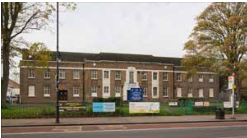
Fig 84 Tottenham High Road drill hall, 1938. A typical large 1930s design with long two-storey front block. © English Heritage DPI72149
