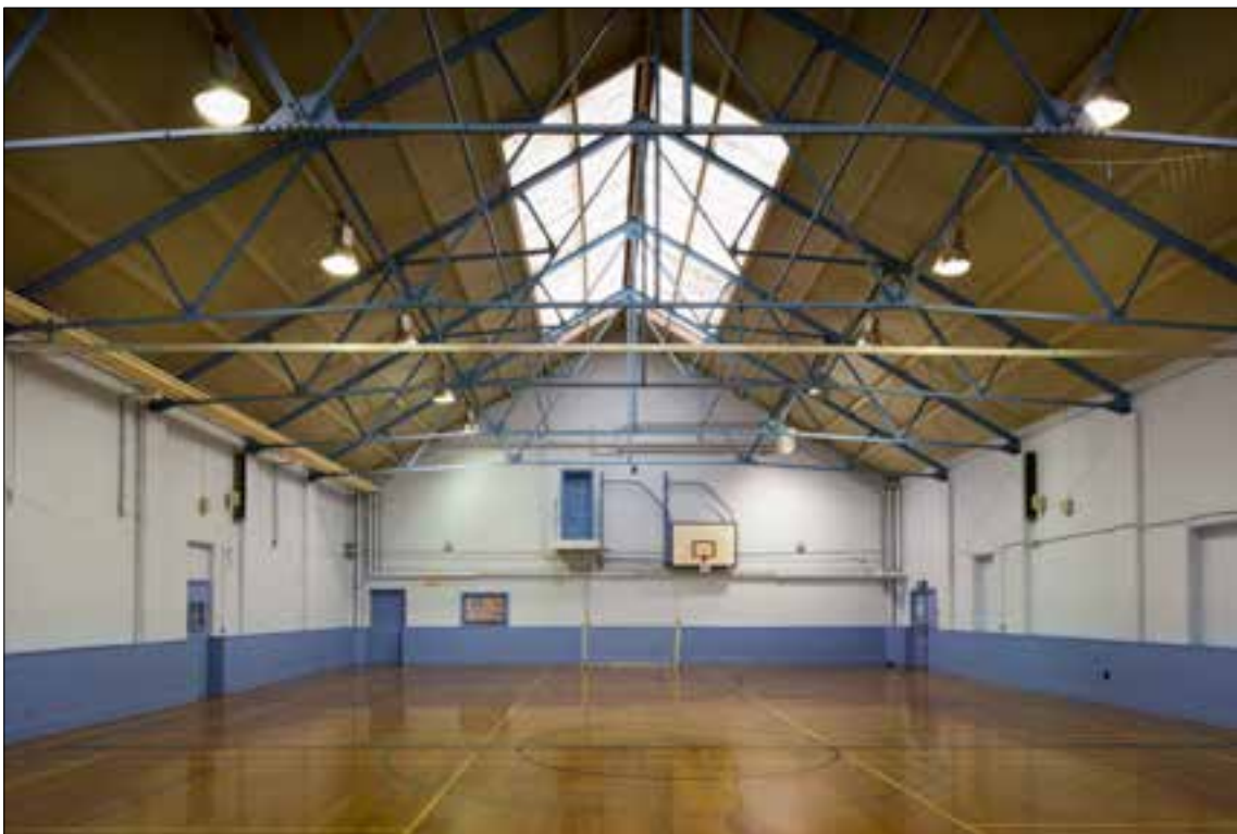
Fig 86 The interior of the hall at Tottenham drill hall with the typically slender Belgian form roof trusses of the period. © English Heritage DPI72153
