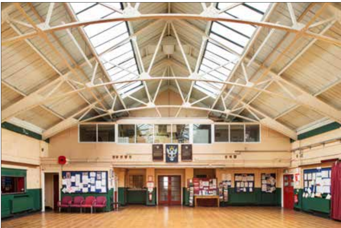
Fig 89 The interior of the hall on Myrtle Street, Crewe, with enclosed balcony. The curving iron trusses are of the Belgian form and the floor appears to be original parquet. © English Heritage DPI66583
