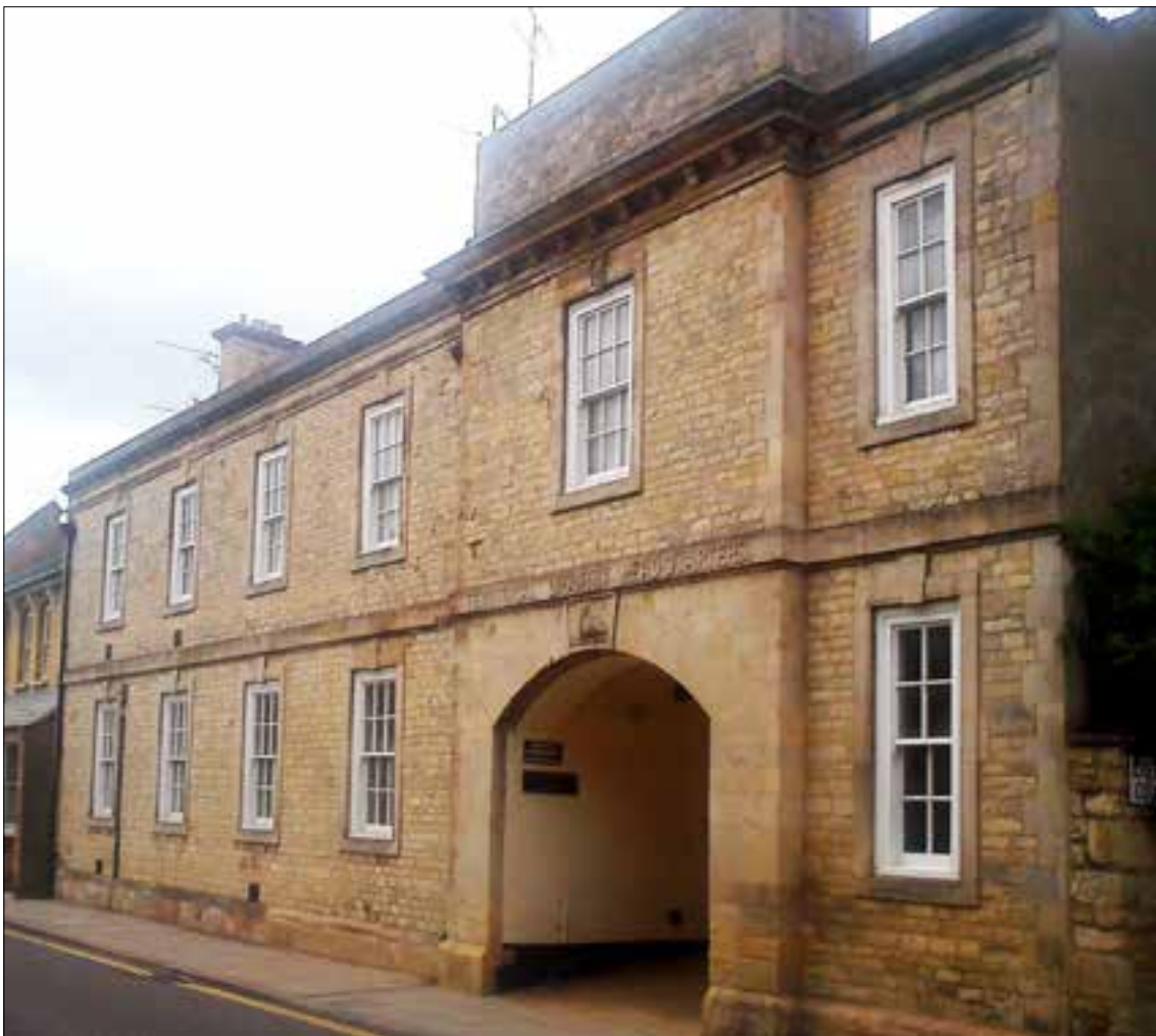
Fig 63 St Peter's Street, Stamford – the hall itself has been demolished but the front block, built in 1913, remains. © Martin Jeffs
