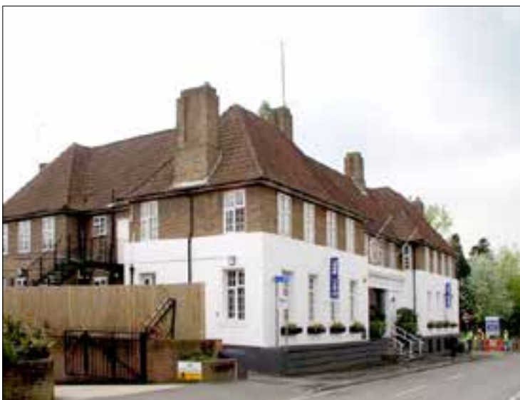
Fig 72 Horsham drill hall, 1922 – one of the first new drill halls to be constructed following the First World War. © Andy Potter. This work is licensed under the Creative Commons Attribution-Share Alike 2.0 Generic Licence
