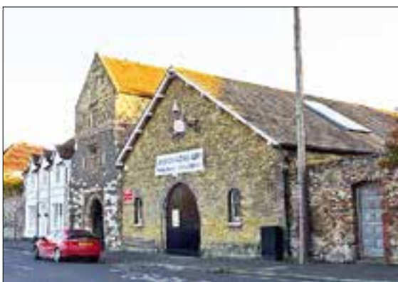
Fig 18 The drill hall in Sandwich, built in 1869, is a simple building with subtle Gothic Revival touches. © Rose and Trev Clough. This work is licensed under the Creative Commons Attribution-Share Alike 2.0 Generic Licence
