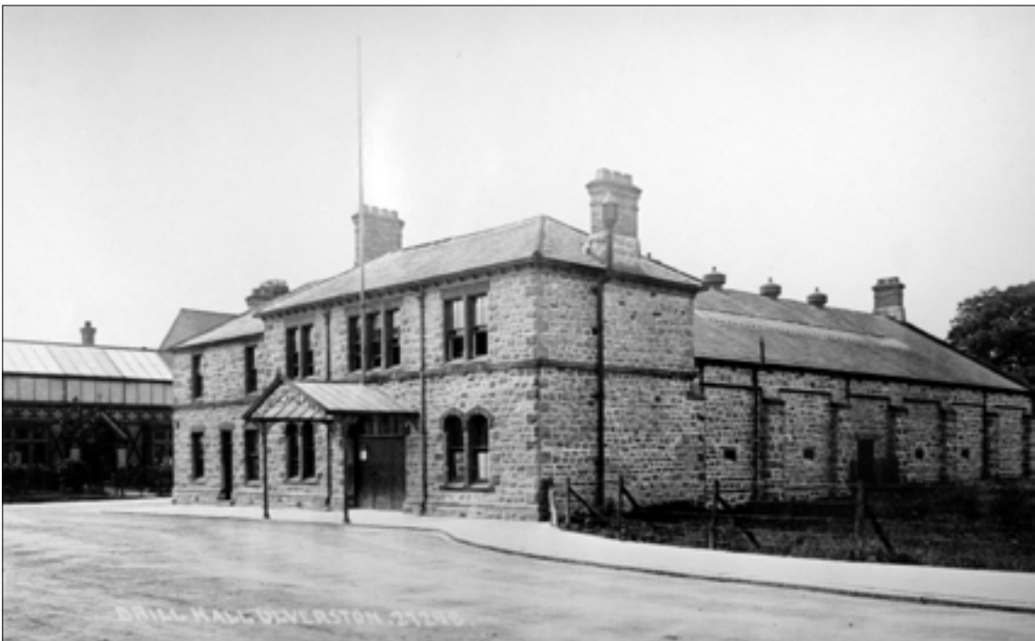
Fig 20 An undated photograph of the c.1873 drill hall in Ulverston, showing the attached staff house, rear hall and a (since removed) entrance canopy with flagpole. Reproduced courtesy of King's Own Royal Regiment Museum, Lancaster
