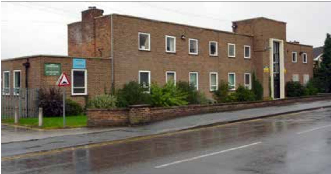
Fig 100 An example of the increasing move towards utilitarian buildings in the mid-to-late 20th century can be seen in Retford, built 1956. © Andrew Hill. This work is licensed under the Creative Commons Attribution-Share Alike 2.0 Generic Licence
