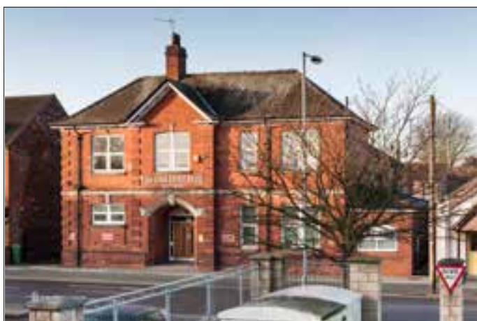
Fig 64 Cole Street drill hall, Scunthorpe. Built in to a Neo-Georgian design also seen in Spalding and Boston. © English Heritage DPI52490
