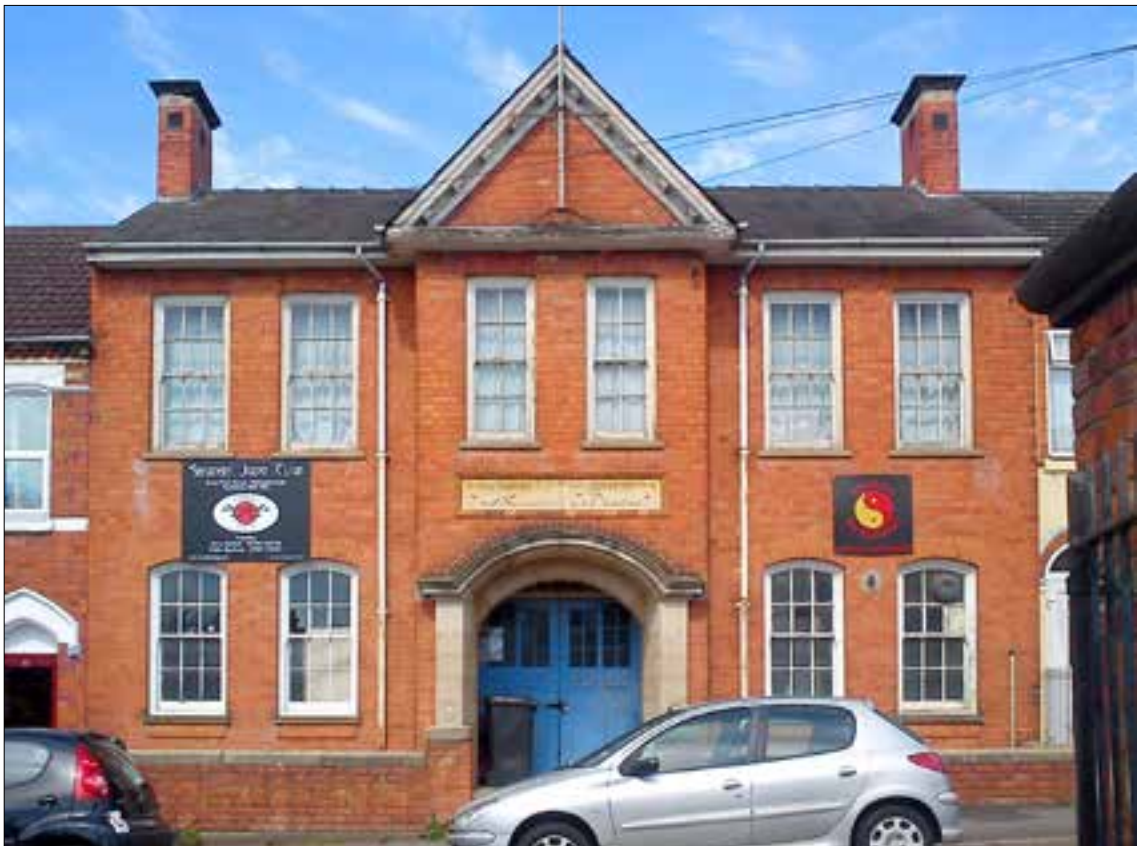
Fig 75 The neo-Georgian drill hall of c.1924 in Wellingborough is strikingly similar to that seen in Rushden, built c.1928. © Martin Jeffs
