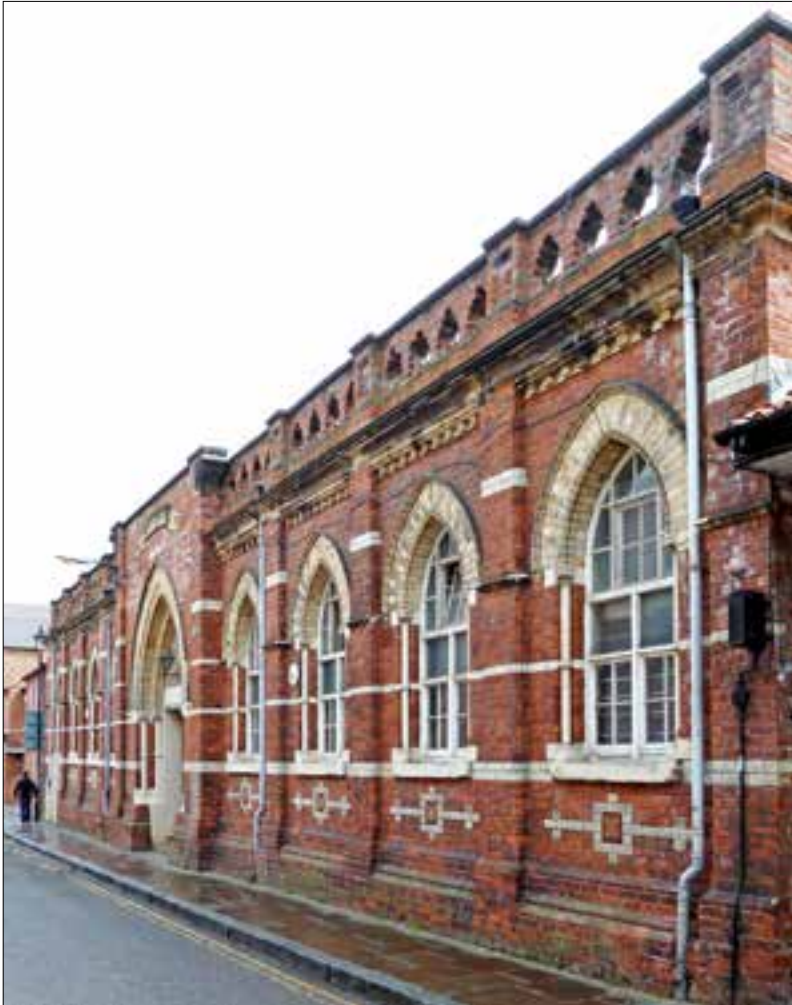
Fig 8 The drill hall on St Andrewgate, York was built in 1872 with fine polychromatic brickwork and foliate capitals. © Tim Green aka atoach. This work is licensed under the Creative Commons Attribution-Share Alike 2.0 Generic Licence
