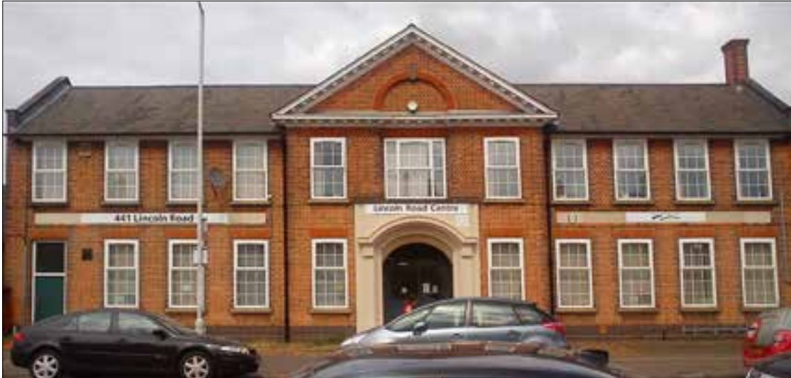
Fig 76 The 1927 drill hall on Lincoln Road, Peterborough, is an expanded version of the form already seen at Wellingborough and elsewhere. © Martin Jeffs
