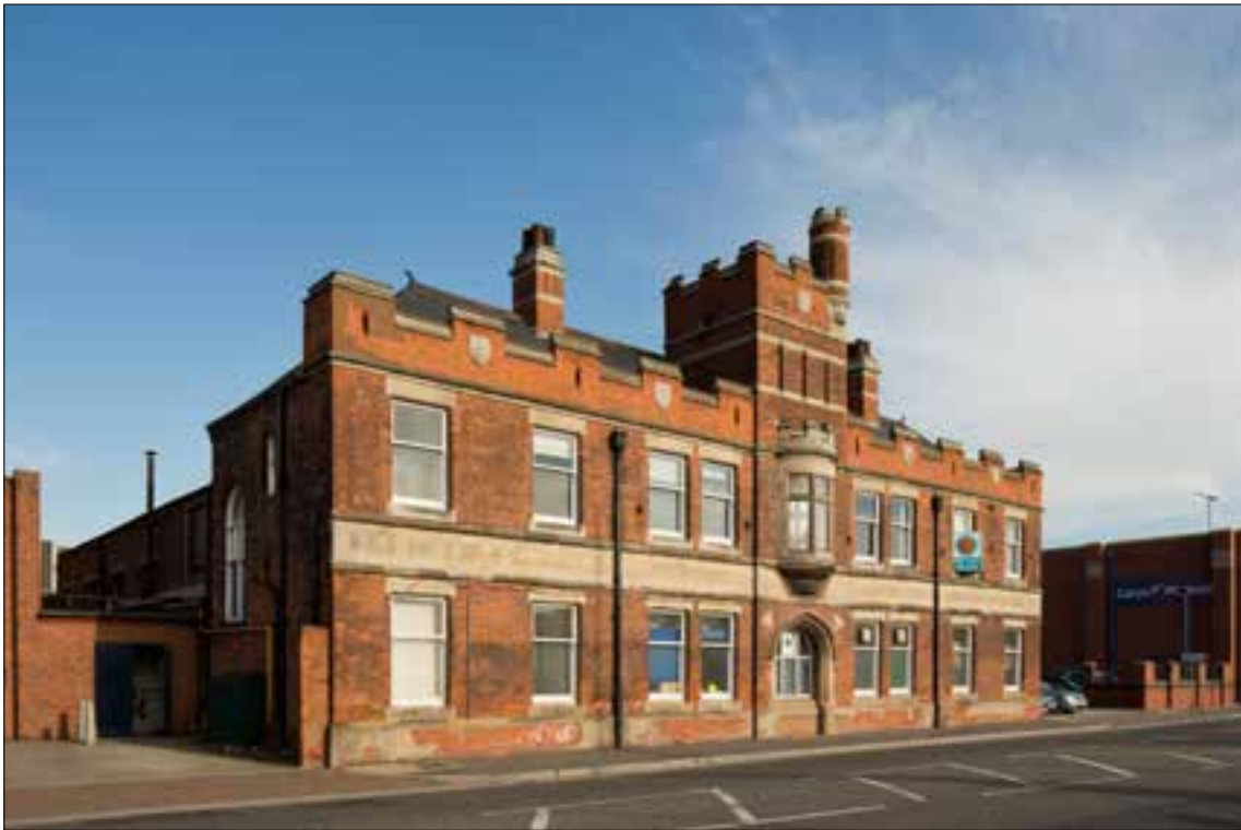
Fig 43 The front block of Grimsby's drill hall was designed in the Tudor revival style in the 1890s. © English Heritage DPI72155
