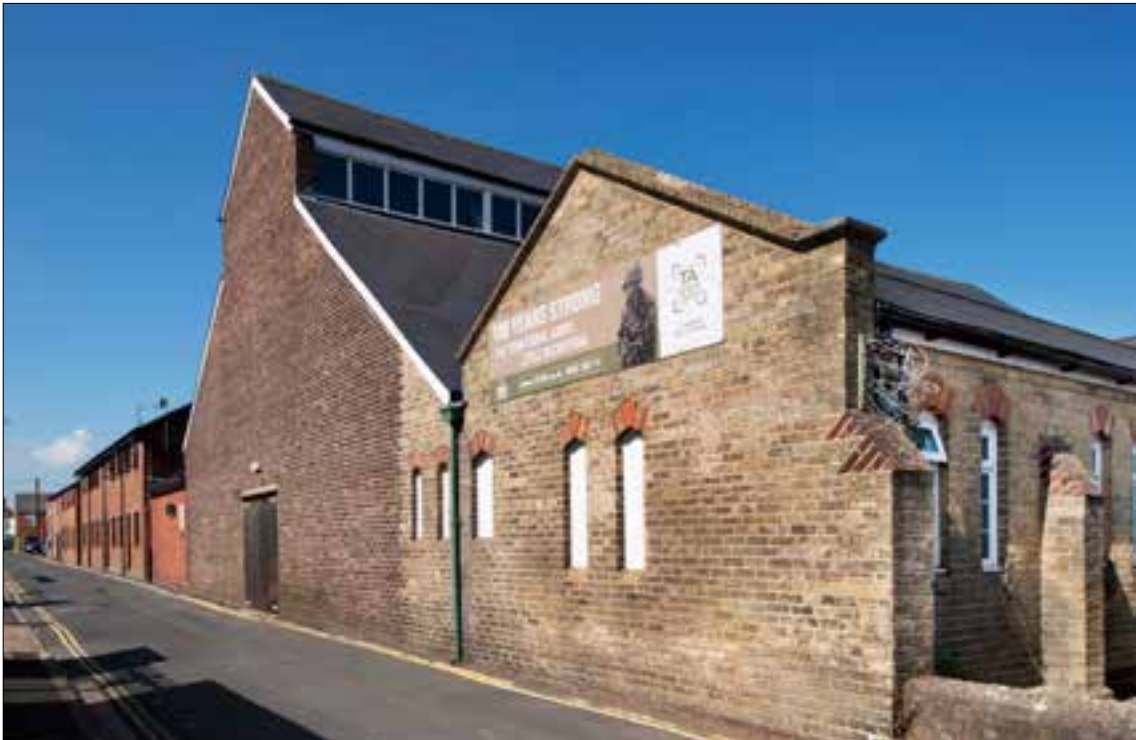
Fig 21 The drill hall in Newport, Isle of Wight, with buttresses and polychromatic brick heads to the front block and a simple hall with raised ridge lantern beyond. © English Heritage DPI66101
