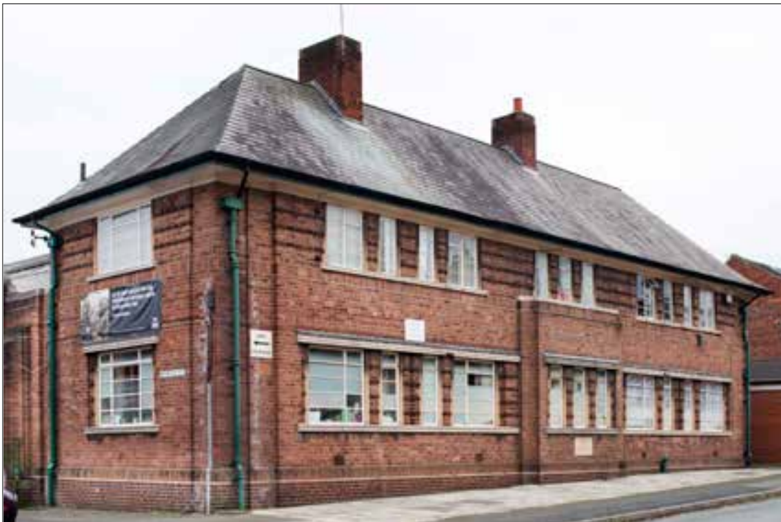
Fig 87 The Myrtle Street drill hall in Crewe was built in 1937 and is an unusual example of a drill hall built to a design which is clearly influenced by the moderne style. The steel-framed windows are connected by heads and sills which curve in a streamline manner whilst horizontal brick banding at first-floor level emphasises the horizontal elements of the façade. © English Heritage DPI66577
