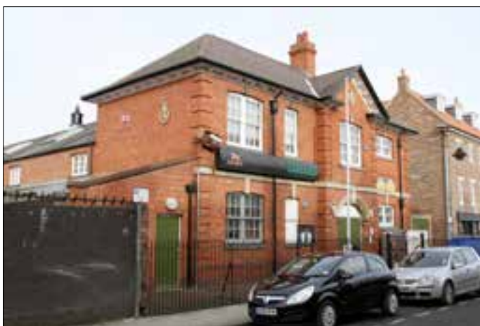
Fig 66 The second drill hall on Main Ridge West, Boston, was built in 1914 and is one of a number of drill halls designed by Scorer & Gamble. © John Minnis
