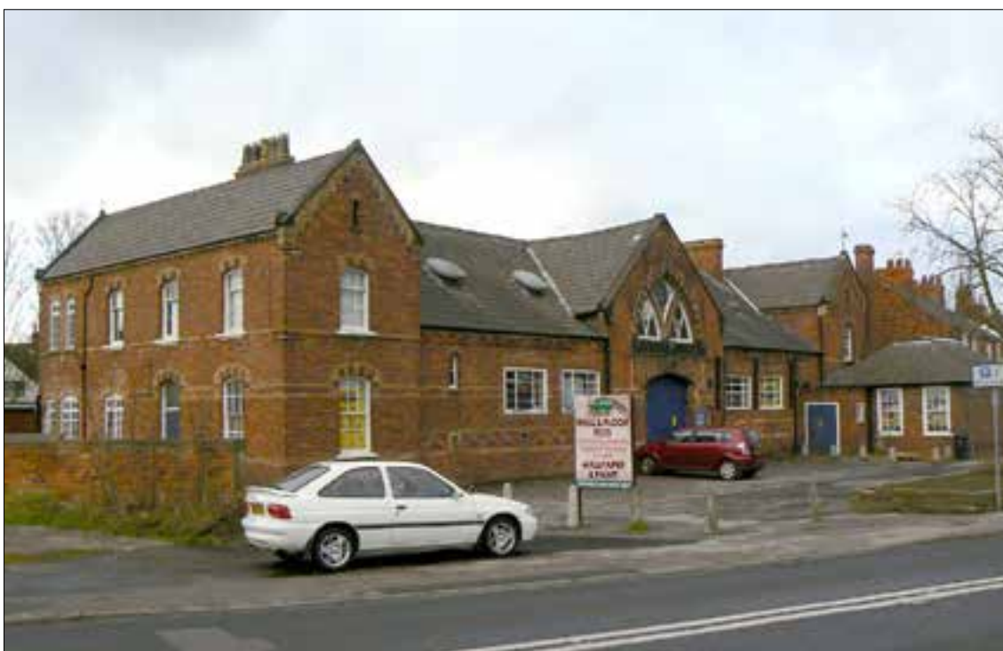
Fig 2 The drill hall on Armoury Road, Selby, built 1864-5 is the oldest listed drill hall in the country. © Alan Murray-Rust. This work is licensed under the Creative Commons Attribution-Share Alike 2.0 Generic Licence
