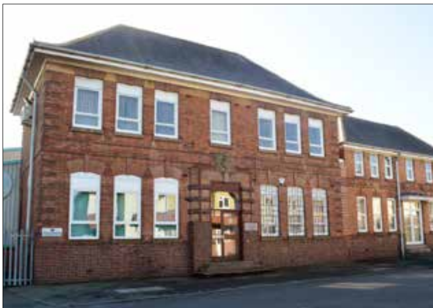
Fig 68 The drill hall on Penn Street, Oakham, was built in 1914 and displays typical features of the modified Wrenaissance style, such as rusticated brick quoins, hipped roof and sash windows. © Martin Jeffs
