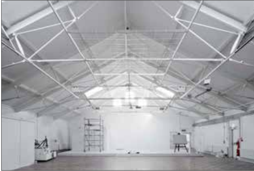
Fig 24 The interior of Grove's Easton Road drill hall. © English Heritage DPI66092
