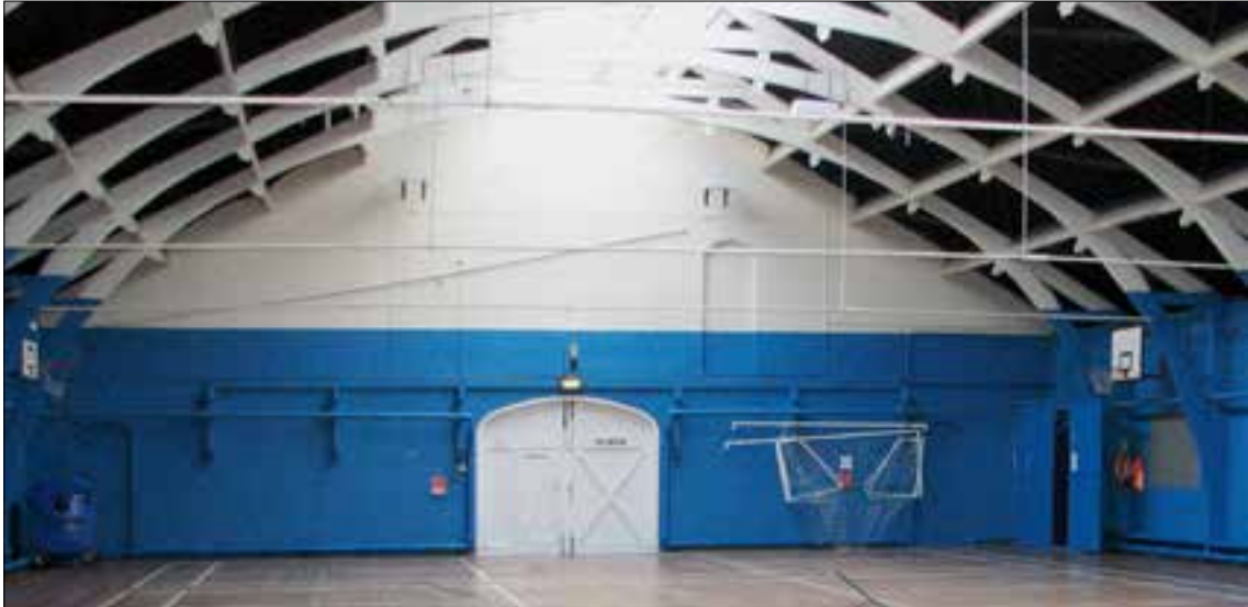
Fig 5 The interior of Great Yarmouth's drill hall with its unusual elliptical roof trusses and a blocked doorway which led to the former balcony, the supports for which are still visible. © Katie Carmichael
