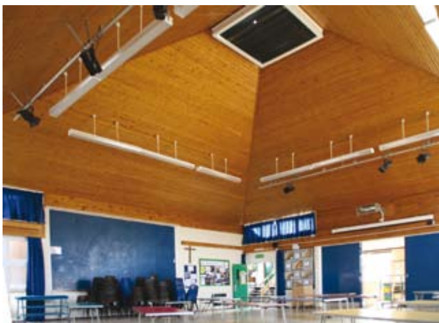
Figure 4.187: A timber shell roof at St Mary's Primary School, Hadleigh; Johns Slater and Haward, 1966-67 (P5925026).
