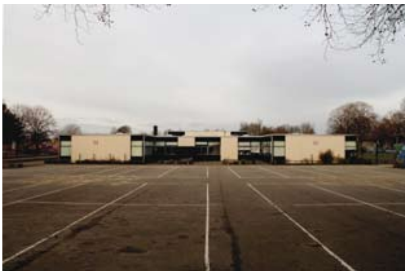
Figure 4.198: Westley Middle School (P5925030).
