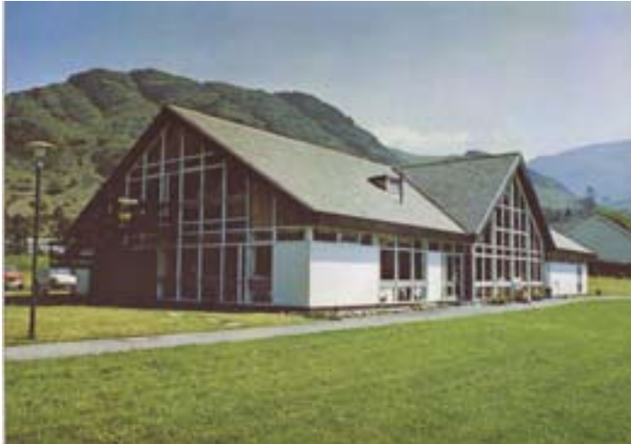
Figure 4.222: Pitched slate roofs were encouraged in scenic locations. Reproduced by kind permission of Lancashire County Council.
