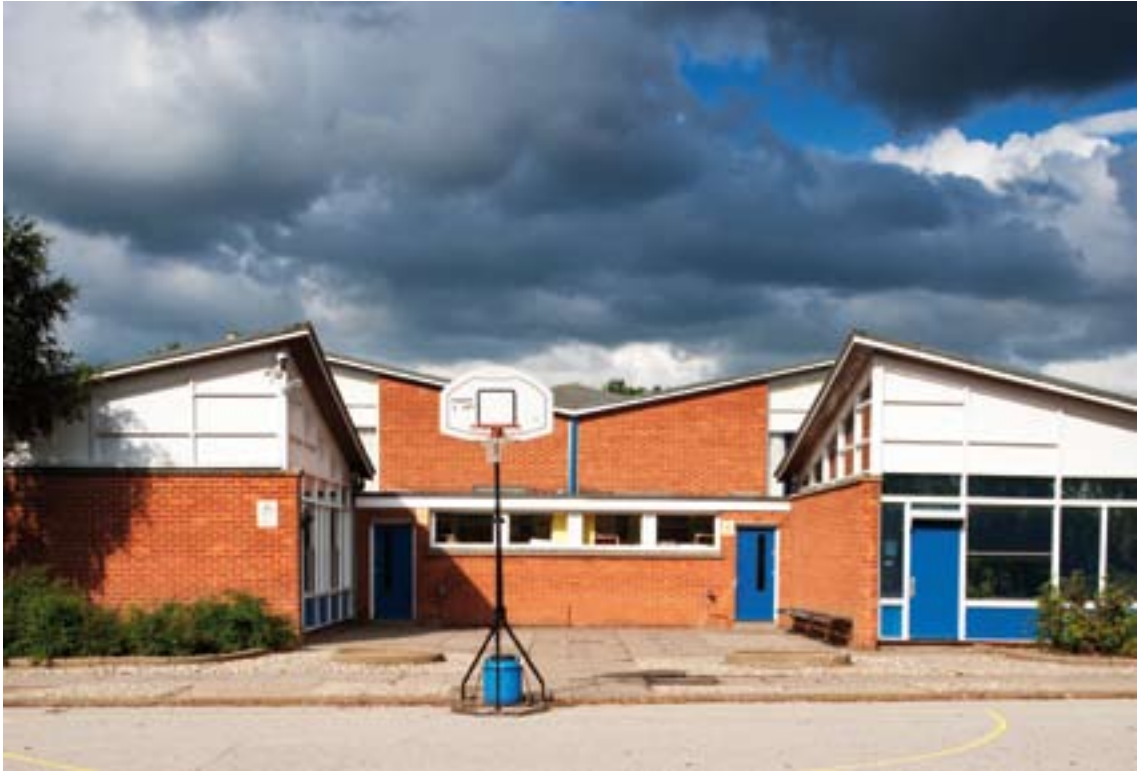
Figure 4.203: Sprites Lane Primary School, Chantry, Ipswich; Johns, Slater and Haward, 1958-60. Photograph by James O. Davies – English Heritage; DPI38300.
