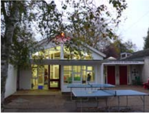
Figure 4.251: South east elevation of the Cringleford Church of England School. The main entrance is visible to the right. On the left, an infilled veranda, replicating the original glazing pattern (P5925037).
