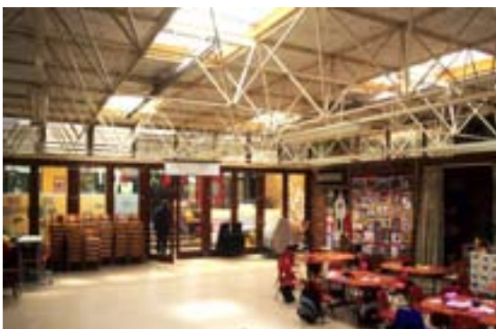
Figure 4.196: The sunken hall at Great Waldingfield with its space frame roof. © Elaine Harwood.
