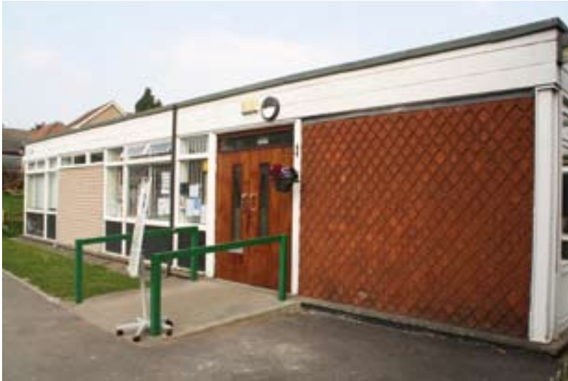
Figure 4.41: Tiling hanging at the CLASP Orchard Infant School, Sprotbrough, Doncaster; Twist & Whitley, completed 1966. Ken Twist and Ken Evans worked together at the Hertfordshire Architect's Department in the early 1950s (P5925004).
