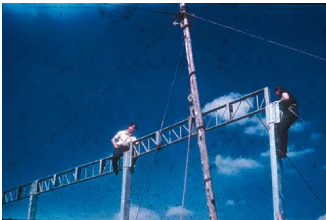
Figure 3.1: Erecting the steel frame at St Crispin's Secondary Modern School, Wokingham, built to the Hills system in 1951-53. Institute of Education Archives: ABB/B/1/75/1.
