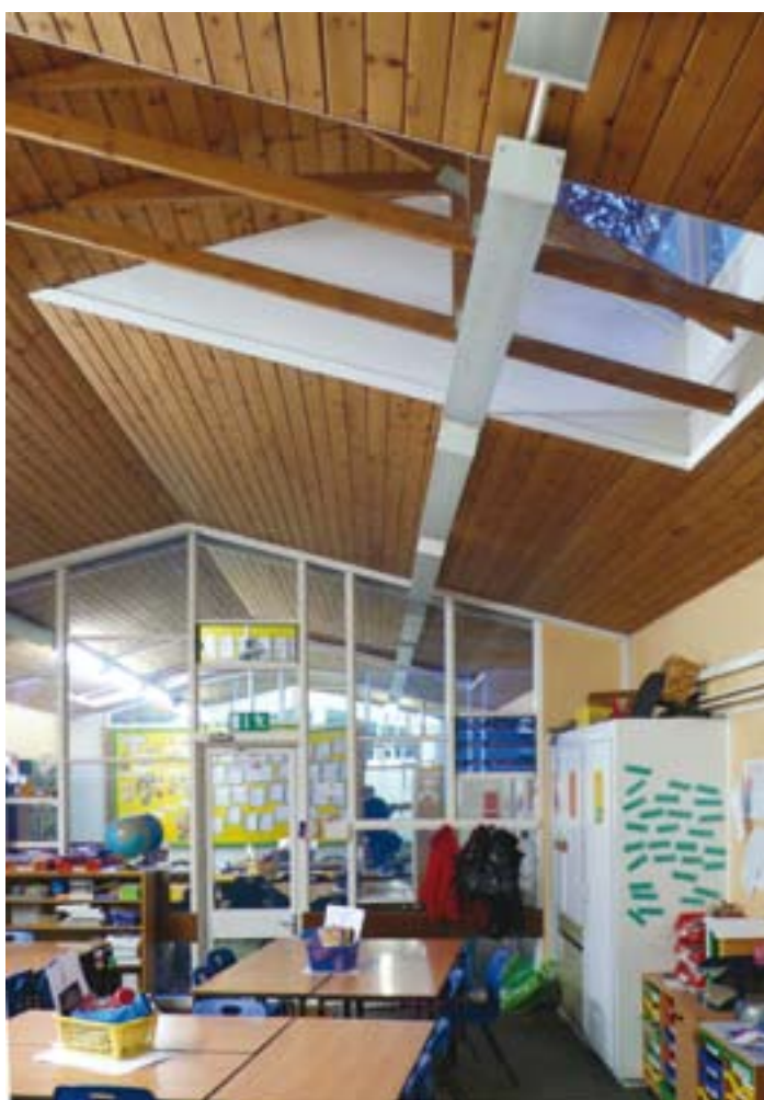
Figure 4.241: Classroom interior at Cringleford Church of England School, Norfolk; Tayler and Green, built in two stages, 1969-70 and 1973-74. Note the sloped and boarded ceiling, cut away at the dormer to expose scissor trusses. Beyond the glass partition is a shared practical area (P5925032).
