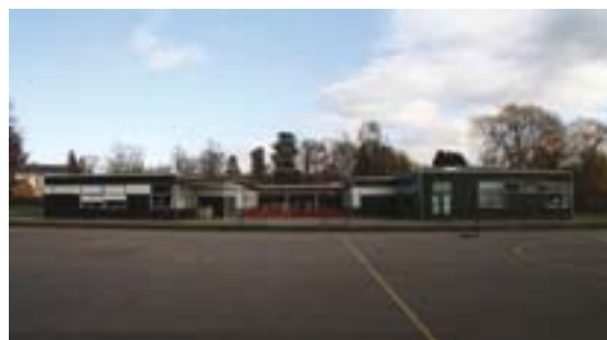
Figure 4.191: Bildeston Primary School; West Suffolk County Council, 1967-68 (P5925028).
