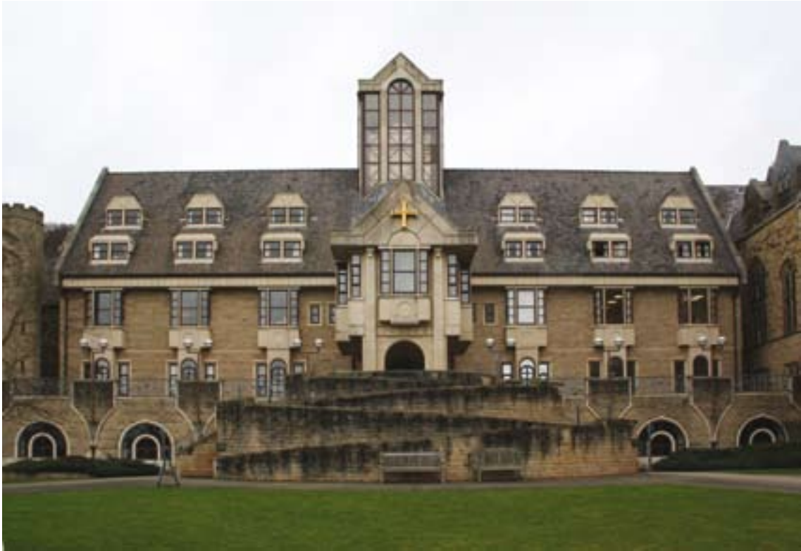
Figure 4.249: Ampleforth Centre at Ampleforth College; the Ellis Williams Partnership, 1986-88 (P5925035).
