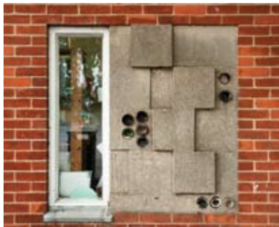
Figure 4.208: Low-relief panel at Sprites Lane. Photograph by James O. Davies – English Heritage; DPI38293.
