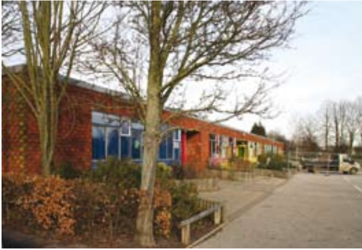
Figure 4.180: The tilehung Westgate Primary School, Bury St Edmunds, of 1968-69, built in SEAC Mark II (P5925023).
