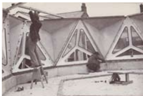
Figures 4.229 and 4.230: GRP classroom extension to Kennington Primary School, Fulwood, Preston; Lancashire County Council Architect's Department, 1973-74. A prototype of a prefabricated system in plastics, foiled by the oil crisis. Reproduced by kind permission of Lancashire County Council.
