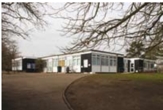
Figure 4.183: Thurston Primary School, one of several West Suffolk schools constructed in the timber-framed Derwent system (P5925025).
