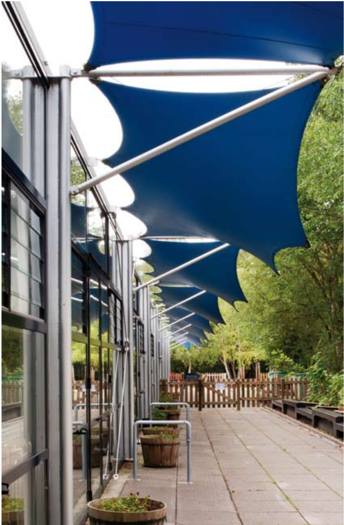
Figure 4.160: Fleet Infant School. The sail-like awning in Teflon-coated PVC is an allusion to Hopkins's initial proposal for a tent-like masted structure. Photograph by James O. Davies – English Heritage; DPI37509.
