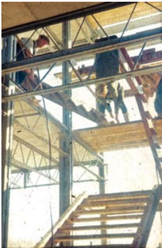
Figure 4.137: Prefabrication in practice: installing stair treads at Harrow Way Secondary School, Andover, c.1966. In a frame structure this kind of work could be completed under cover. Institute of Education Archives: ABB/B/1/216/2
