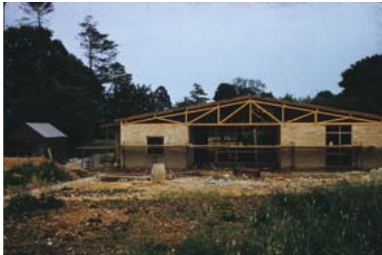
Figure 3.5: 'Rat. trad.' construction at Finmere Primary School, Oxfordshire in 1959. Lightweight, exposed timber trusses rests on load-bearing panels of brickwork; the timber-framed window-walling is last to be installed. For the plan of this school see fig. 2.4. Institute of Education Archives: ME/Z/5/2/150.
