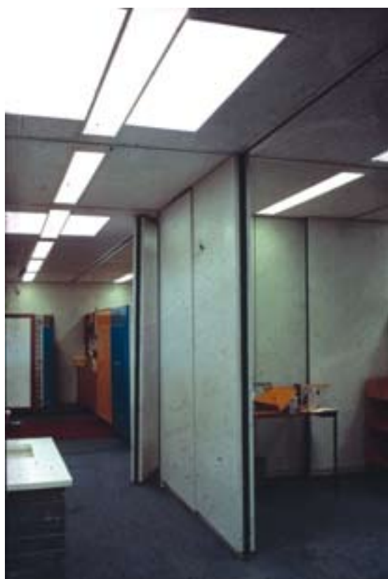
Figure 4.252: A 1970 photograph of Ilford Jewish Primary School. Note the office-like interior and 'moving wall', with its ceiling rails. Institute of Education Archives: ABB/B/1/25/2.
