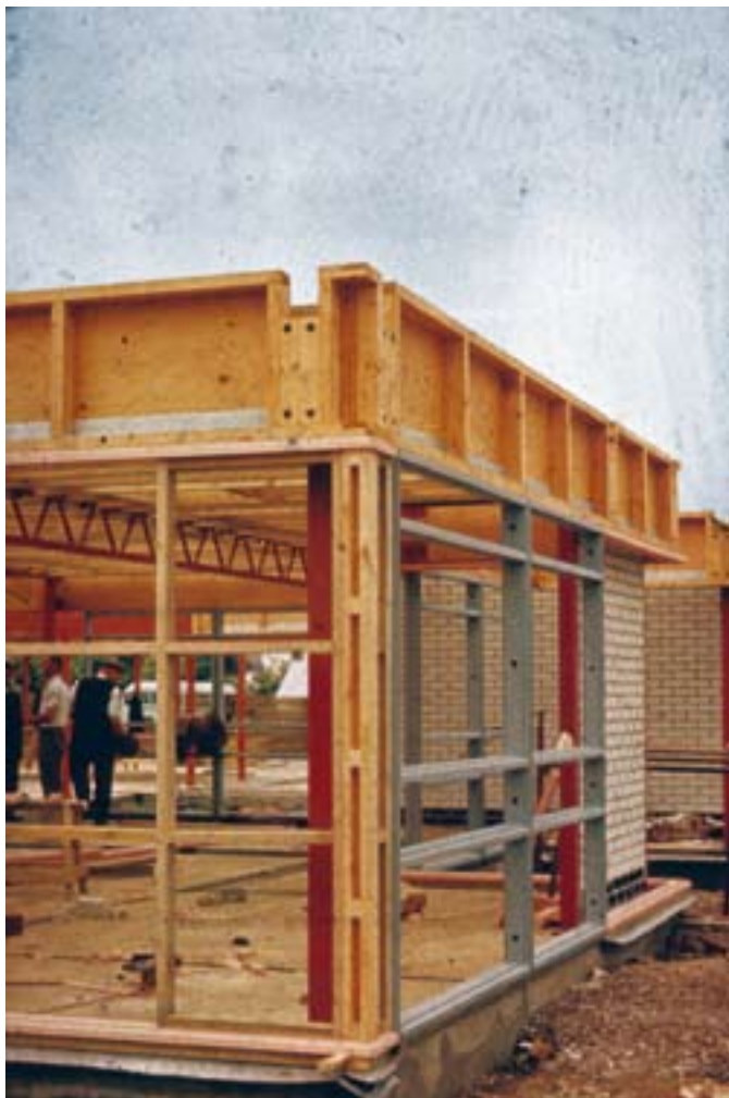
Figure 3.6: Yatton Junior School, Somerset in construction c.1967. The Consortium for Method Building employed a wide range of materials and components, some prefabricated, others assembled on site. Institute of Education Archives: ABB/B/9/14/1
