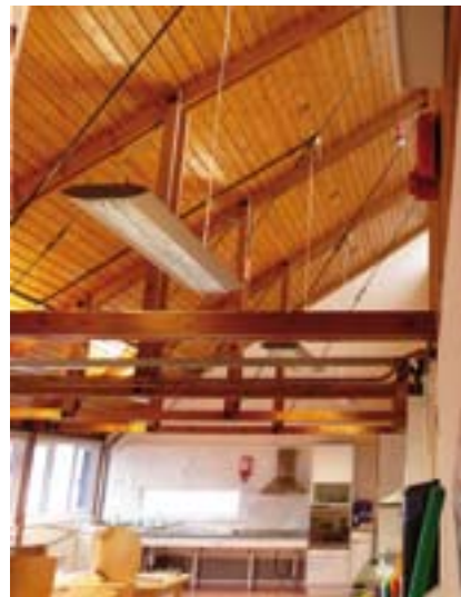
Figure 4.268: Meldreth Manor School. The school has ceiled some of the exposed trusses to improve thermal comfort (P5925042).
