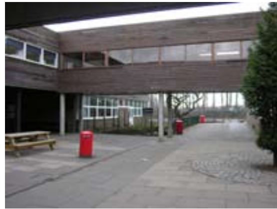
Figure 4.49: Bruntcliffe County Secondary School (P5925006).
