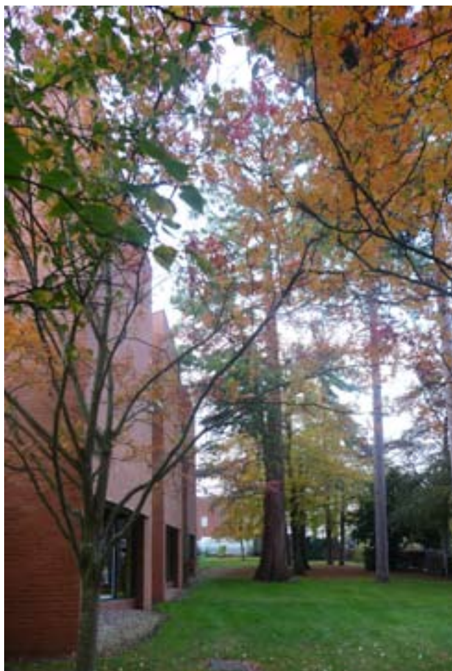
Fig: 4.240: The Scandinavian-inflected north elevation of the Library and resource centre at Millfield School, Somerset, of 1978-80 by Jeremy & Caroline Gould. Photograph by Jillian Wallis, reproduced by kind permission of Millfield School.
