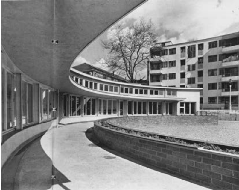
Figure 51: The Kensal House Day Nursery, with Kensal House behind; 1936-37, principal architect Maxwell Fry (English Heritage London Region photographic collection, box 476).
