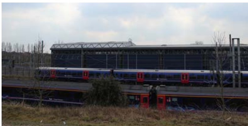
Figure 20: A view of the Eurostar maintenance shed of 1991-92 at North Pole International Depot (P6846009).
