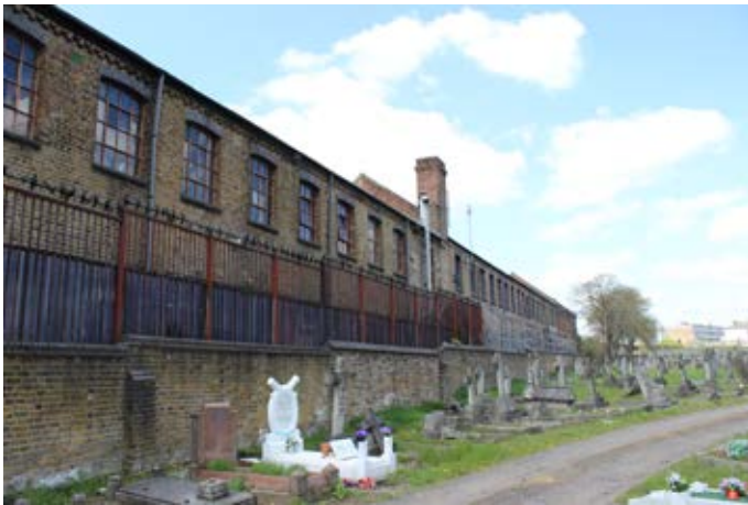
Figure 28: The rear elevations of the former Cumberland Park Factory overlook St Mary's RC Cemetery (P6846016).
