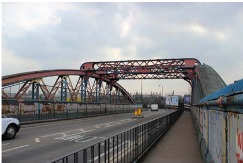
Figure 23: Early twentieth century bowstring truss bridge carrying Scrubs Lane over the Great Western main line (P6846012).
