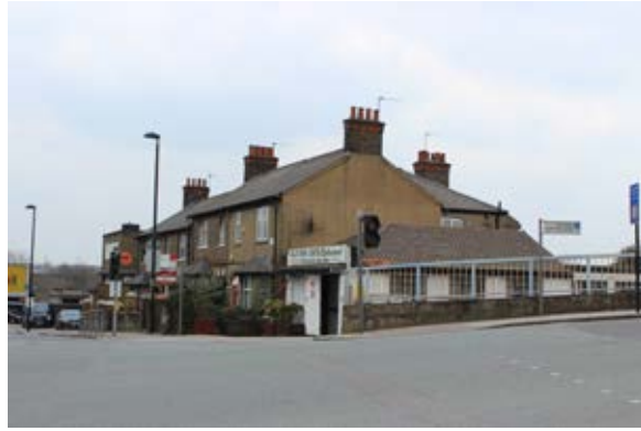
Figure 17: Victoria Terrace. To the right is the Old Oak Common Lane overbridge (P6846007).
