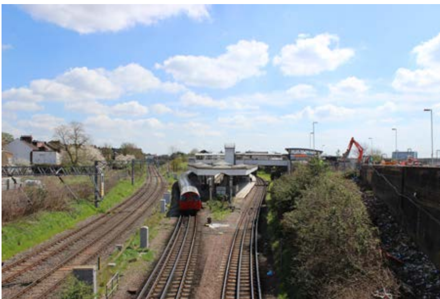
Figure 27: View of the early twentieth century low-level platforms of Willesden Junction Station, from the road bridge over the Bakerloo Line (P6846015).
