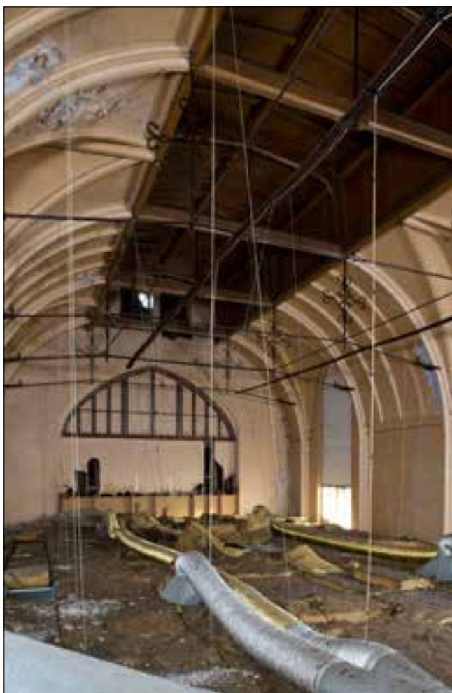
Fig 13 Roof structure and suspended false ceiling of the great hall. © Pat Payne, English Heritage, DPI61079
