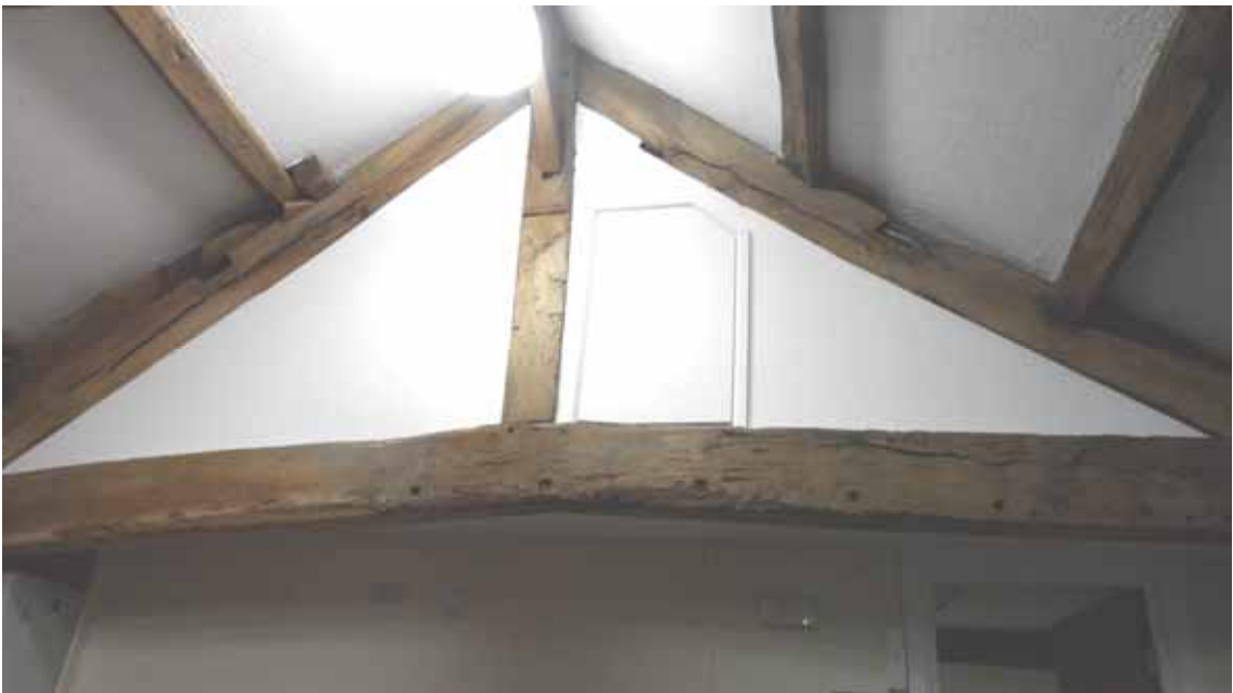
Figure 8: Stables; truss 4 with canted tiebeam, photograph taken from the west (Alison Arnold)
