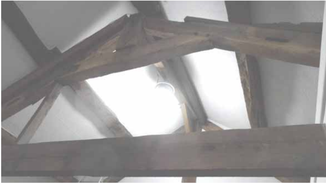
Figure 7: Stables, truss 2 with high collar and modern tiebeam, photograph taken from the east (Alison Arnold)
