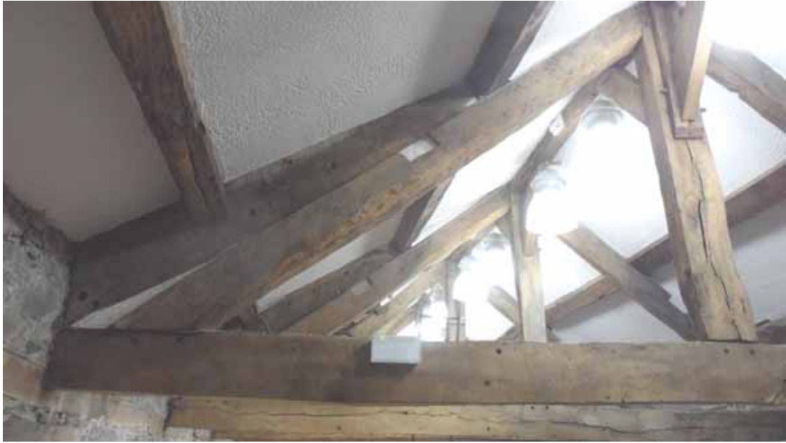
Figure 9: Stables, one of the backing rafters used to modify roof pitch, photograph taken from the west (Alison Arnold)
