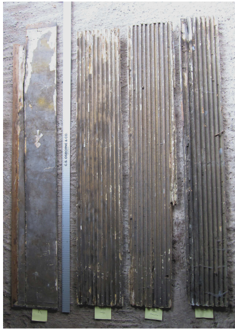
Figure 6: Larger board K, and moulded boards H, I and J (left to right) from Brooke House, Hackney; all grain running top to bottom (photograph Ian Tyers)
