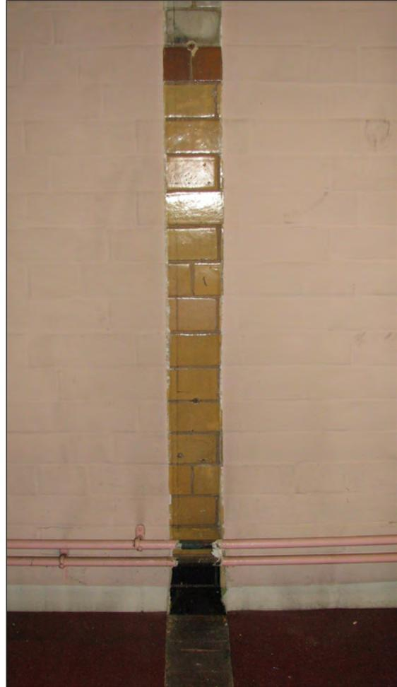
*Fig 19 An exposed strip of glazed brickwork in Clay, first floor. (K. Morrison)*
