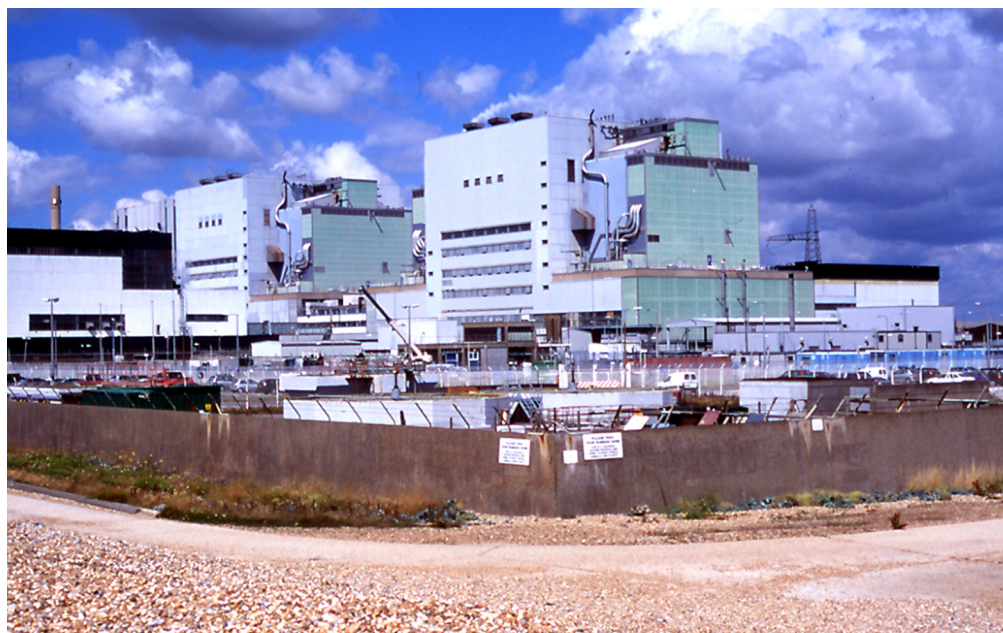
Figure 9 Dungeness, Kent, the 1960s Magnox station © W D Cocroft
