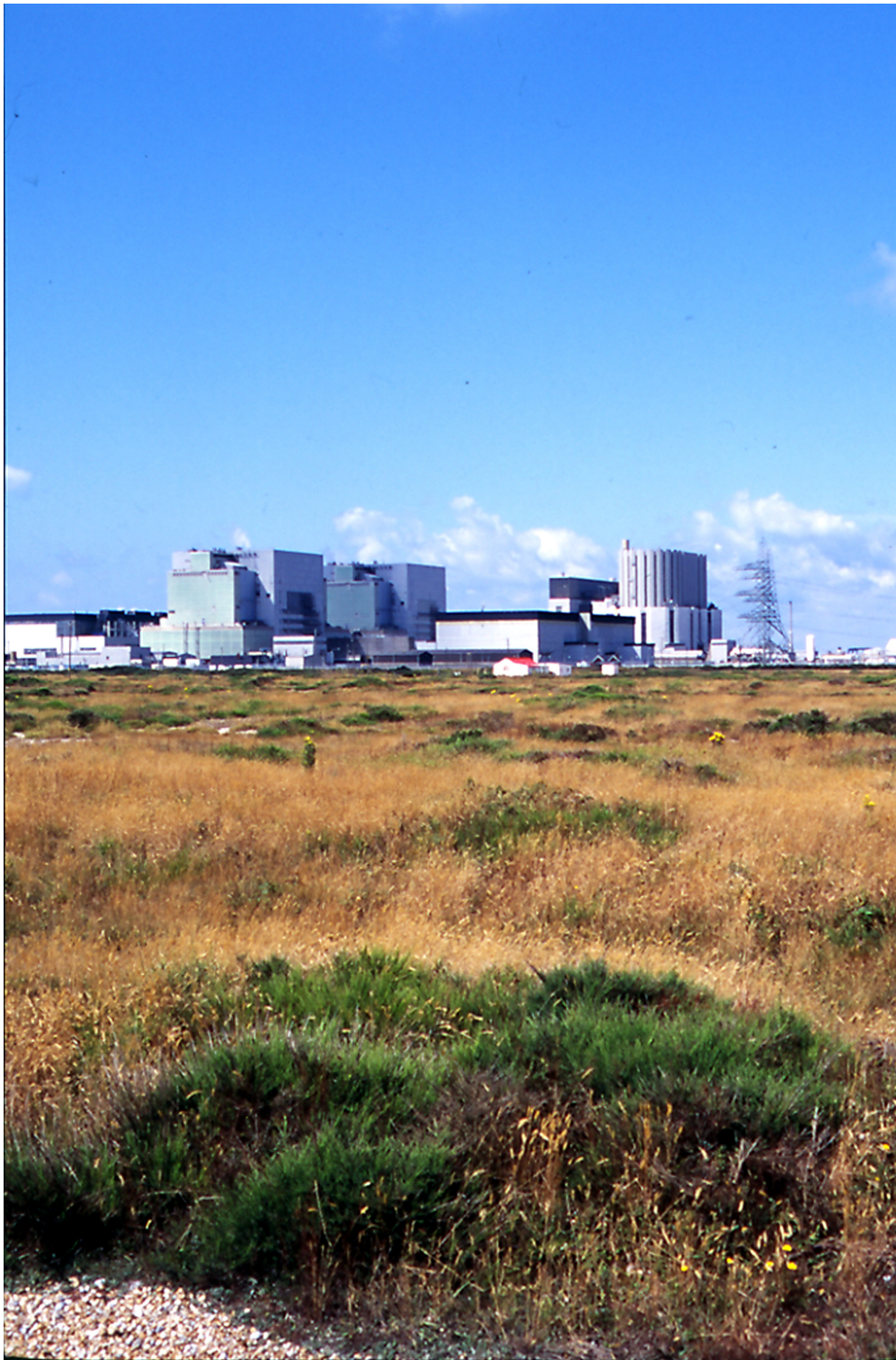
Dungeness power station (c) W D Cocroft
