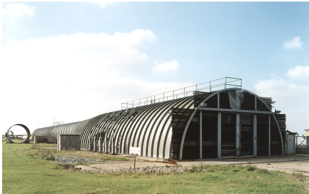
Figure 4 Foulness, Essex, air blast tunnel used in the simulation of blast waves © English Heritage BB99/15990
