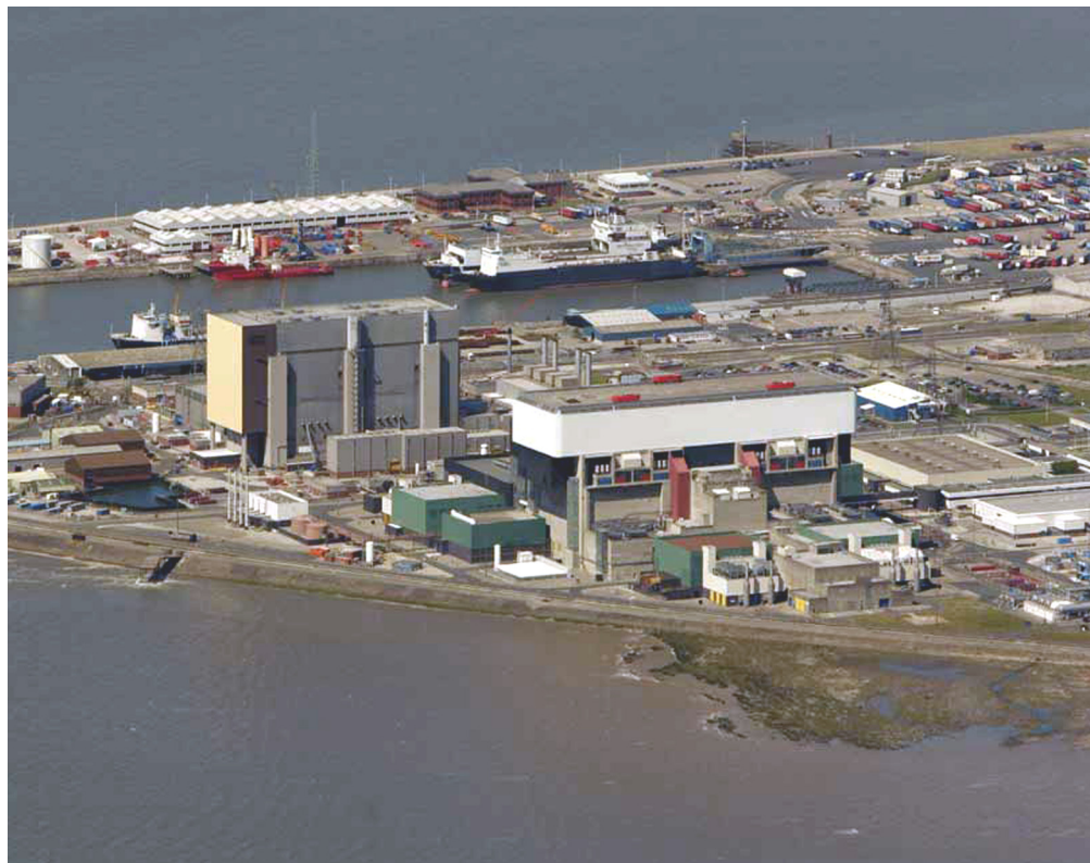
Figure 10 Heysham, Lancashire, the two Advanced Cooled Reactor stations have a combined output of 1320 MWe © English Heritage NMR 20319-015
