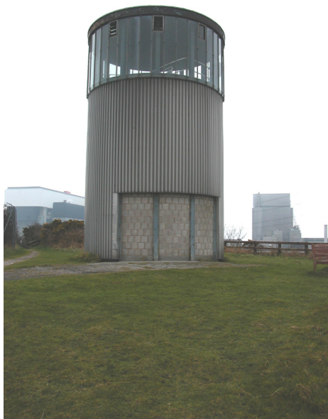
Figure 17 Heysham, Lancashire, observation tower, its entrance was bricked up after the 2001 terrorist attacks on New York © English Heritage
