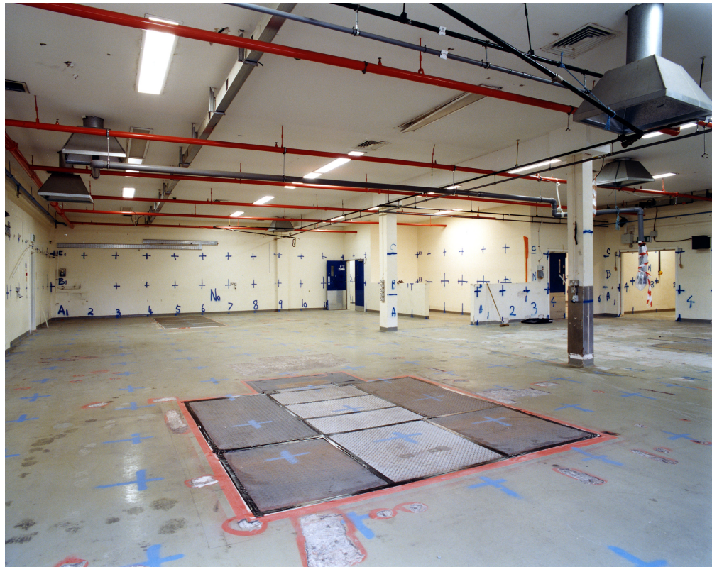
Figure 30 Featherstone, Staffordshire, Royal Ordnance Speciality Metals, one of the depleted uranium machining areas during decontamination operations © English Heritage AA05104
