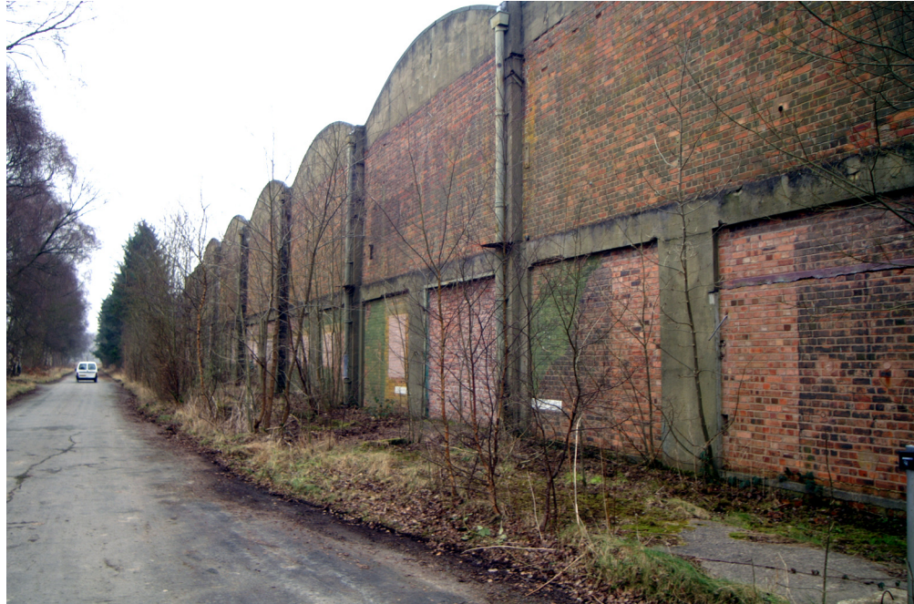
Figure 2 Rhydymwyn, Clywd, July 1997, during the Second World War building 45/P6 housed ICI's experimental isotope separation plant © Peter Bone
