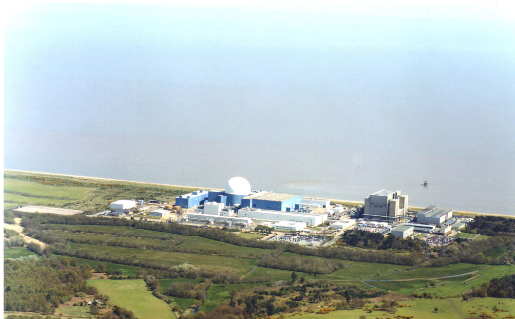
Figure 27 Sizewell, Suffolk, to the right is the 1960s Magnox station Sizewell A and to the left the is the 1200 MWE Pressurised Water Reactor © English Heritage NMR 23495/12
