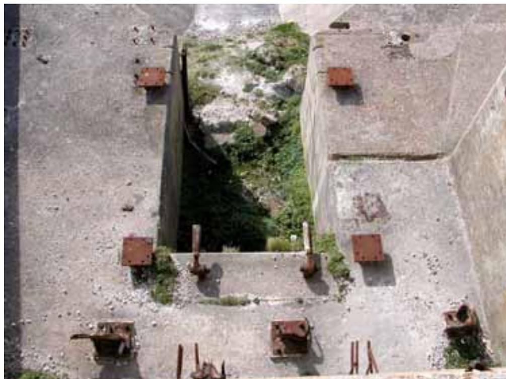
**Figure 19** Gantry 2 detail showing the fixing plate for the gantry and efflux duct beneath.
