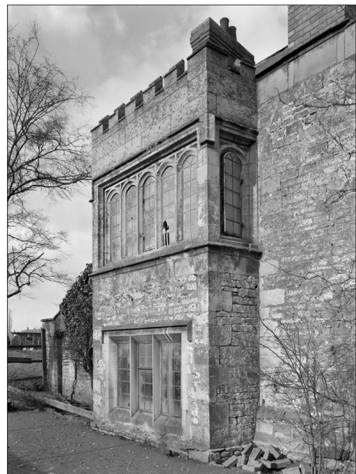
Figure 26. Bay window on south façade.
