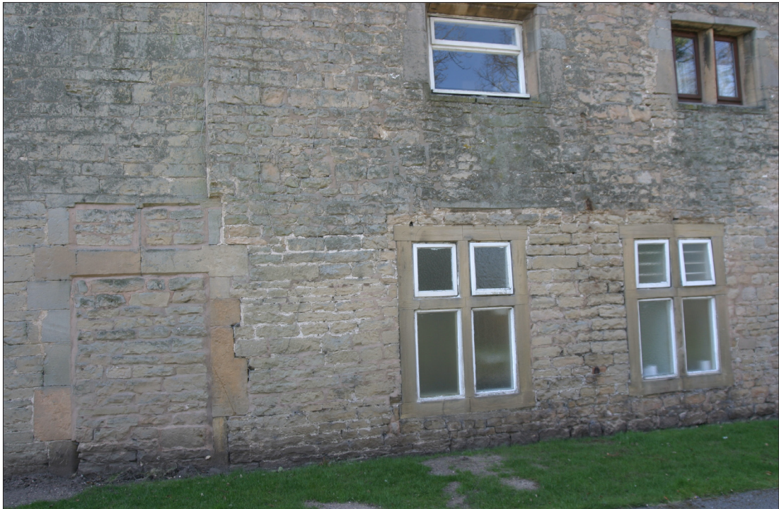
Figure 11. Detail of east façade of east range, southern end showing two surviving late 17th-century windows of 'hall' (now lighting WCs).
