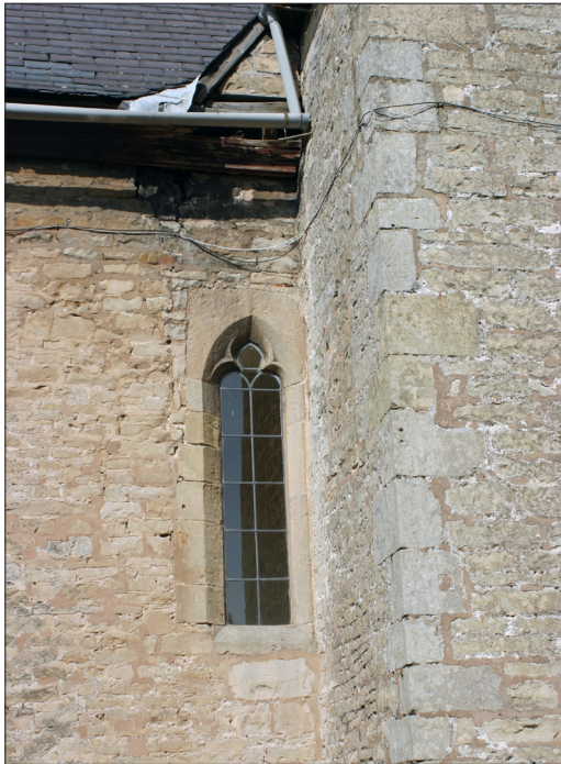
Figure 5. Gothic single-light window, now lighting landing of 19th-century staircase. Linda Monckton 04/06
