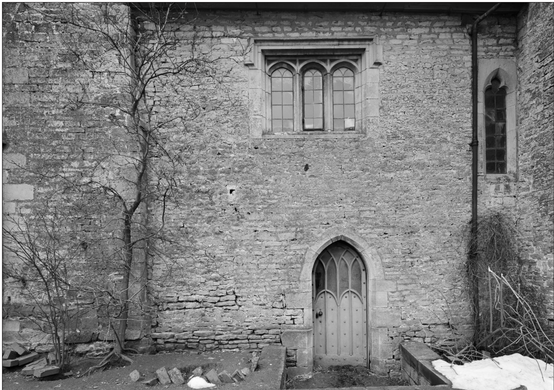
Figure 16. Main entrance to south range from c.1800, note alteration in ground level.
