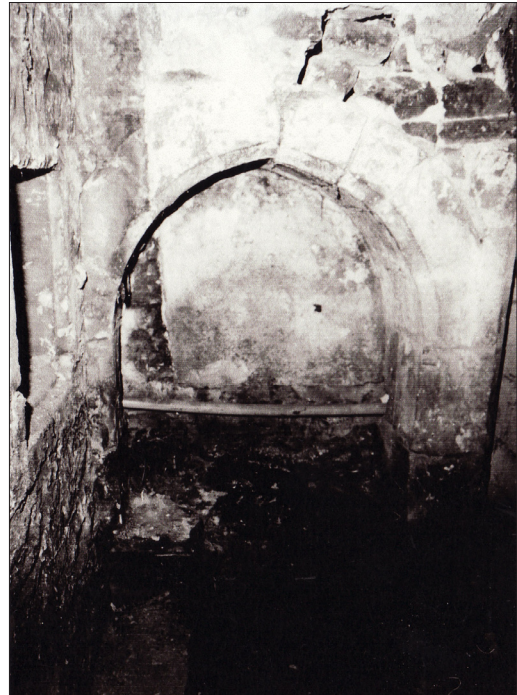
Figure 6. Blocked medieval opening situated in east wall, now confined within storage cupboard. Shows square headed opening to left. Courtesy of the Old Warsop Society
