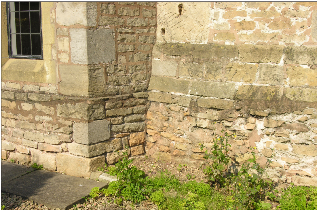
Figure 27. Detail of bay window, showing masonry abutting against 1706 chimney.
