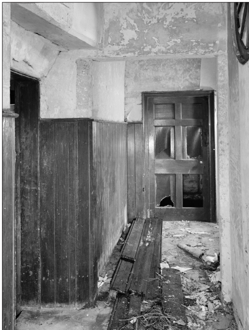
Figure 33. View along hall passage looking east, with 19th-century stairwell circular window to right. Opening to left, now location of inserted wooden staircase.
