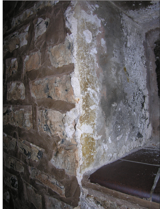
Figure 19. Detail of inserted breather in east wall of north range (barn) showing surviving 16th-century plaster on left jamb. Pete Smith 04/06
