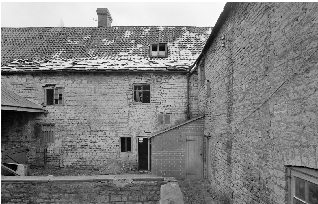
Figure 32. View into courtyard from south in 1966 Showing entrance arrangements at farm.
