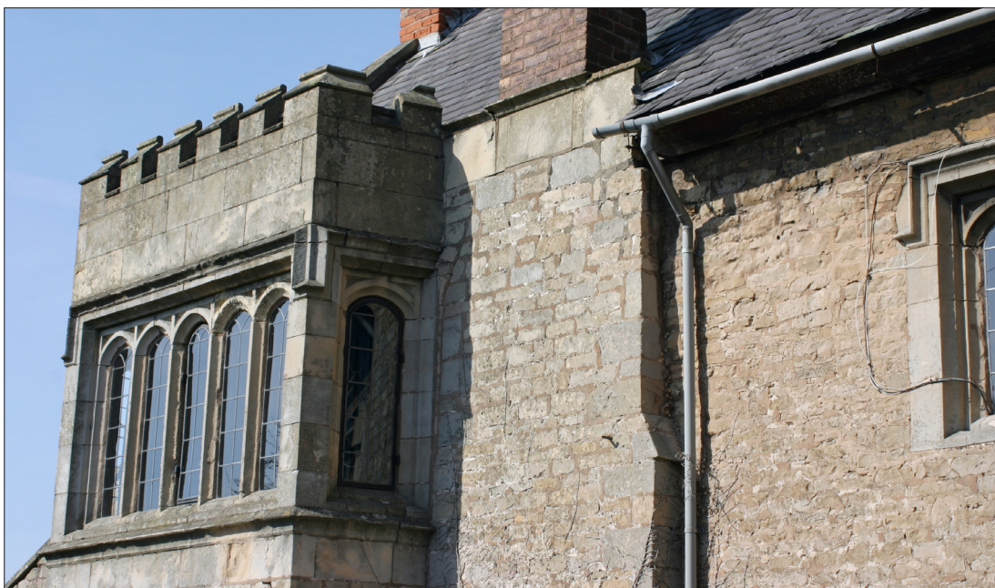
Figure 24. First floor of south façade of south range.
