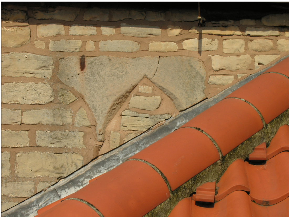
Figure 13. Detail of in situ blocked medieval window, in south side of barn.
