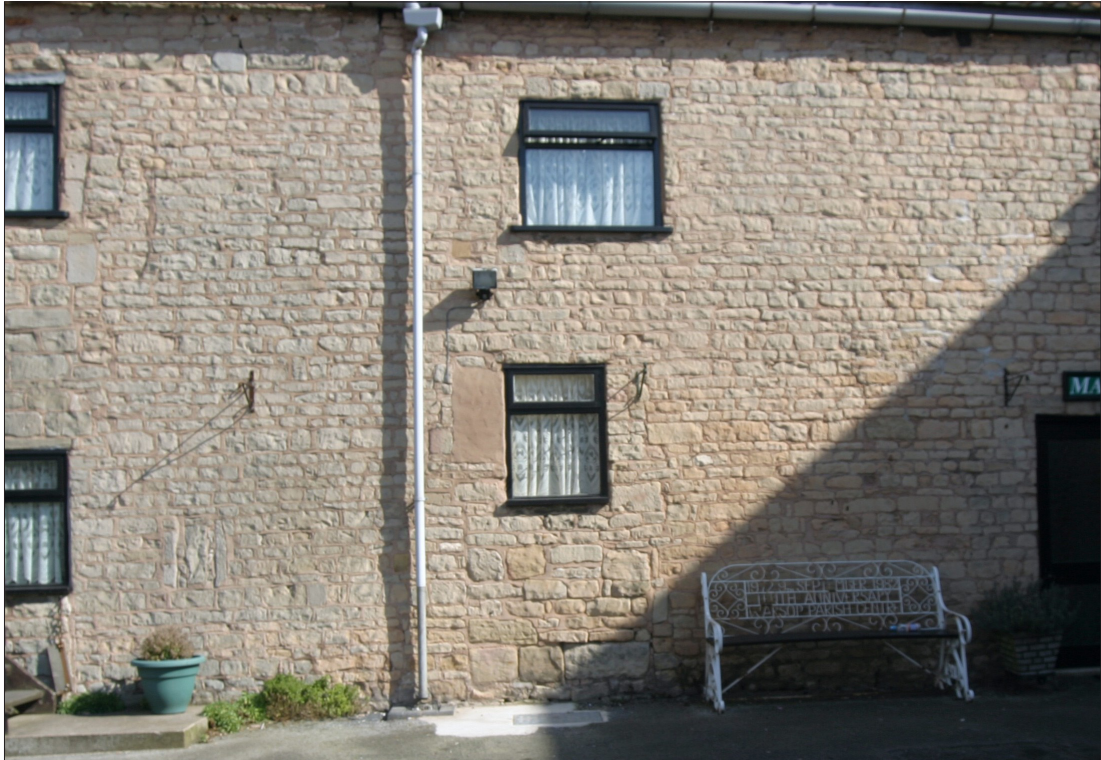
Figure 20. West façade of east range, central section, showing blocked entrance to centre of range.
