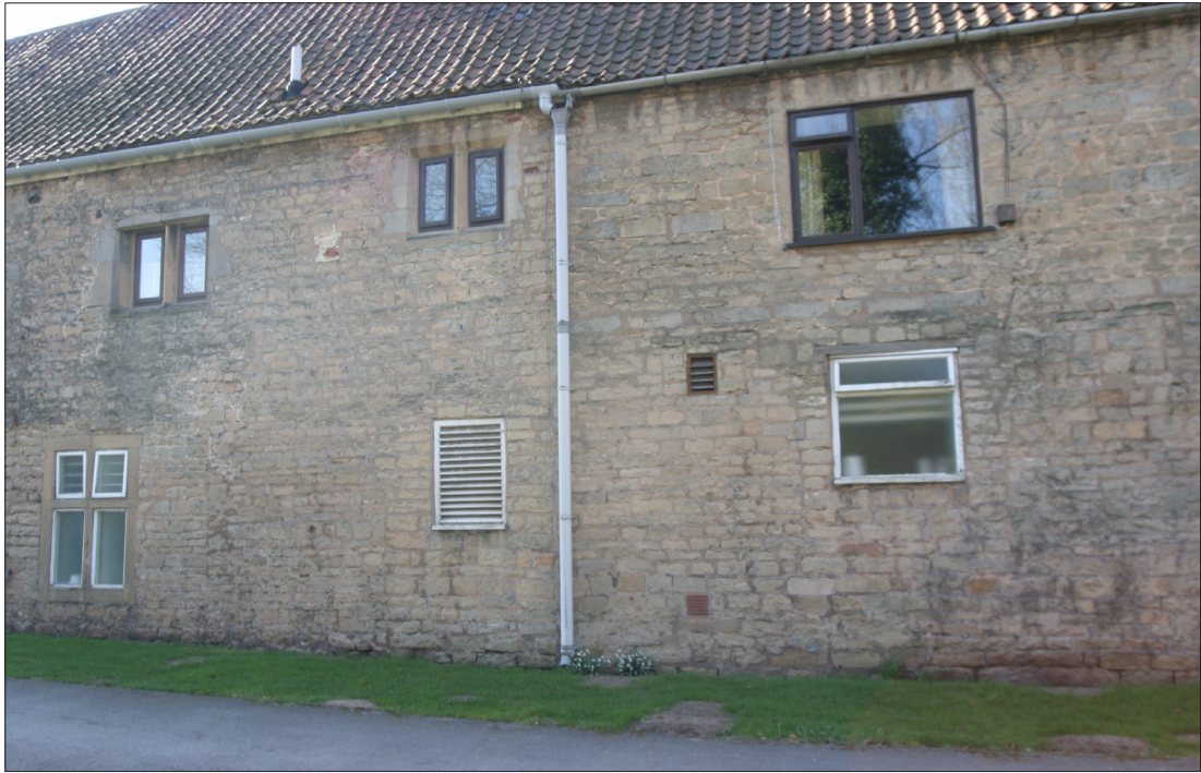
Figure 8. East façade of east range central section showing first floor early 17th-century windows above blocked doorway.
