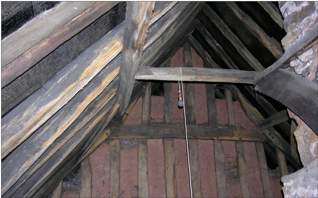
Figure 15. Roof over central area of east range.
