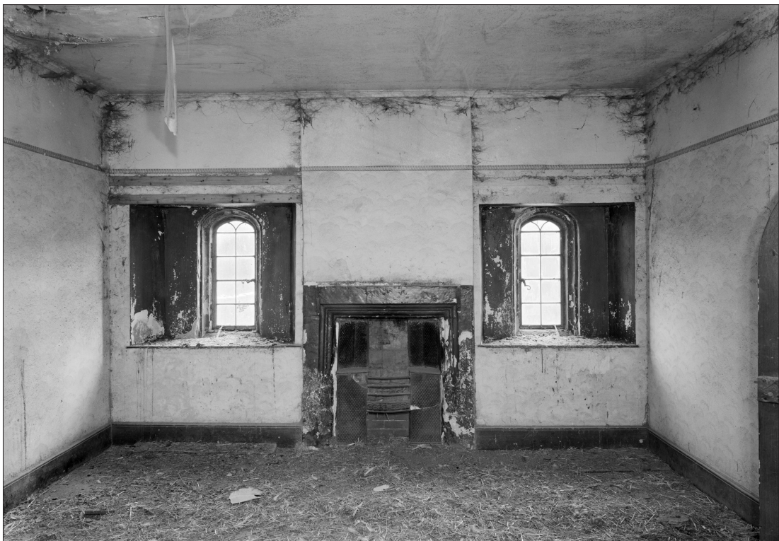
Figure 30. South wall of east range showing rearranged medieval features to provide symmetrical interior feature wall in c.1800.
