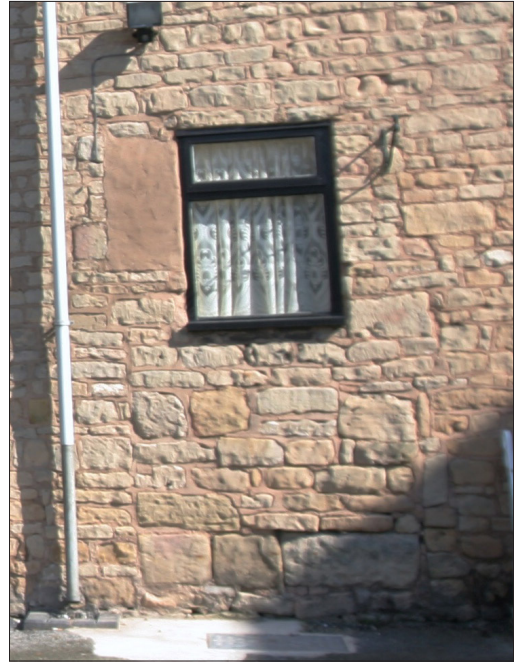
Figure 17. West facade of east range, showing blocked doorway to former great hall.
