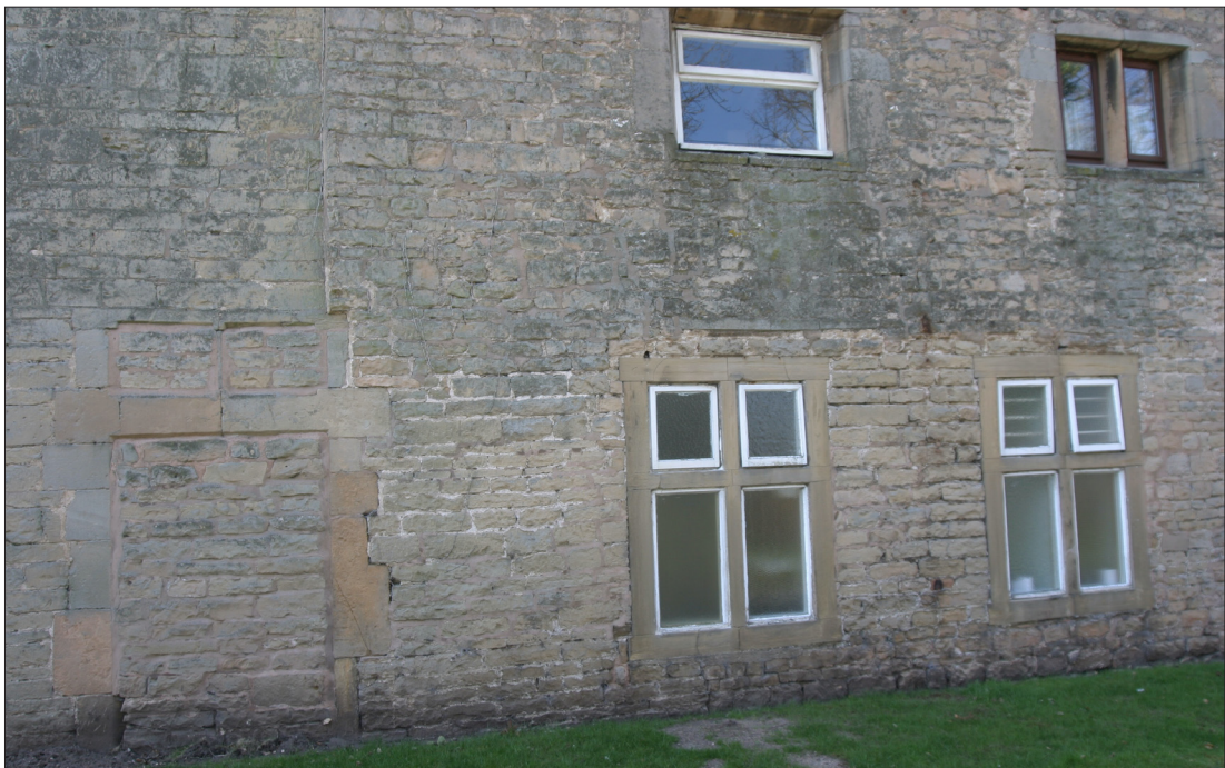
Figure 21. Detail of east façade of east range, southern end showing blocked early 17th-century doorway.
