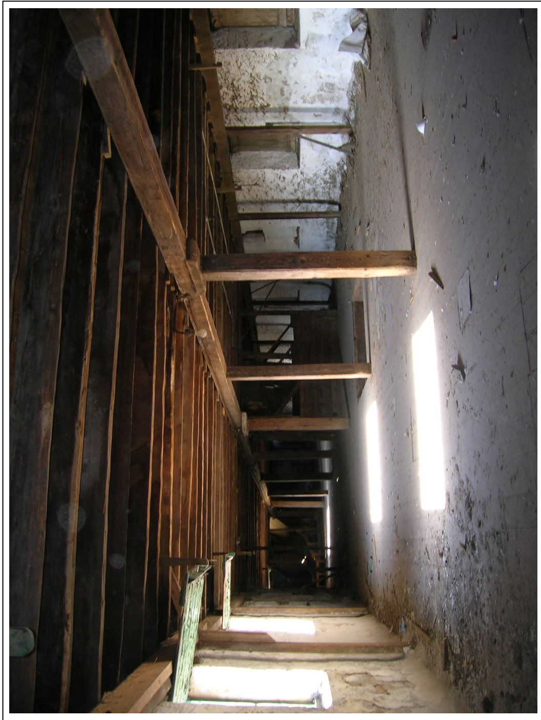
Figure 2: Second floor, looking north
