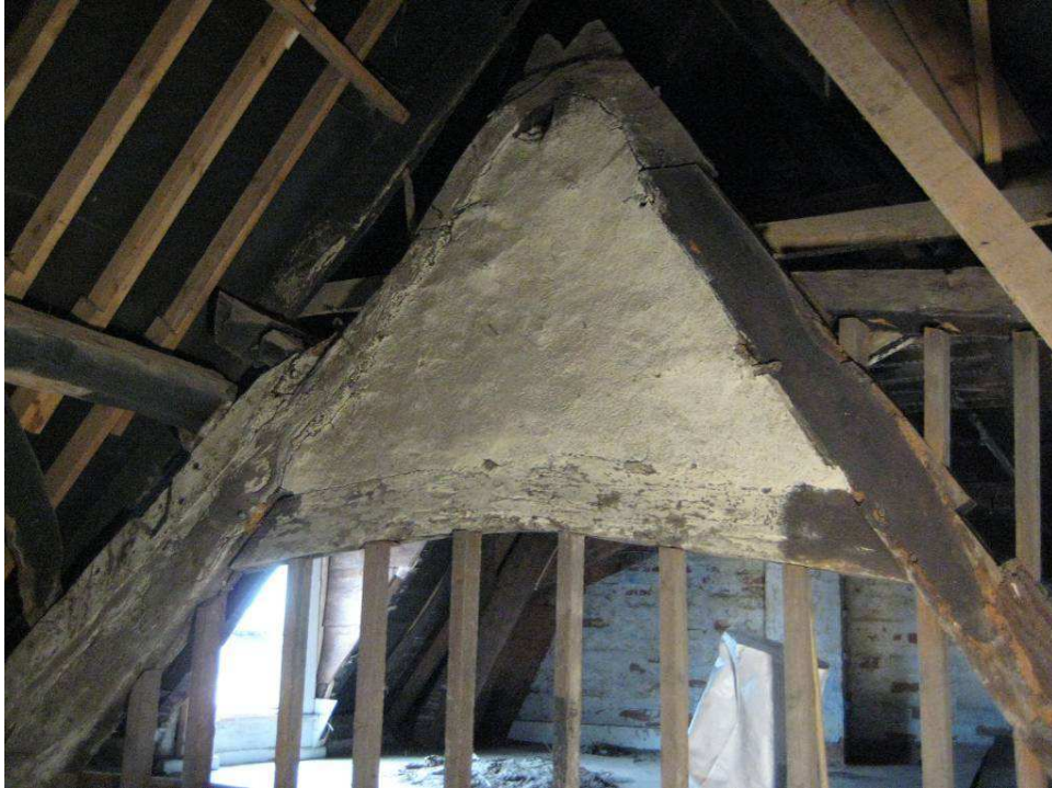
Figure 5: Truss B west face (photo Matt Hurford)
