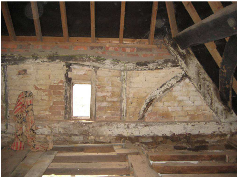
Figure 6: Truss C east face (photo Matt Hurford)
