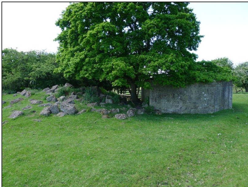
Figure 25 NRHE 1426123 Type 24 pillbox (No. 6 in Fig 22 and the table below) with adjacent rubble, possibly from a demolished pillbox. Photographed in May 2015.
