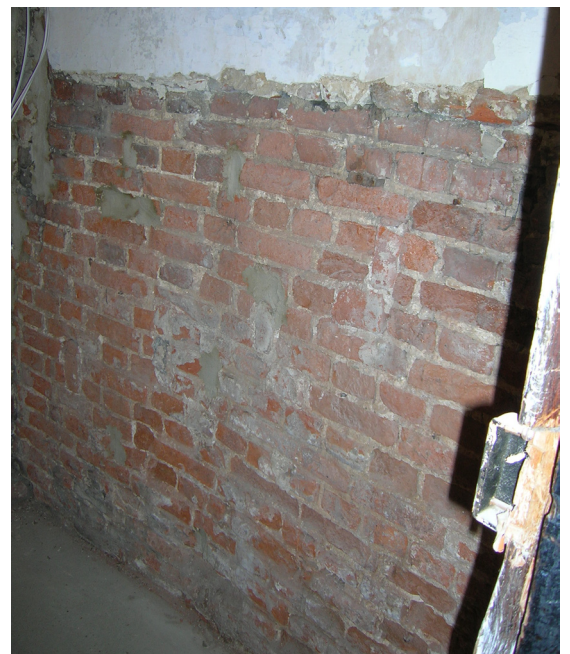
Fig. 57: East wall of room 12 (west wall of principal stack) exposed during works in 2007-08. Note inserted, and subsequently blocked, sockets for stair risers. (DP0070339).
