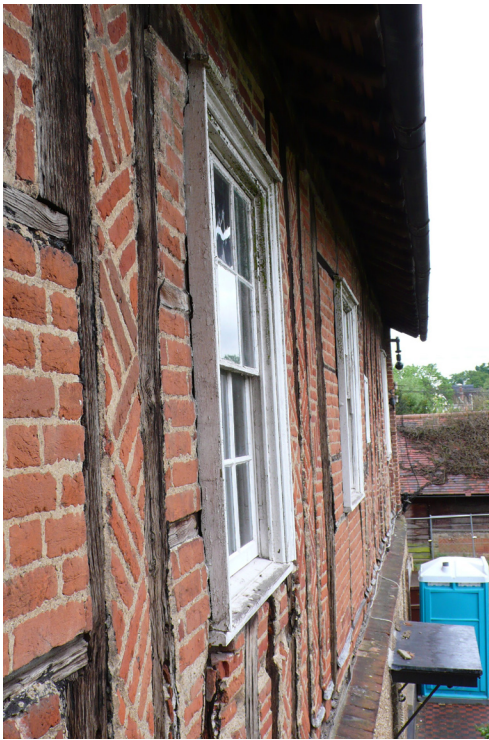
Fig. 49: Detail of south elevation, showing projecting 18 th century architraves (DP070335).
