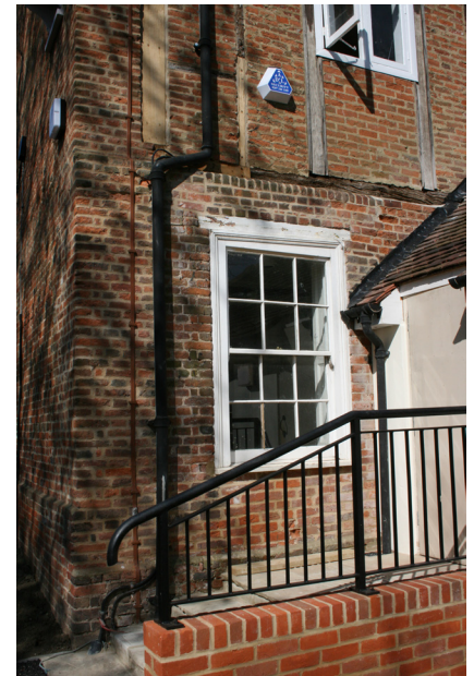
Fig. 11: Detail of east elevation, showing inserted sash window (DP040080).
