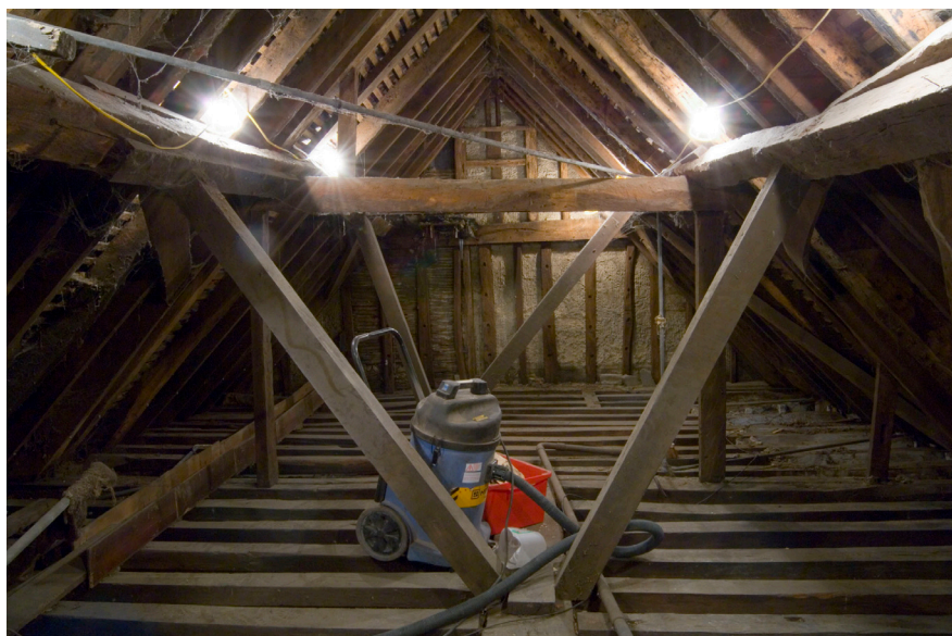
Fig. 35: Roof space of hall range, looking north. The struts in the foreground are later insertions. Photograph by Derek Kendall (DP042418).
