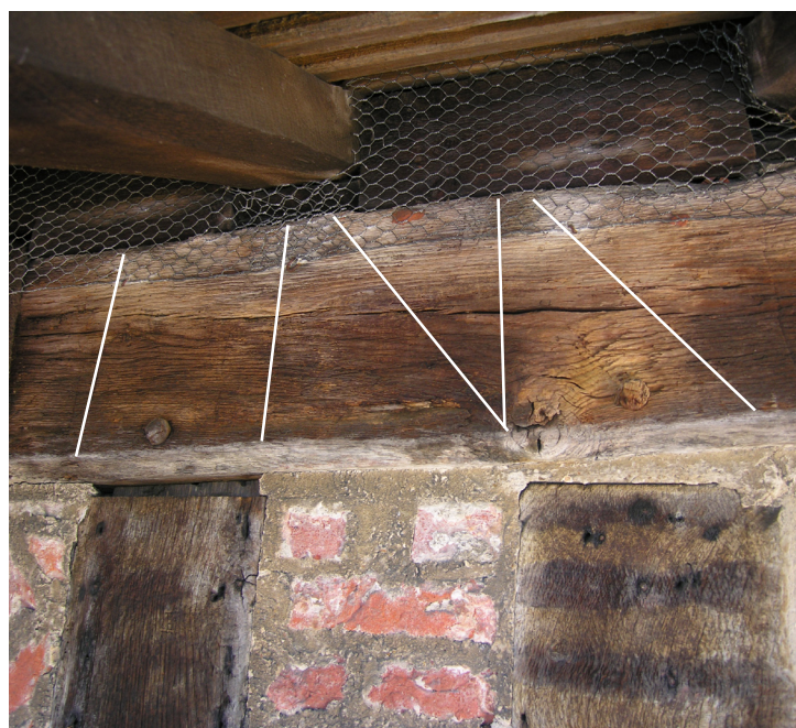
Fig. 10: Scribing marks on the wallplate of the west elevation (highlighted in white), inscribed during the 'setting-out' of the timber frame to indicate the position of the adjoining studs (DP040078).
