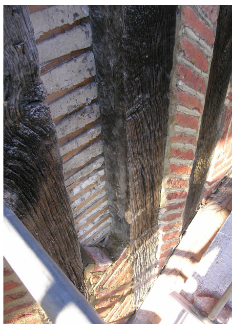
Fig. 9 The partial removal of nogging during conservation works in 2007 showed that the reveals of the studs were hollowed to provide a mortar key (DP040076).
