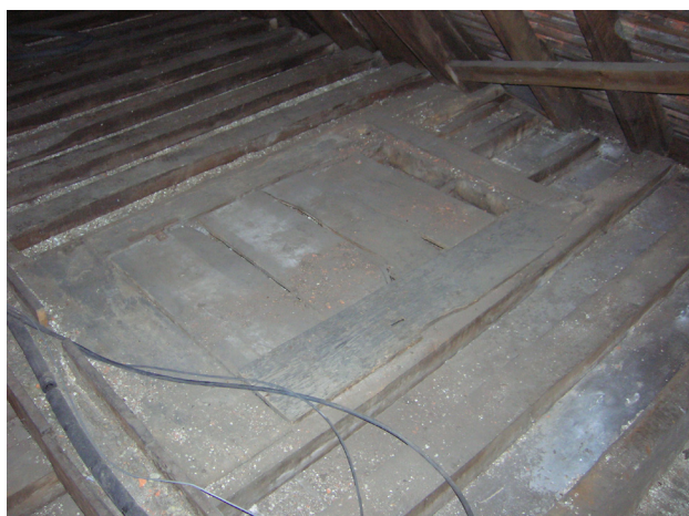
Fig. 34: Framed opening in attic floor (DP040094).
