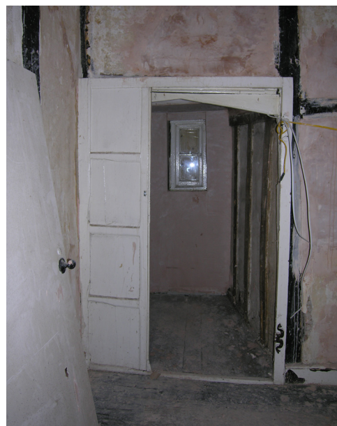
Fig. 33: Original, four-centred doorway to closet (room 26), reduced in size with reused 17 th century door (temporarily removed) and panelling (DP040093).
