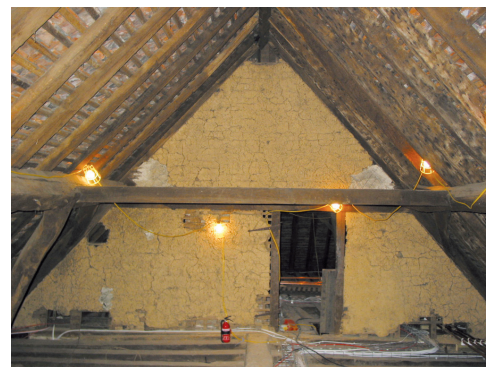
Fig. 39: Closed truss III of hall range (DP040096).
