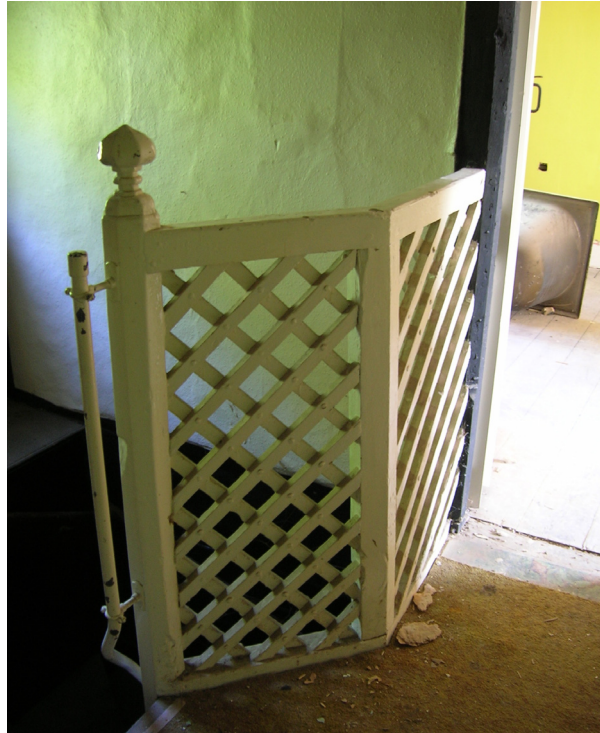
Fig. 19: Lattice balustrade, octagonal newel and finial of principal stair. (DP040086).
