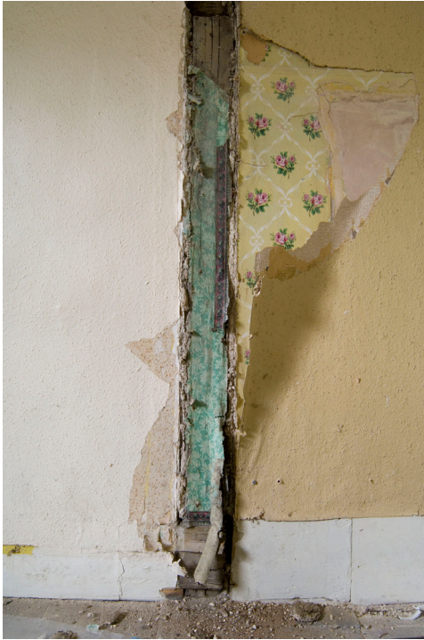
Fig. 64: Wallpaper fragments discovered in 2007 on the north wall of the hall chamber when partitions formerly dividing rooms 23, 31 and 32 were removed. Photograph by Derek Kendall (DP042394).
