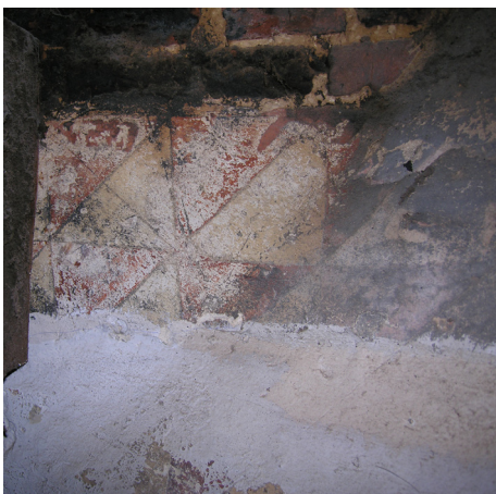
Fig. 17: Traces of a geometric decorative scheme of probable 17 th century date surviving on the plasterwork lining of the hall fireplace jamb. (DP040085).
