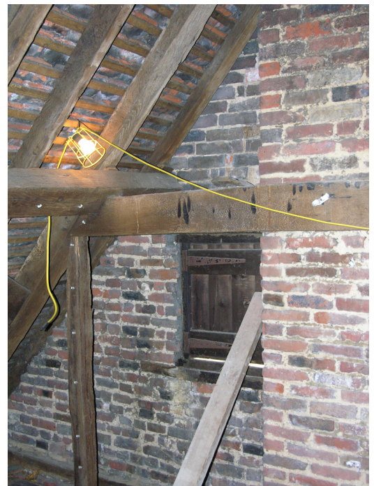
Fig. 45: Detail of south truss of hall range. Fair face outwards, indicating a terminal truss. The purlin extends beyond the principal rafter and there are no signs that the truss was ever closed. The stack is visible to the right (DP040099).
