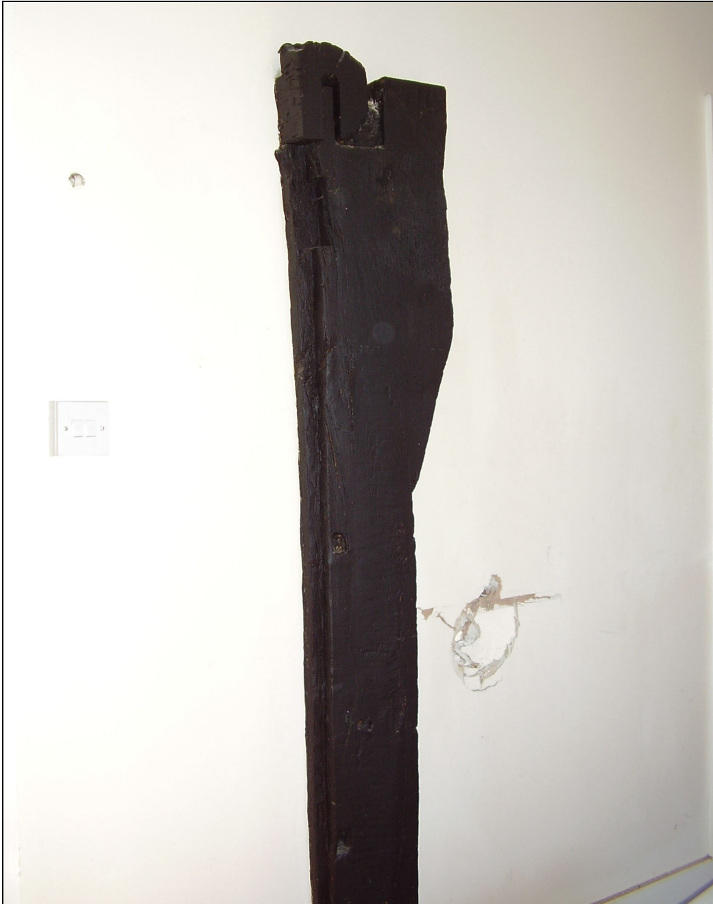
Figure 2: The east post exposed at first-floor level.
