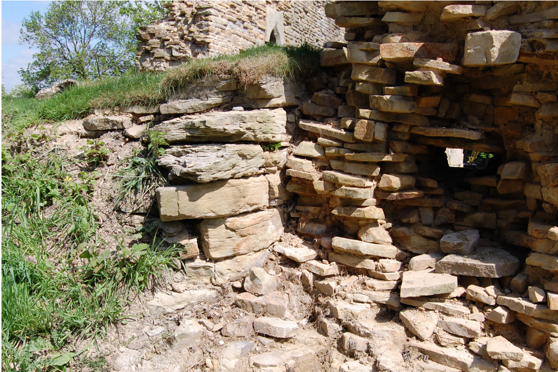
Figure 4: The junction between the south front of the Upper Court (left, with thicker courses) and the west wall of the Lower Court (right).
