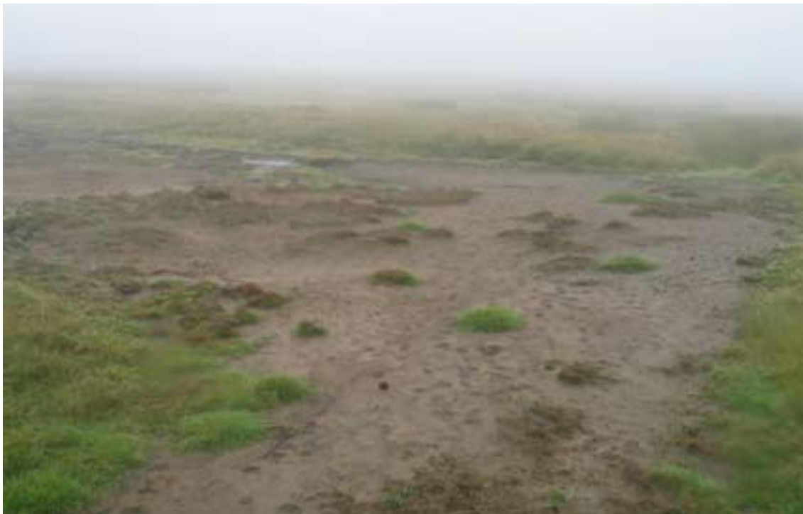
Figure 48: Sheet erosion where soils have been lost (272). Photograph taken in low cloud/ driving rain.
