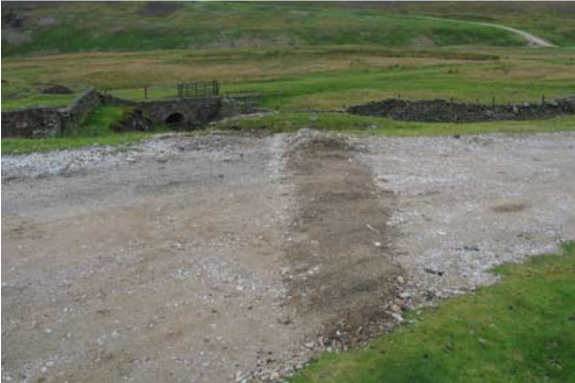
Figure 10: Example of Category 1a: deflection drain along Road 1 (85).
