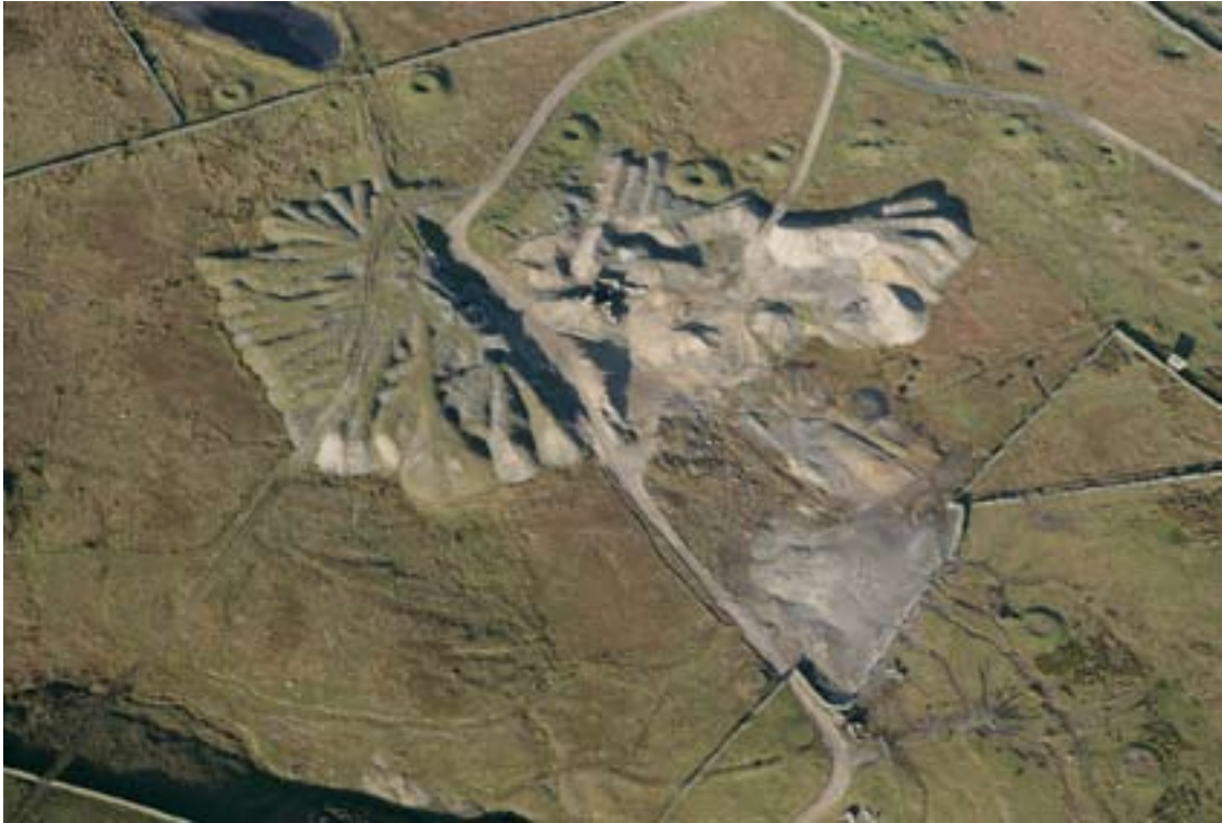
Figure 57: Zone H. Oblique aerial photograph from the south-east in 2008. Road 4 runs from top-centre to bottom-centre. NMR 20844/030/25-NOV-2008. © English Heritage. NMR.
