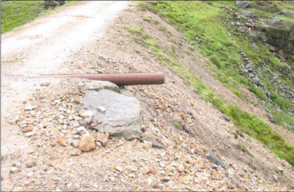
Figure 12: Example of Category 1c: metal-pipe drain along Road 1 (70).
