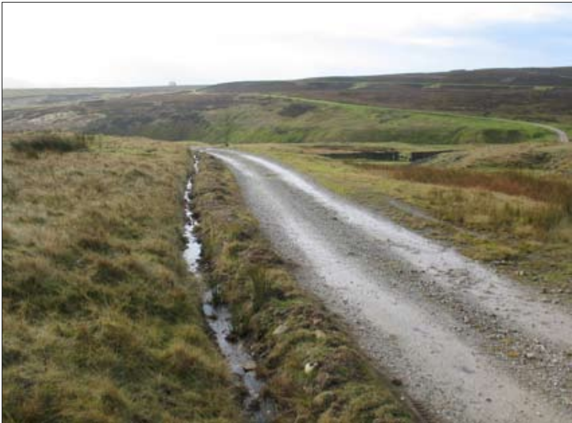
Figure 11: Example of Category 1b: roadside drain along Road 1 (108).
