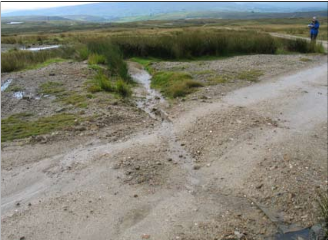
Figure 13: Example of Category 1d: wooden-trough drain along Road 1 (327).
