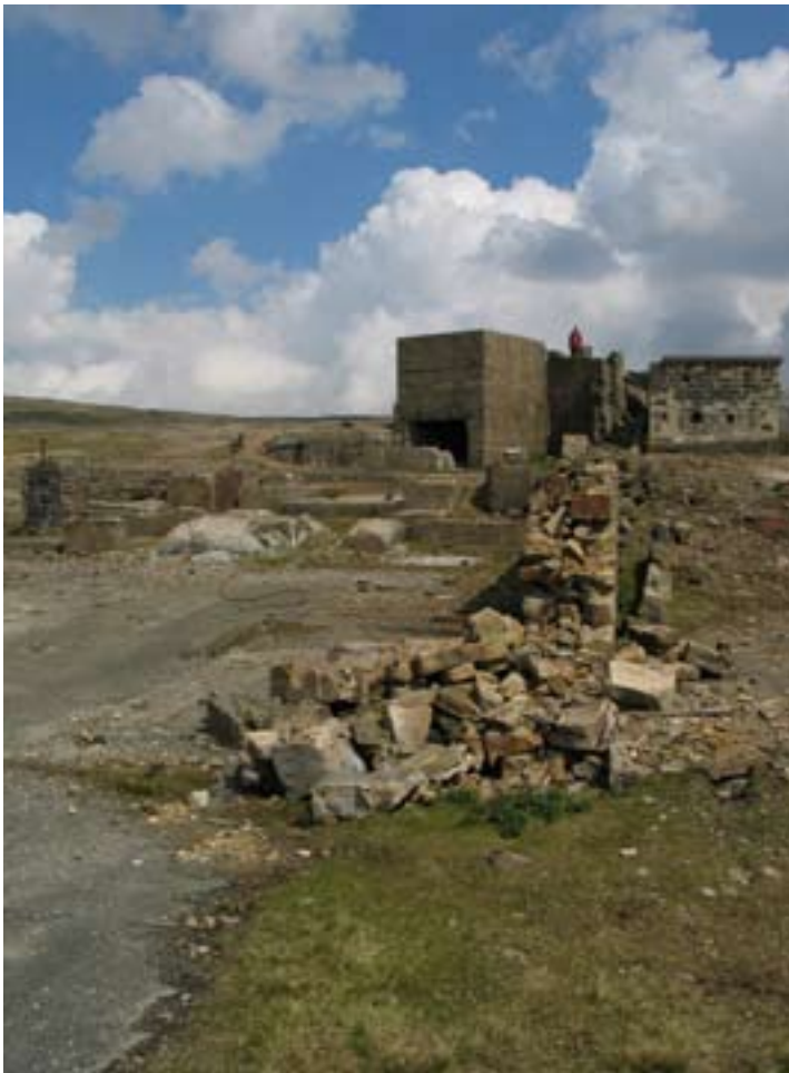
Figure 33: Example of Category 3f: visitor impacts. Visitors were observed climbing on the ruins of the Dales Chemical Company plant and the High Grinding Mill (in the background) and may have contributed to the collapse of fabric in this area (126).
