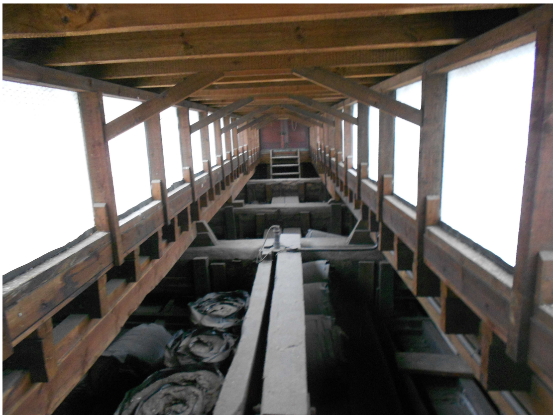
Figure 3: View looking south showing three of the four large pine beams over the Hall (Martin Bridge)
