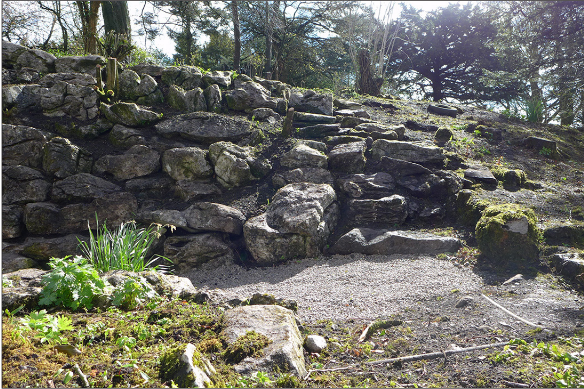
Figure 16: The blocked steps at the south end of the rock face, with a clear stretch of pipe relating to the buried irrigation system visible following a right-angled course across the surface in the foreground, looking east. © Historic England/Rebecca Pullen, 29th April 2015.
