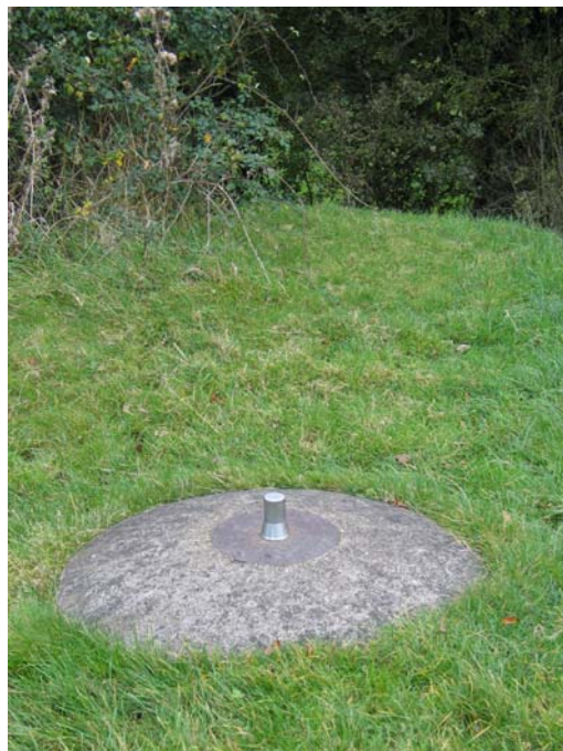
Figure 20 The mounting for the spigot mortar
