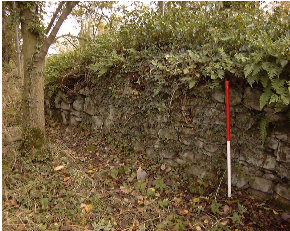
Figure 13. The possible standing section of precinct wall viewed from the north
