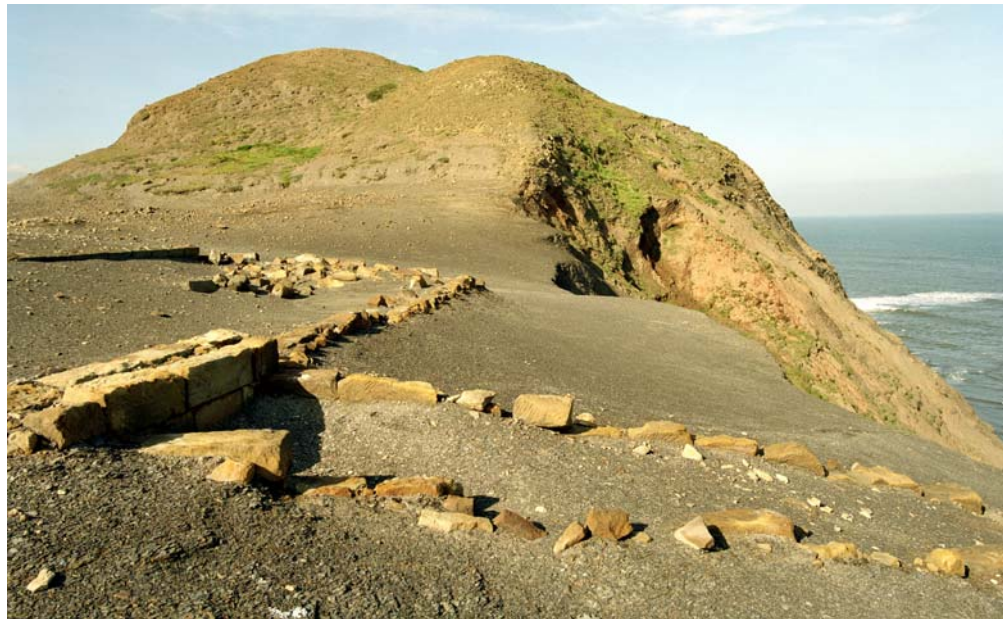
Figure 39. Detail of the north-east side of building 1, showing the junction of the main range and northern annex. (NMR AA040241)
