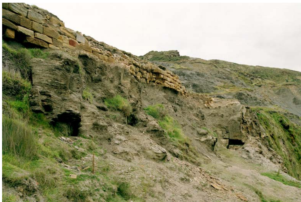
Figure 48. The collapsed ledge at the edge of the alum-house shelf. Note the entrance to mine 5 at right of frame, and wall 3 (part of the alum house) along the top of the rear edge of the ledge. (NMR AA040229)
