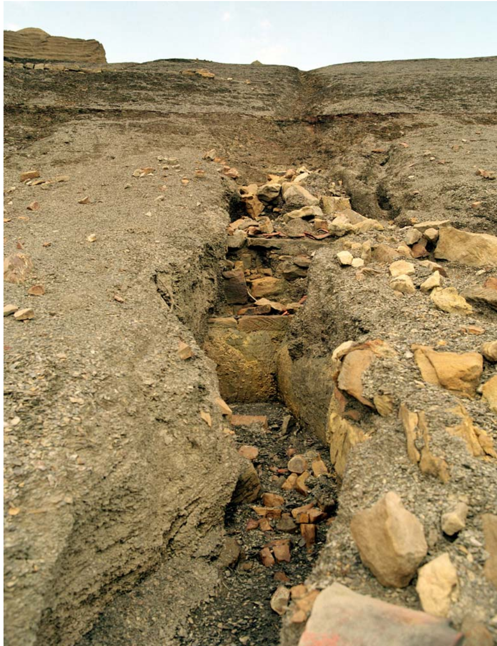
Figure 34. Detail of the silted clarifying tanks north of alum house 2. (NMR AA040252)
