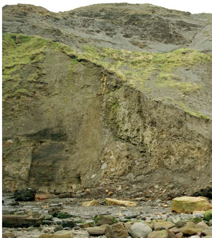
Figure 47. The possible side wall of cistern 3 in the cliff face at the edge of the 1829 landslip. (NMR AA040244)
