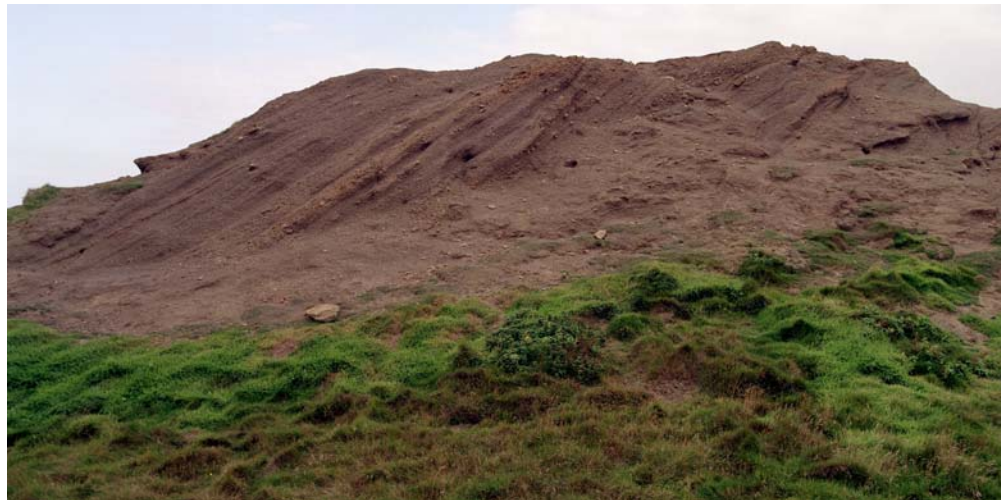
Figure 18. Tip lines in spoil dump area 4 exposed in the east side of the cut for track 9. (NMR AA040266)
