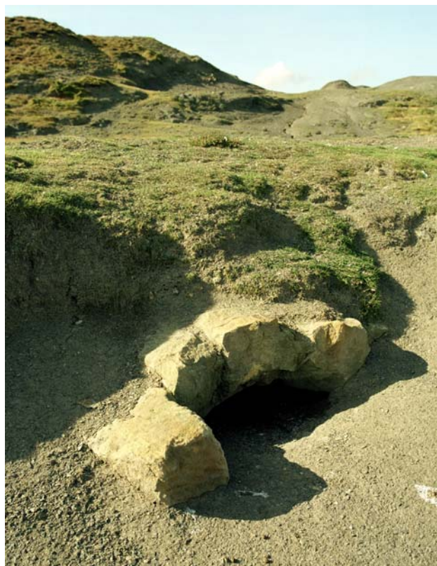
Figure 30. Detail of the vaulted roof at the probable eastern portal of the liquor-trough tunnel. (NMR AA040222)
