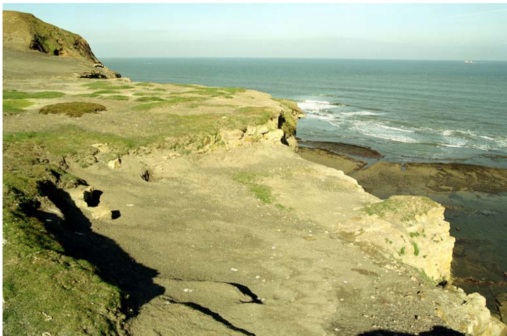
Figure 41. The surviving south- western end of building 3. The roof of the liquor-trough tunnel is just visible left of frame. (NMR AA040223)
