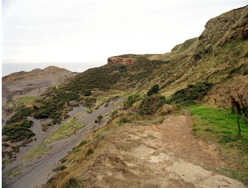
Figure 42. View north-east along track 1 from the edge of the 1999 cliff collapse. In the foreground a diagonal line of capstones presumably marks the course of the gutter taking water to the steeping pits, whilst in the middle distance the slumped sandstone marks the heel of the 1829 landslip. (NMR AA040237)
