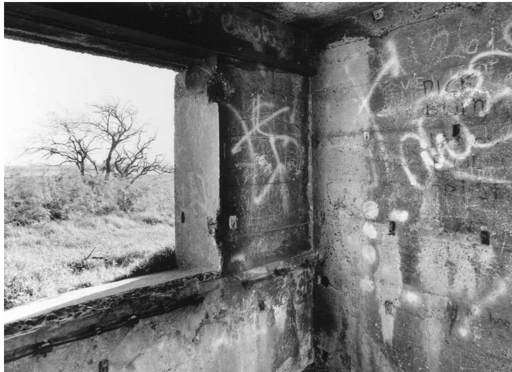
Figure 16 Detail of the aperture inside DEL 2, showing the remains of metal guide rails for sliding shutters (©Crown copyright. NMR: AA/031300)
