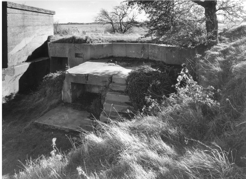
Figure 10 Emplacement for gun no III, showing the gun floor, ready-use lockers and barquette (©Crown copyright. NMR: AA/031303)
