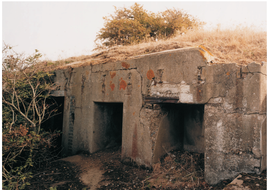
Figure 14 Ready use lockers in the flank wall north of emplacement no II, with the scars of sawn-off RSJs for the elevated walkway above (©Crown copyright. NMR: AA/046703)
