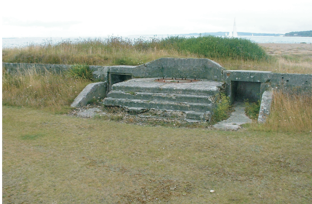
Figure 17 One of the emplacements of the 1893 6-pounder QF battery at Hurst Castle. Note the similar gun floor and barbette but the simpler layout and the scarcity of ammunition lockers
