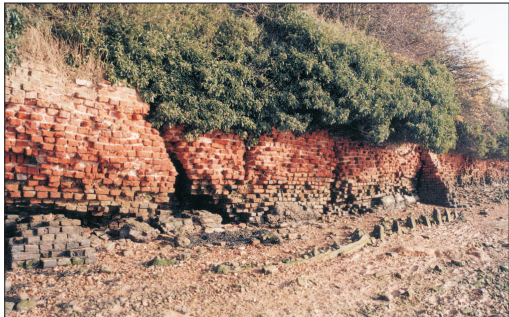
Figure 25 The revetment wall of the lower gun line with the timber remains of the tidal defences in front (NMR: AA031343)
