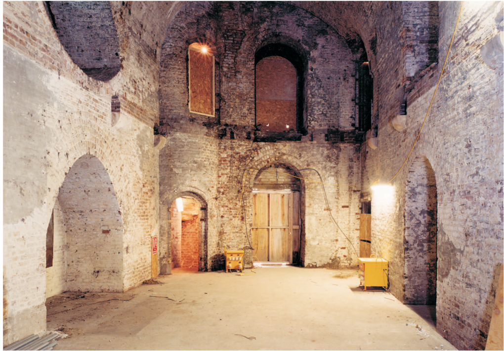
Figure 17 Clarence Tower, west casemate ground and first floor levels looking north. The timber floor structure has gone, leaving only the stone corbels from the tie beams. Note the different design of the artillery embrasures on the ground and first floors (at left) (© NMR:AA020022)
