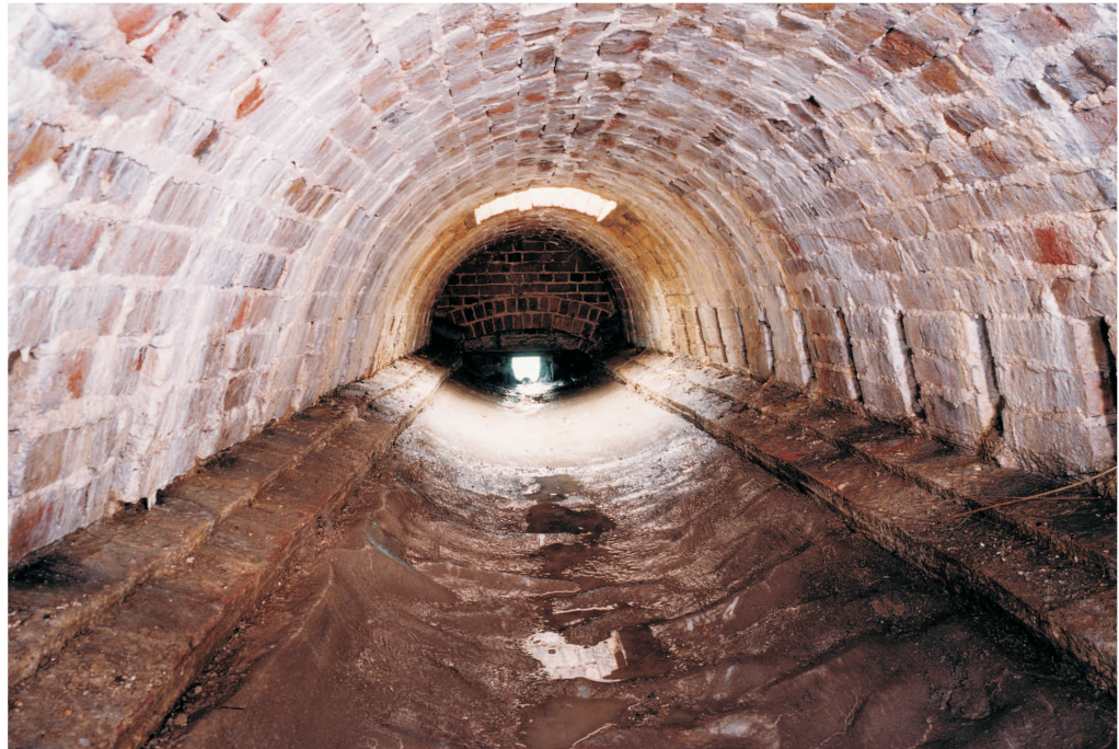
Figure 31 Clarence Tower; interior of the large central cistern, situated between the roof level and the first floor vaults, looking north to the drainage aperture (© NMR: AA021147)
