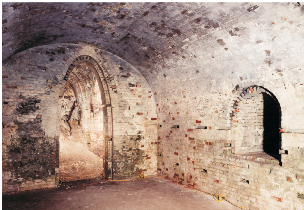
Figure 37 Clarence Tower; the main magazine, looking north-west. Note the parabolic entrance and the lighting recess (at right) (© NMR: AA020011)
