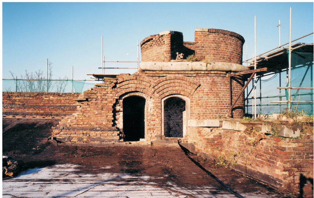
Figure 34 Clarence Tower; the NW turret. The right-hand entrance is to the newel stair, the left-hand to the store room (© NMR: AA021108)
