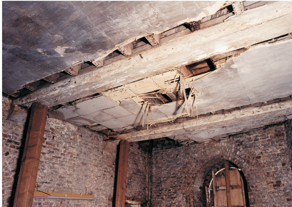
Figure 21 Clarence Tower, detail showing the structure of the ceiling in the ground floor east casemate. The wooden props at left are modern (© NMR: AA020015)
