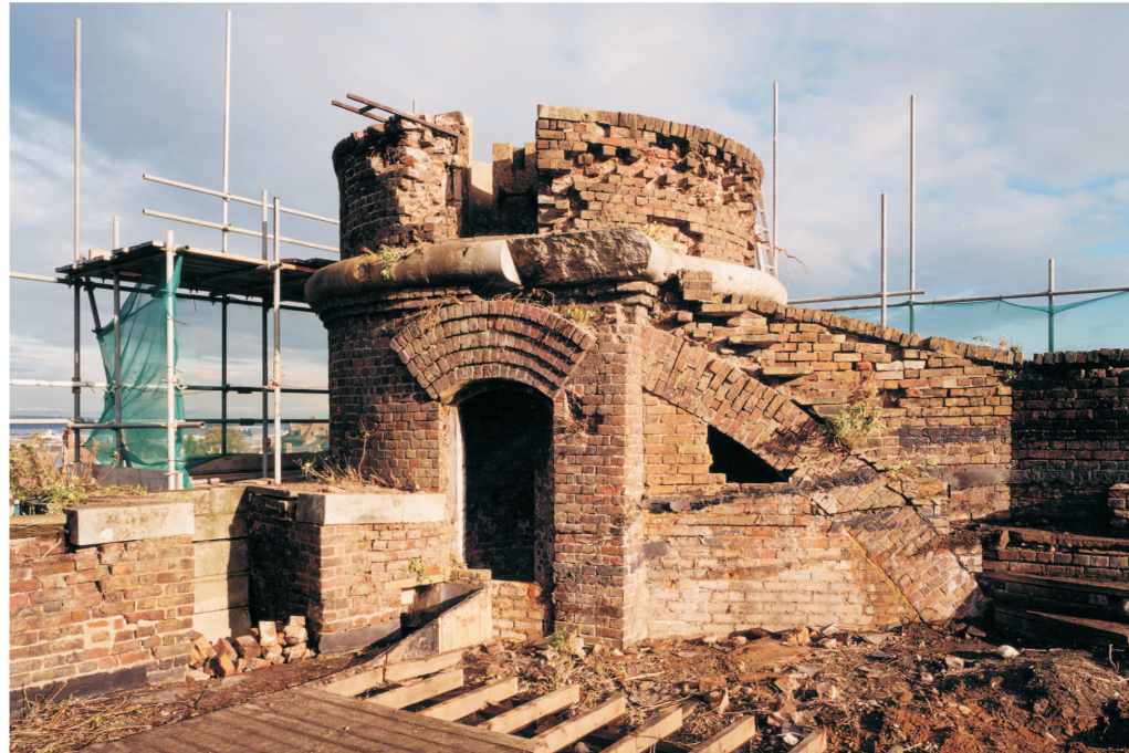
Figure 36 Clarence Tower; the NE turret. Note the steps over the flying buttress, ascending to the observation platform (© NMR: AA020048)
