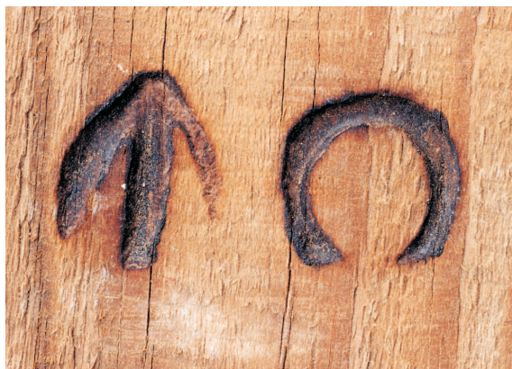
Figure 24 The Board of Ordnance symbol, as branded onto one of the first floor timbers in Clarence Tower. The symbols are each 3.5cms tall (© NMR: AA031469)
