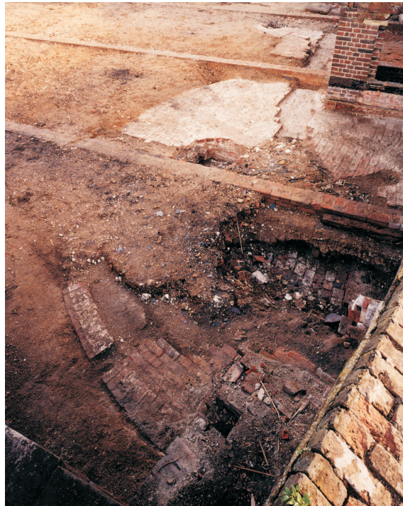
Figure 27 Clarence Tower; the south-western corner of the roof level, showing the emerging semi-circle of gun position no I, badly damaged by a broad trench cut for the insertion of a 20th-century dwarf wall for a later roof (© NMR: AA021135)
