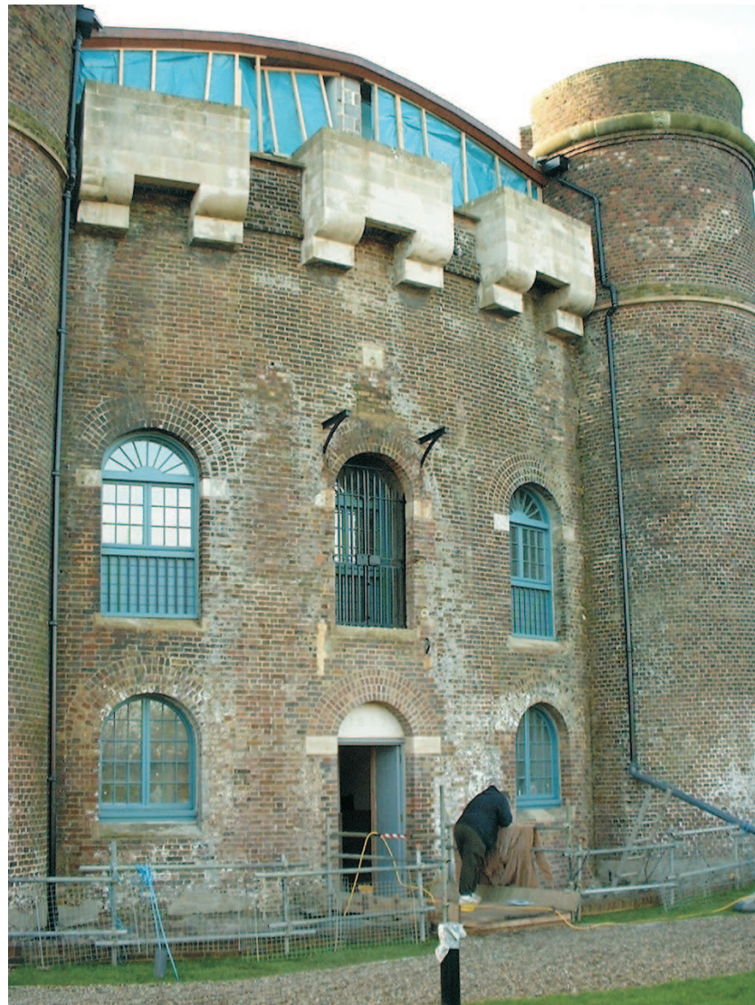
Figure 9 The north elevation of Clarence Tower, with refurbishment nearing completion, in December 2002. Note the Portland machicolations, original entrance at first floor centre and new entrance at ground floor centre. The structure above the machicolations is modern (author)
