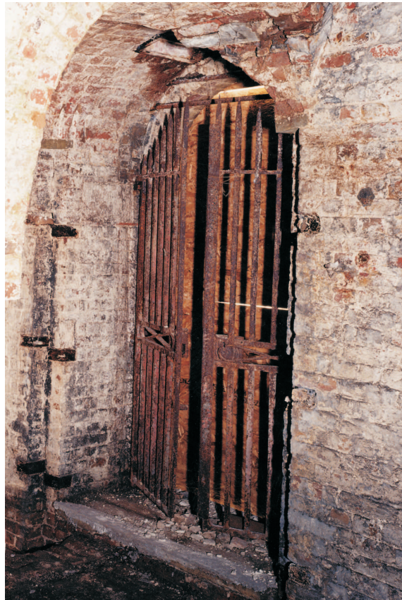
Figure 22 Secondary phase iron gates in the north elevation of Clarence Tower, guarding the first floor entrance (© NMR: AA020019)
