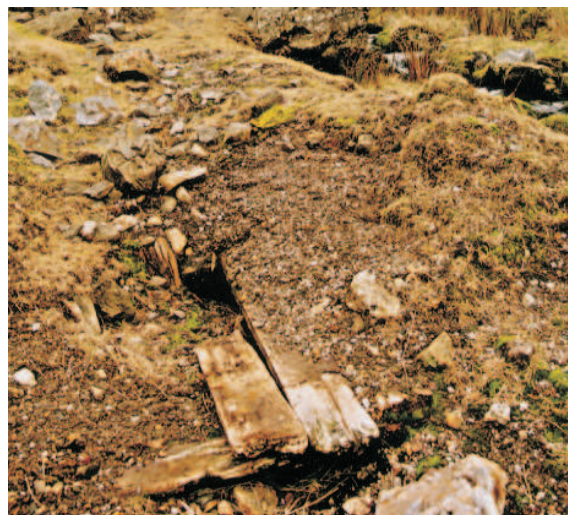
Figure 13. Exposed roof timbers in mine level ML6 in Todd Gill, viewed from the west (NMR/AA021950)
