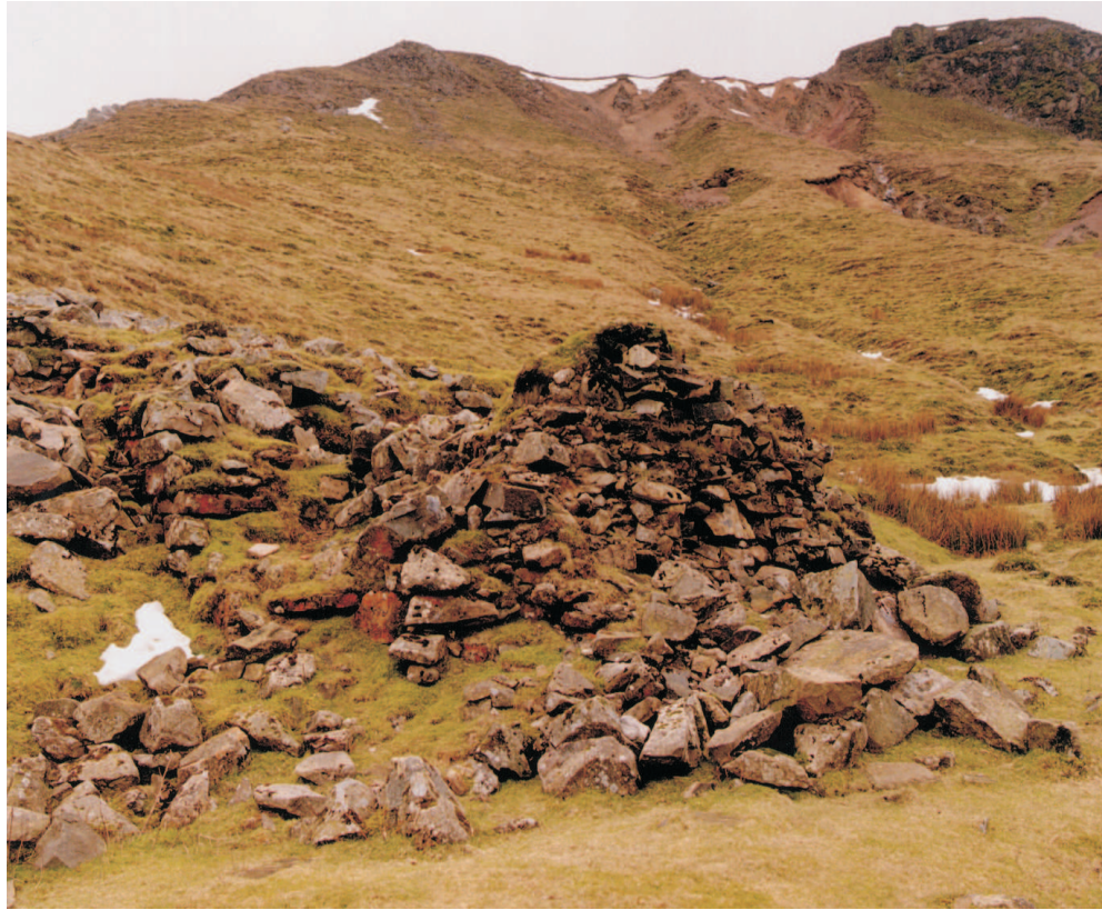
Figure 33. Ruins of the Cornish engine house at Lainton's Shaft, viewed from the north (NMR/AA021957)
