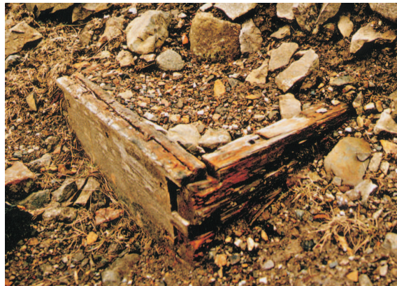
Figure 30. Wooden mortice-and-tenon frame exposed by erosion at mill complex MC5 (NMR/AA021946)
