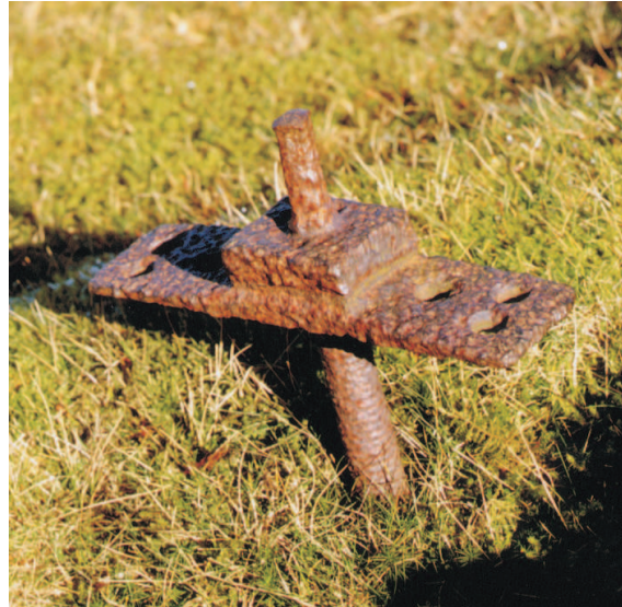
Figure 22. Spindle near top of dam to reservoir R2 (NMR/AA021994)
