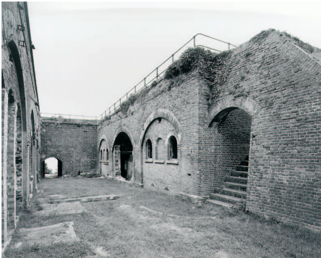
Figure 30 The Guard House range from the north-east (NMR: BB99/15911)
