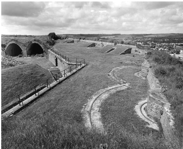
Figure 15 The terreplein along the eastern and north-eastern faces, showing the parapet, the gun emplacements and the racers for the traversing platforms (NMR: BB99/15925)
