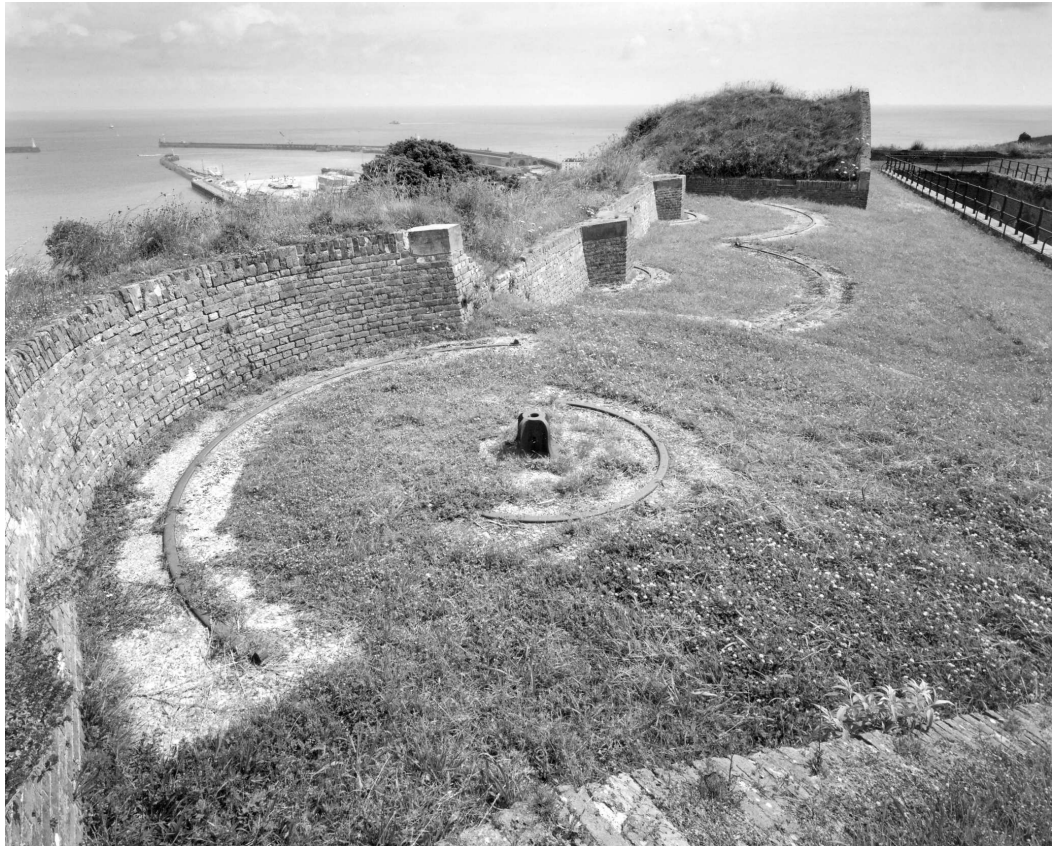
Figure 17 The east face of the terreplein, showing emplacement 3 with its 'C' pivot; emplacements 10 and 11 lie beyond (NMR: BB99/15924)
