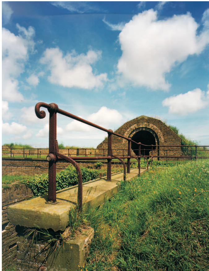
Figure 18 The side arms store, western elevation (NMR: BB99/15922)
