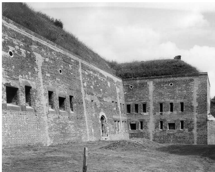
Figure 20 No 4 caponier with adjacent Sally Port and embrasures of gun rooms and musketry gallery (NMR: BB99/15890)
