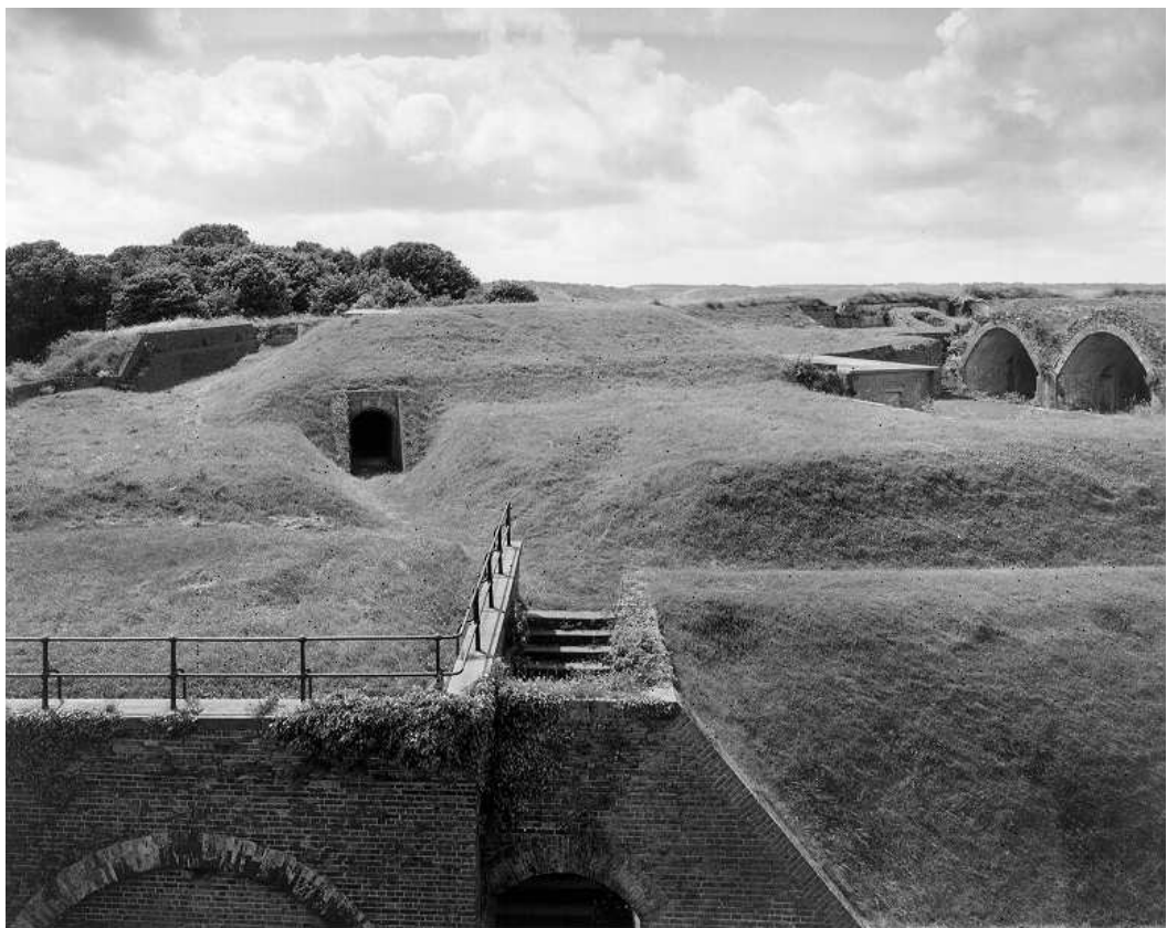
Figure 45 The Main Magazine mound and entrance, from the east (NMR: BB99/15934)
