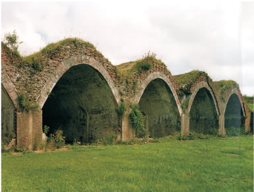
Figure 37 The Soldiers' Quarters: general view from the south (NMR: BB99/15930)
