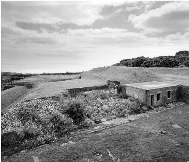
Figure 43 Remains of the Ablutions building and adjacent Staff Sergeants' Quarters, with the 20th-century shelter at extreme right (NMR: BB99/15932)
