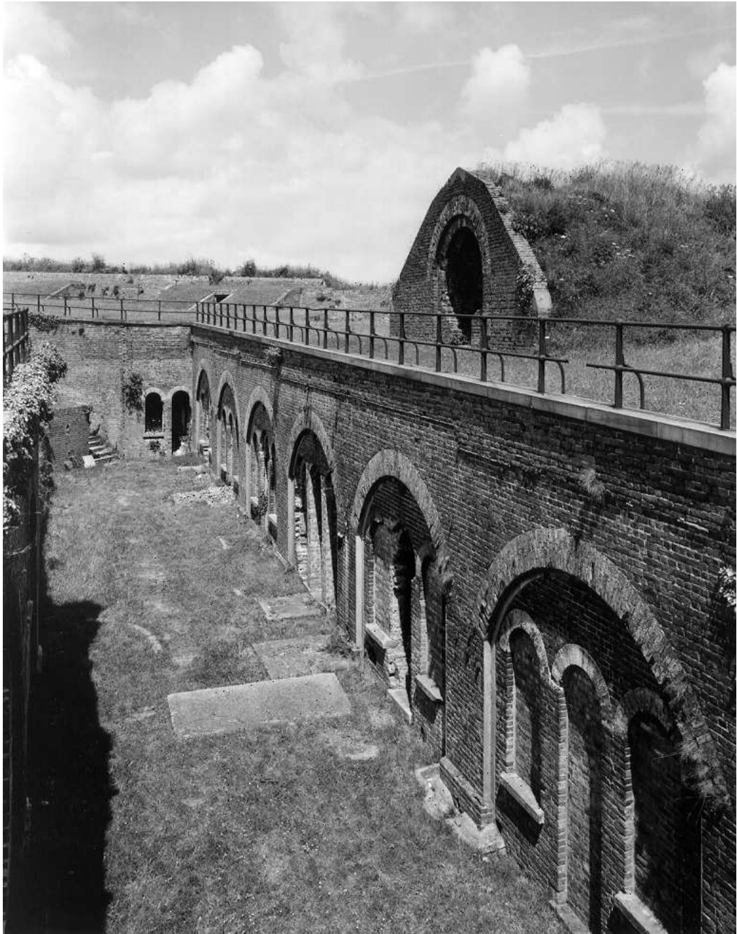
Figure 34 The Officers' Quarters: general view from the south, also showing the side arms store on the terreplein above (NMR: BB99/15918)
