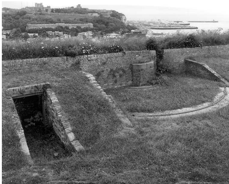
Figure 16 Emplacement no 5, on the north-east face of the terreplein, with its ready-use ammunition locker (NMR: BB99/15927)
